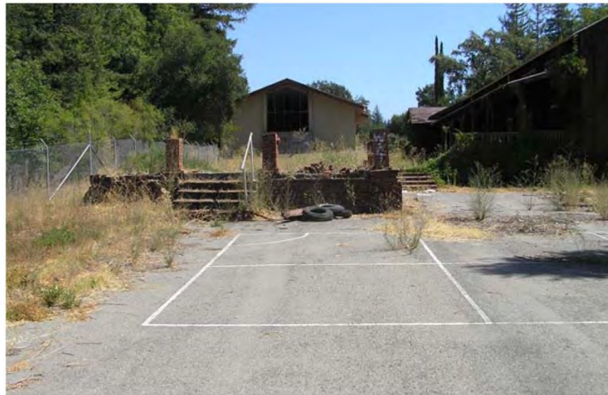
Alma College Dormitory porch ruin, exterior view looking east. The brick paving, stairs, and a few piers remain.
