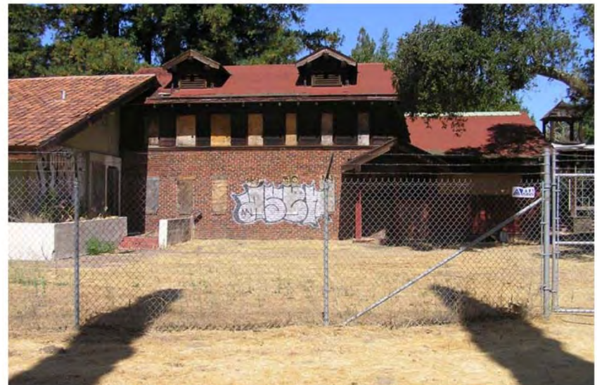
The brick and shingle 1934 library with larger 1950 library to the right.
