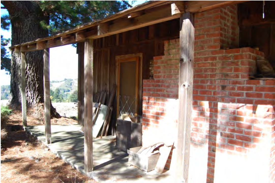
View from the southeast
