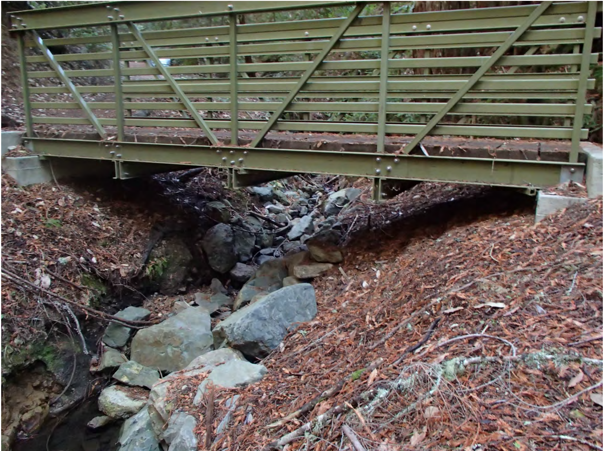
Exhibit C: Railings Alternatives Non-vehicle truss bridge on ECDM trail
