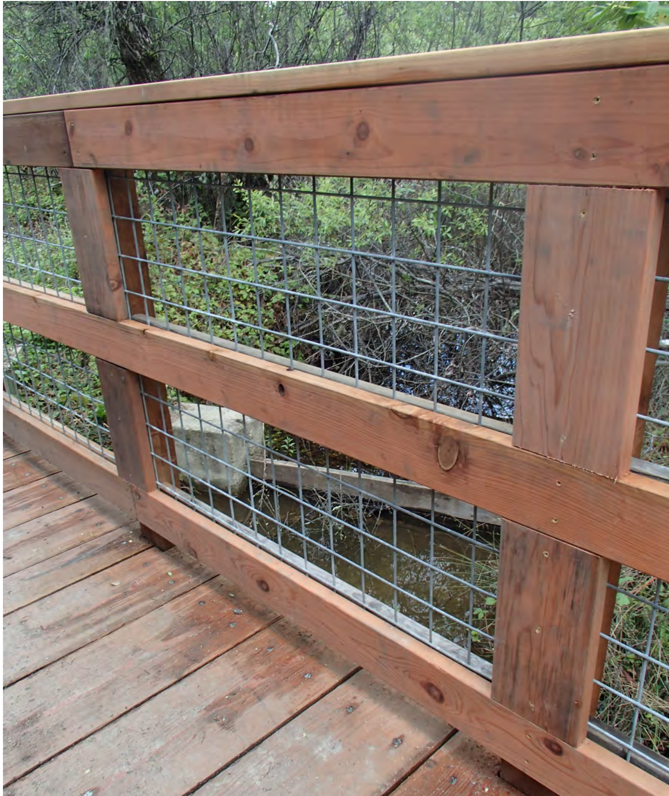
Exhibit C2: Welded Wire Mesh Detail
