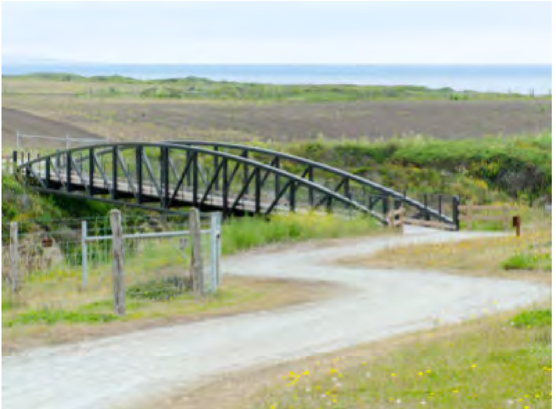
Exhibit B8: Prefabriacted Vehicle Truss Bridge at Cowell-Purisima Trail (POST)
