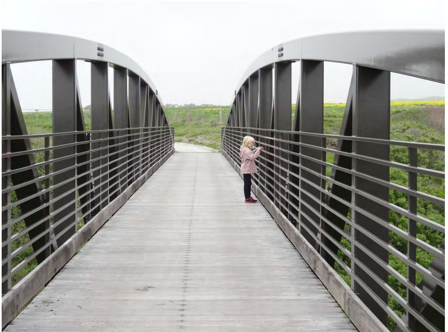
Exhibit B7: Prefabricated Vehicle Truss Bridge at Cowell-Purisima Trail (POST)
