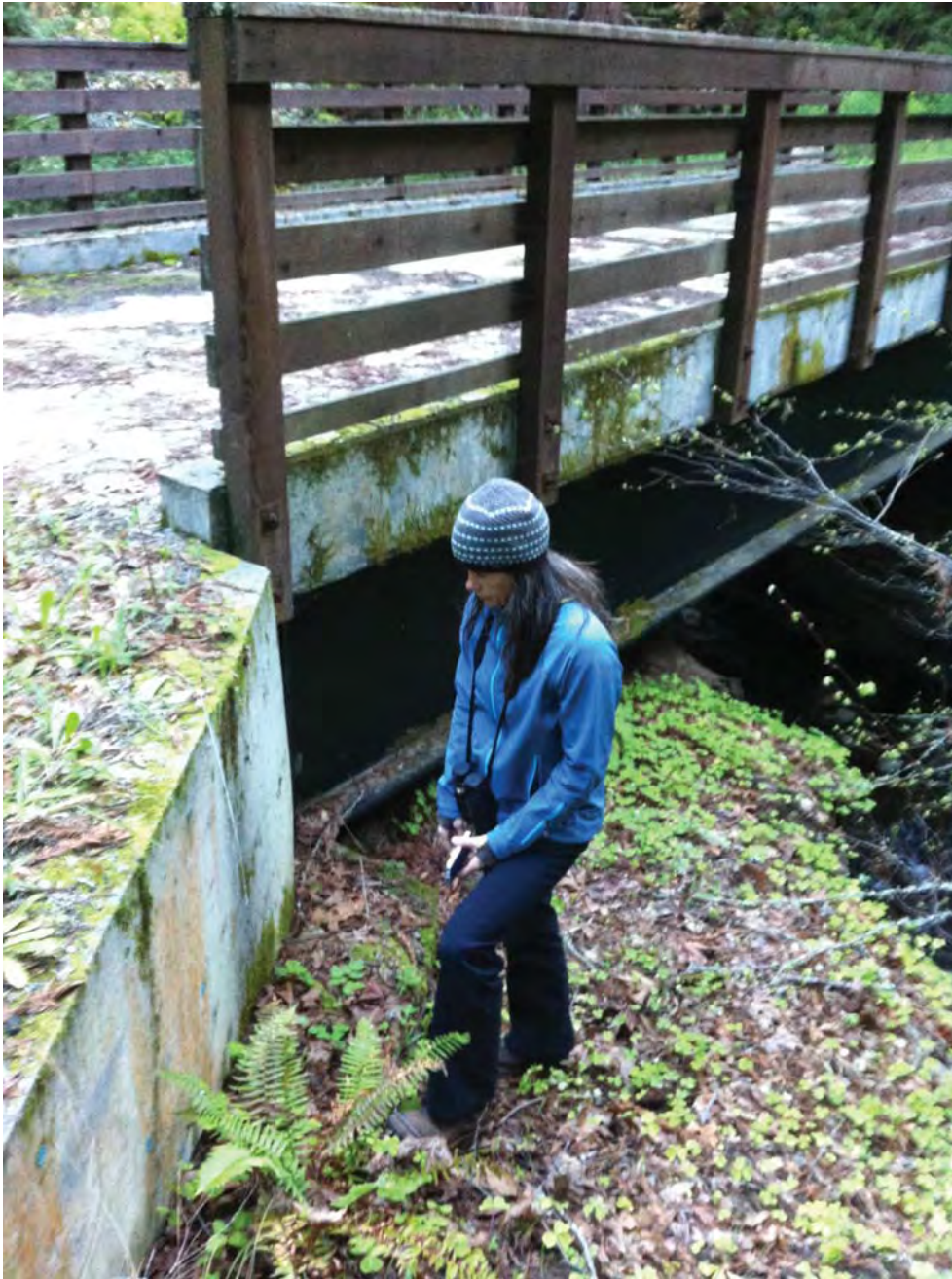
Exhibit B4: MROSD 2000 I-Beam Bridge on La Honda Creek
