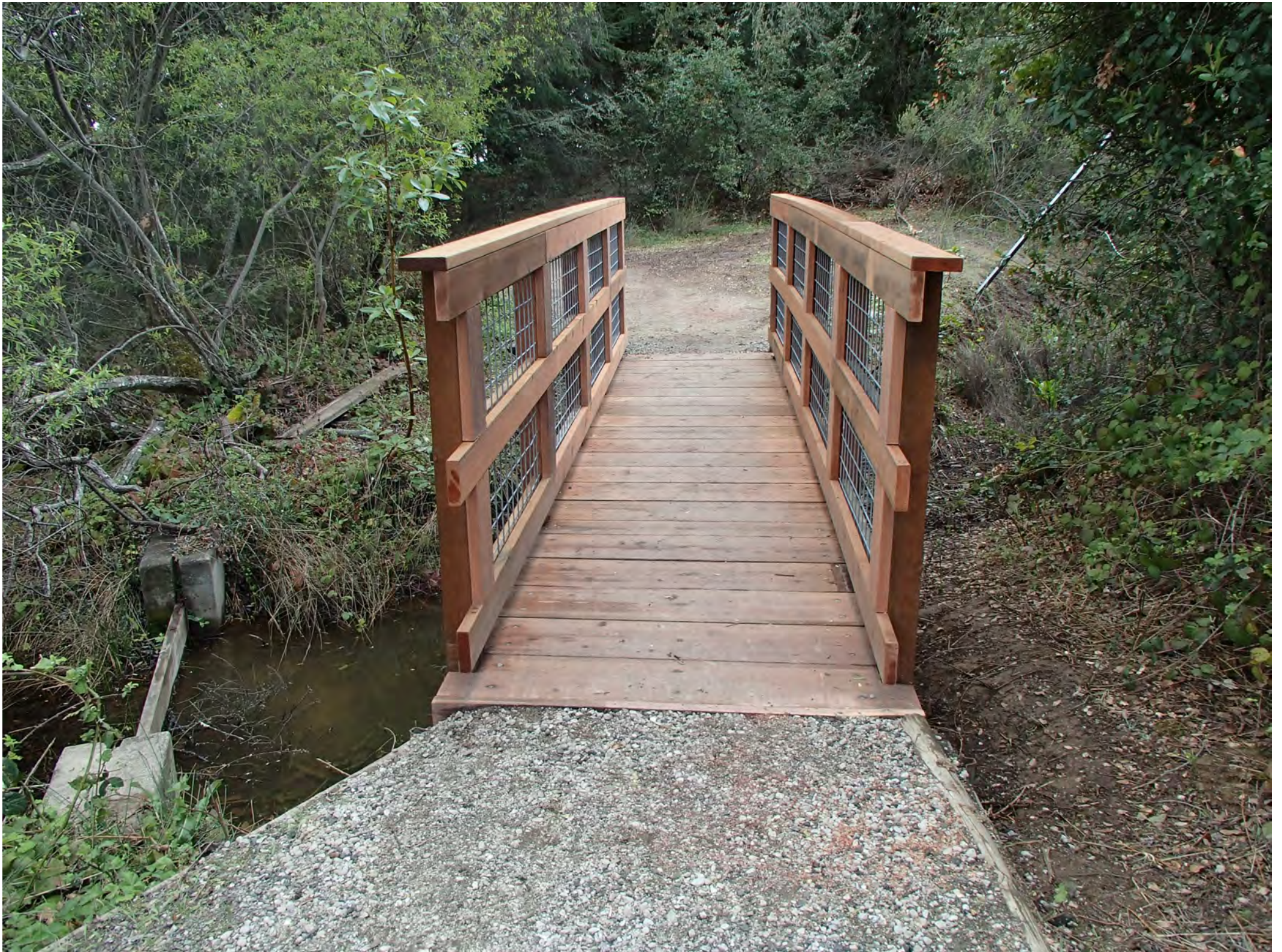
Exhibit C1: New Redwood and Welded Wire Mesh at Alpine Pond
