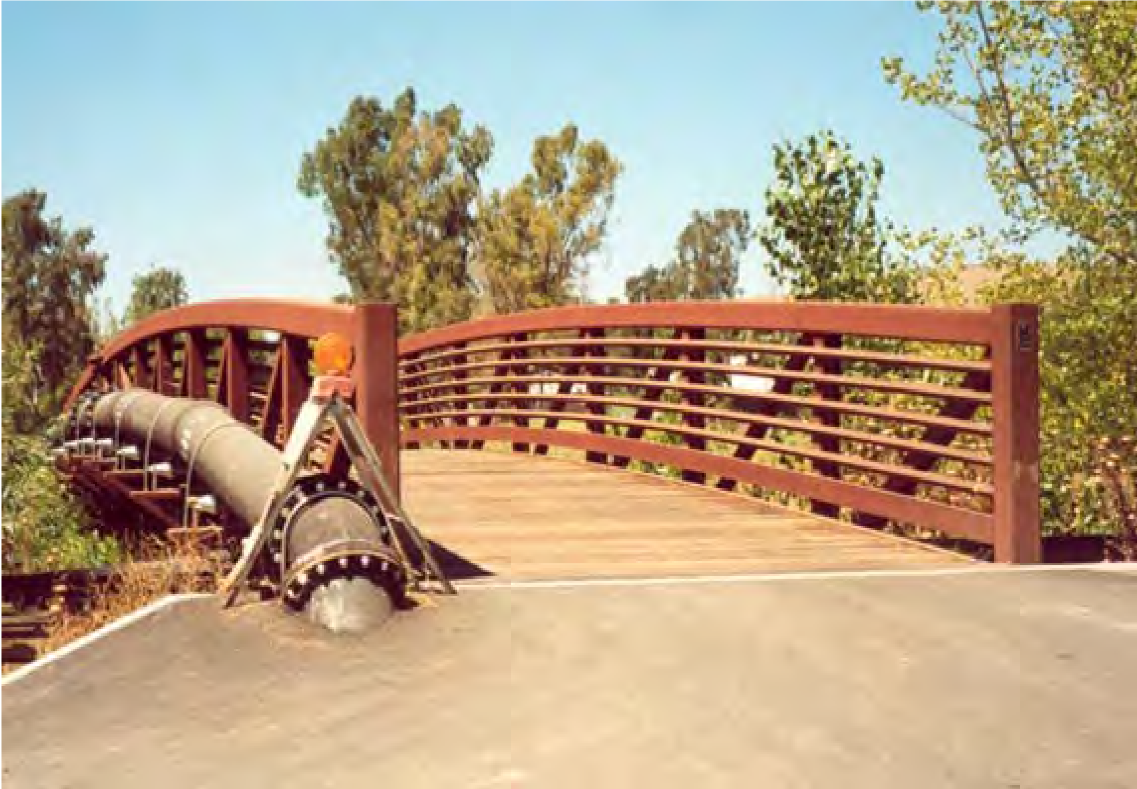
Exhibit C3: Prefabricated Truss Bridge with Manufacturer Installed Railings
