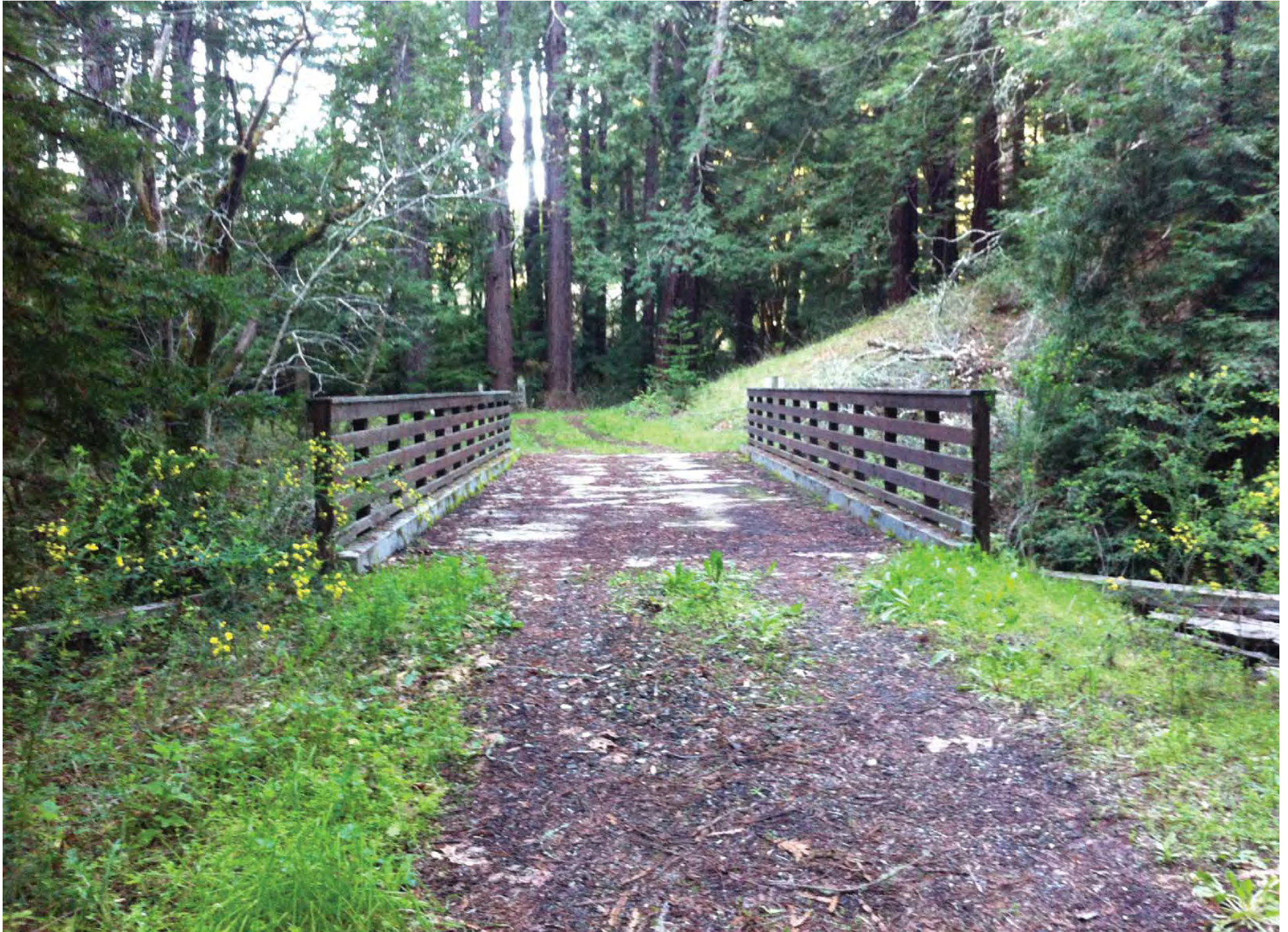
Exhibit B5: MROSD 2000 I-Beam Bridge on La Honda Creek
