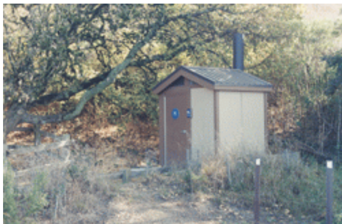
Typical vault toilet at the District's Open Space Preserves.
