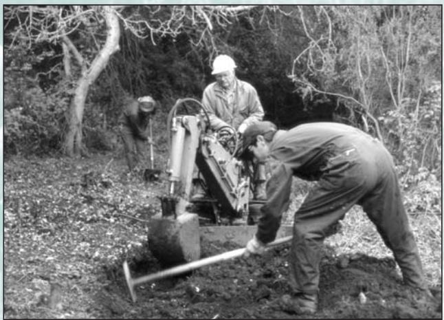
Michael works with trail building contractor to realign the Toyon Trail at Fremont Older Preserve.
