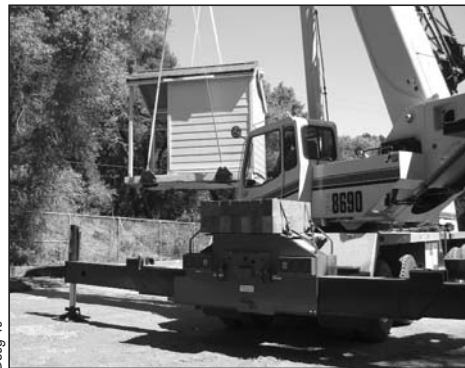
District contractor prepares to install the new vault toilet restroom at Pulgas Ridge Preserve.
