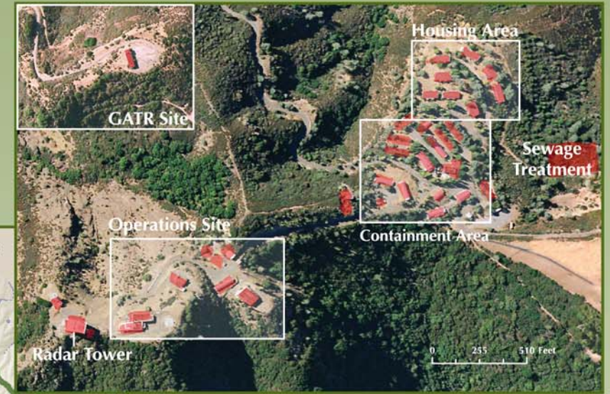
Many of the Air Force Station's 88 buildings contain deteriorated lead-based paint and friable asbestos.
