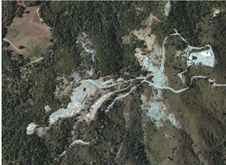
Figure 22. Former Mill Valley Air Force Station, 2010. FAA facility to the right, remaining foundations of other buildings to the left. (Source: Google Maps, 2010)
