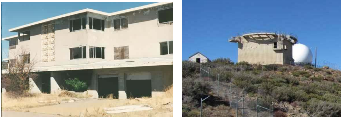
Figures 35 and 36. Former Mt. Laguna AFS, married enlisted quarters, ca. 1994 and the AN/FPS-26 height-finder radar/AN-FSS-7 SLBM radar tower with the FAA's ARSR-4 radar behind, 2009. (Source: http://www.radomes.org/museum/recent/MountLagunaAFSCA.html )
