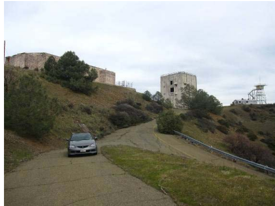
Figure 6. The road leading east to the Operations Building and radar towers. (Source: Page & Turnbull, February 2010).
