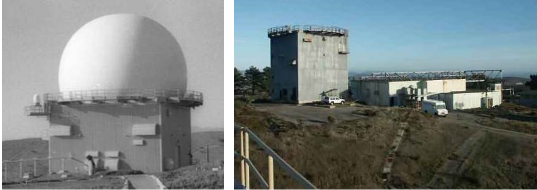
Figures 28 and 29. Former Cambria AFS—the AN/FPS-26A radome in 1968, and the AN/FPS-107 radar tower in 2004.
