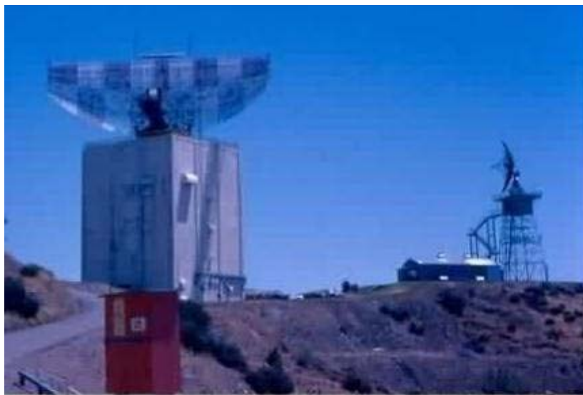
Figure 35. Buildings 102, 108, and 110 in about 1969. (Source: http://www.radomes.org/museum/ )
