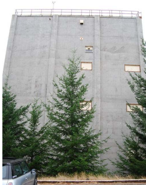
Figure 23. Point Arena AFS, AN/FPS-24 tower. (Source: http://www.uneceda-audio.com/776th/ )
