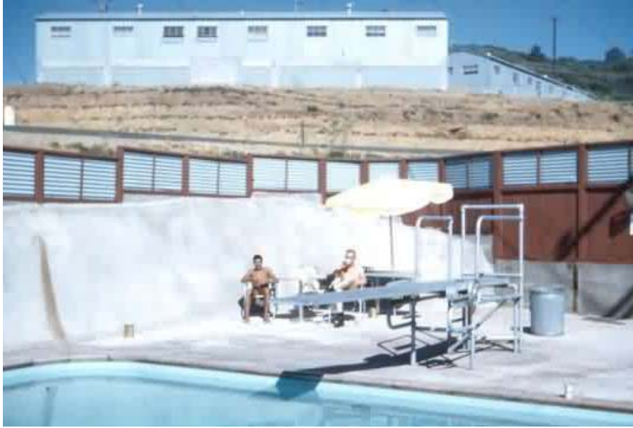
Figure 21. View east to the Orderly Building (Building 207) from the swimming pool, ca. 1959-1960. (Source: http://www.radomes.org/museum/ )
