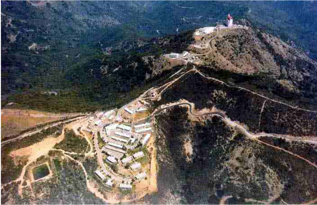
Figure 2. Aerial, Almaden Air Force Station, ca. 1960s. Cantonment in the western foreground and radars to the east (several steel barracks buildings were removed in the 1970s). (Source: http://www.radomes.org/museum/ )
