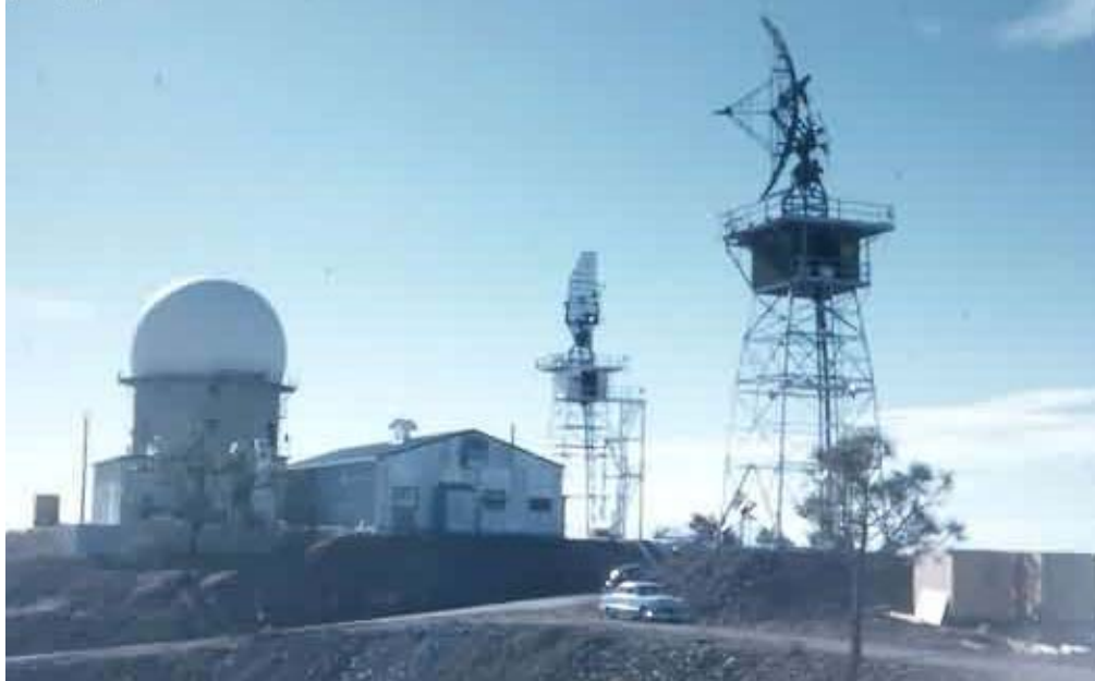
Figure 11. Operations (Building 100) with AN/FPS-20 radome to the left, AN/MPS-14 radar to at center, and AN/FPS-6A to the far right, ca. 1959-1960. (Source: http://www.radomes.org/museum/ )
