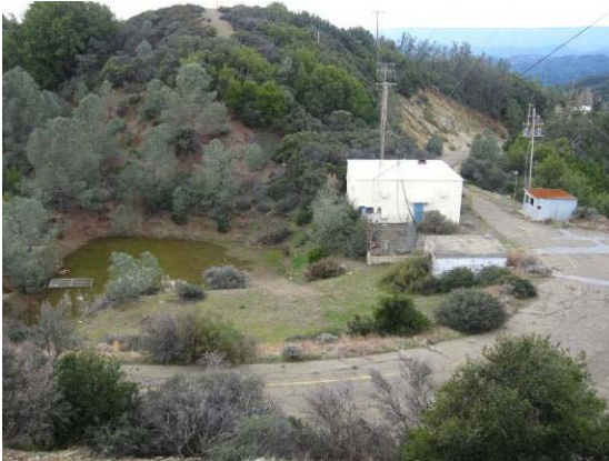
Figure 5. The TELCO, Security, Diesel Fuel Pump, and spill containment pool at the east end of the operations area. (Source: Page & Turnbull, February 2010).
