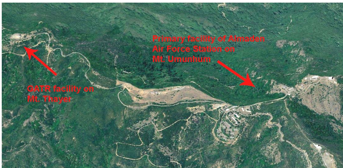
Figure 3. Aerial, former Almaden Air Force Station on Mt. Umunhum in relation to GATR facility on Mt Thayer, ca. 2010. (Source: Microsoft Corporation, www.bing.com )
