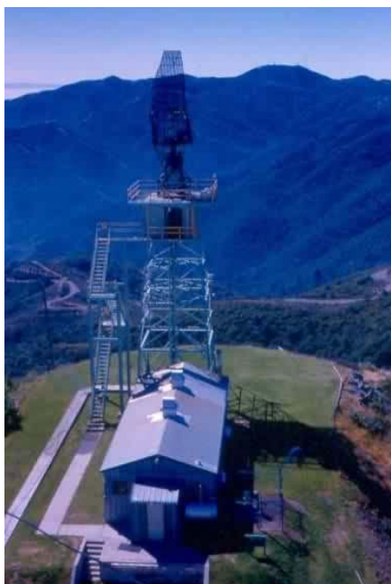
Figure 36. Building 108 and 110, ca. 1969. (Source: http://www.radomes.org/museum/ )
