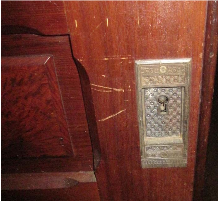
Hardware detail at the pocket doors. Photograph B. Maley, March 2013.
