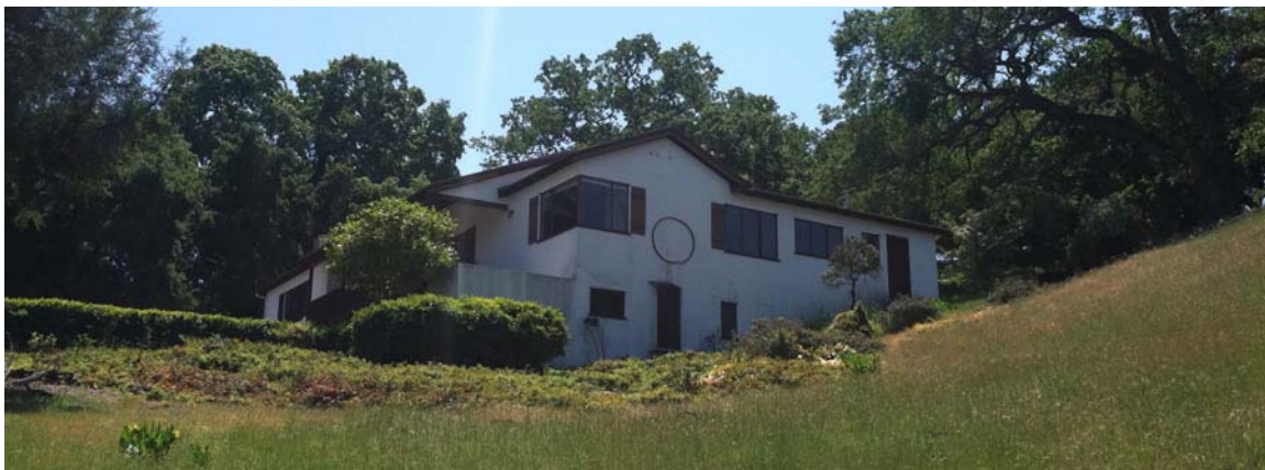
Below: The side elevation of the Alpine Road house showing how it is built into the hillside, viewed from the entry drive below. Photograph B. Maley, March 2013.
