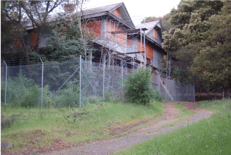
Above: Section of the internal road system that runs in front of the Hawthorn House. Photograph Denise Bradley, March 2013.
