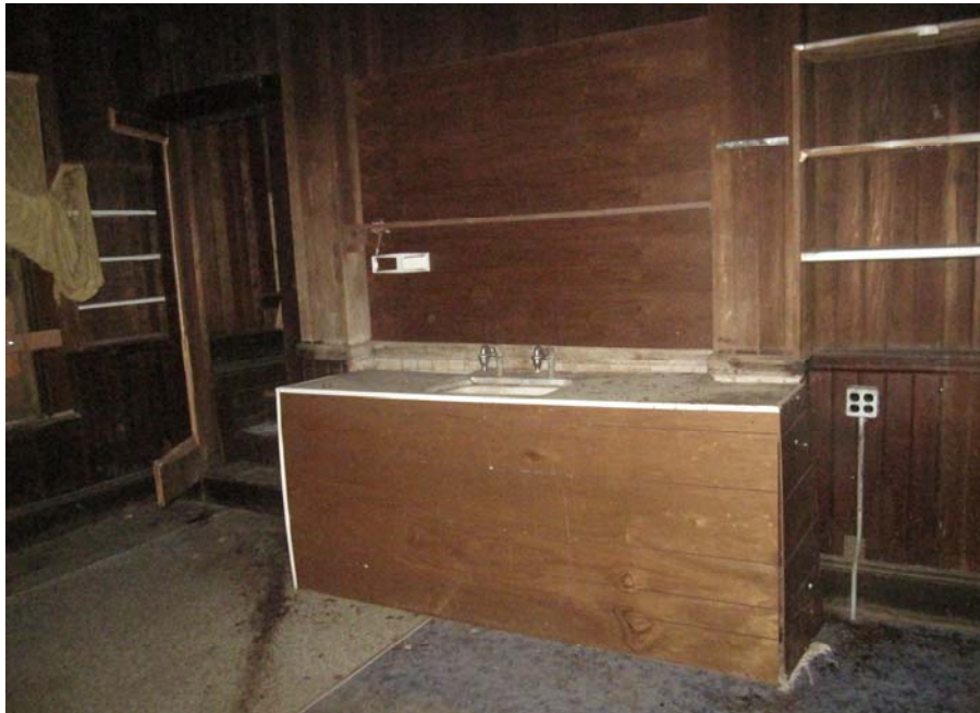
The interior of the Cottage, showing the alterations that have occurred. Photograph B. Maley, March 2013.
