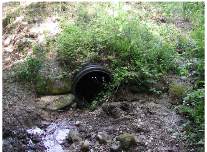
MP 16: 24" culvert inlet. Culvert is undersized and
