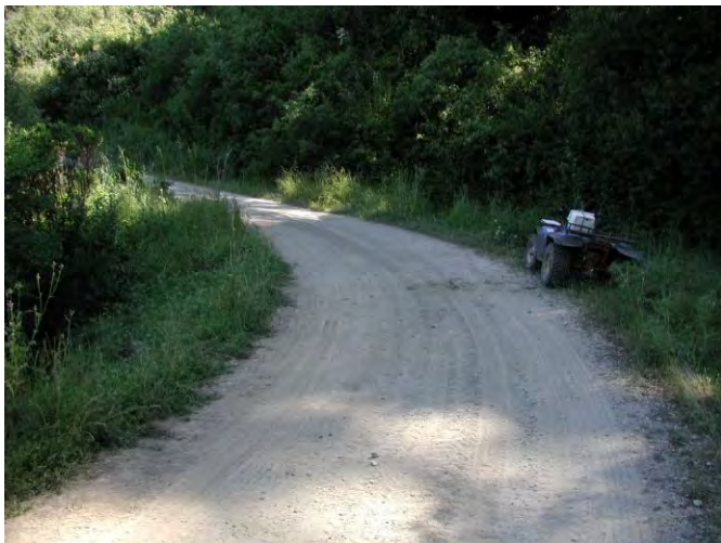
MP 16: General site photograph
