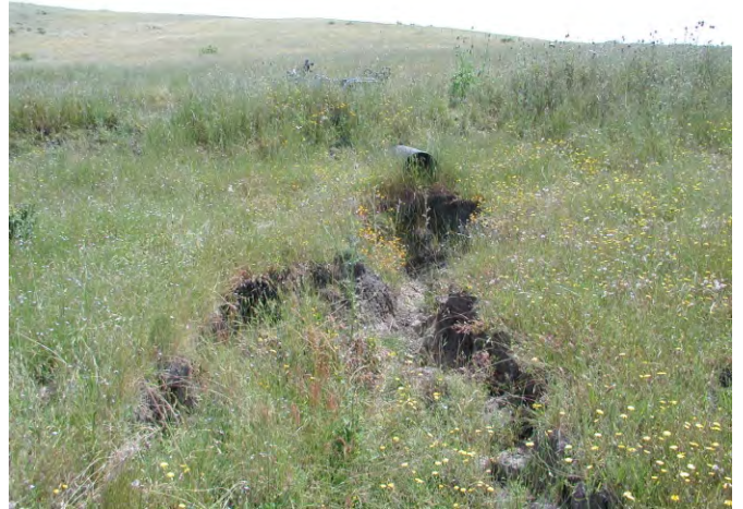
MP 50: Gully at outlet of culvert
