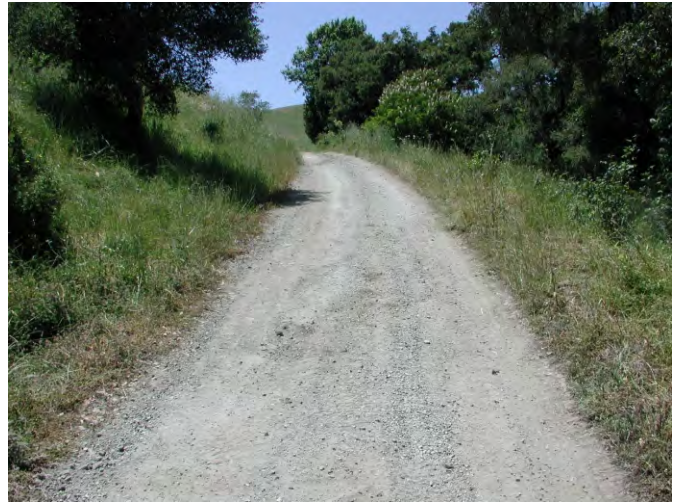
MP 15: Long inboard ditch
