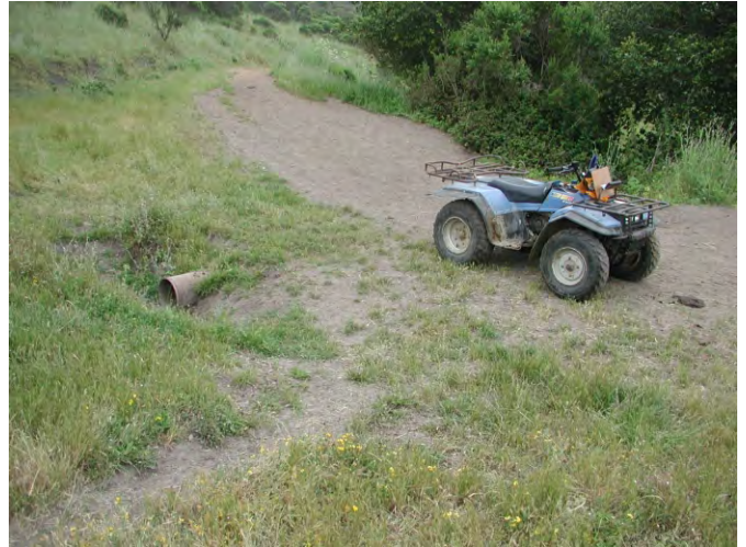
MP 45: Culvert inlet
