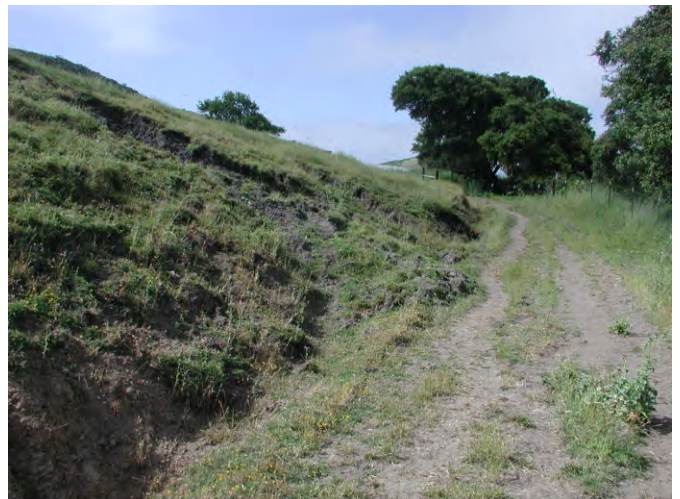
MP 46: Cutbank failure slumped onto road.
