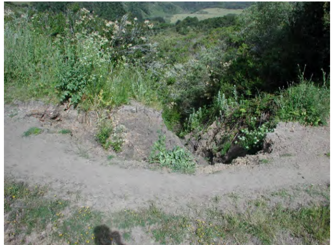
MP46: Gully narrowing road.
