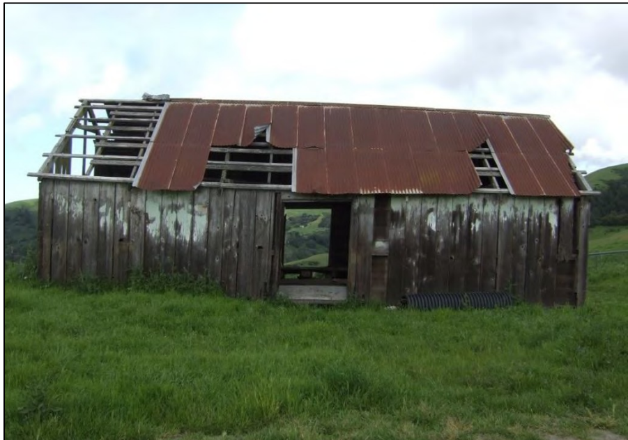
Figure 8. GZR-1, small barn, east elevation (Recommend DEMO)
