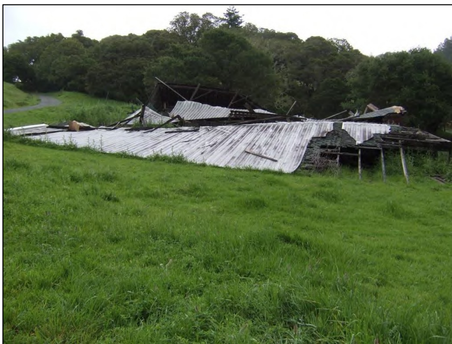
Figure 24. LFR-4, collapsed hay barn (Recommend DEMO)
