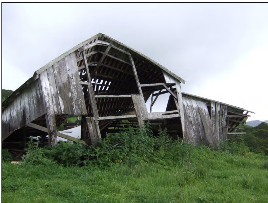
Figure 20. UFR-3, collapsed barn, north elevation (Recommend DEMO)
