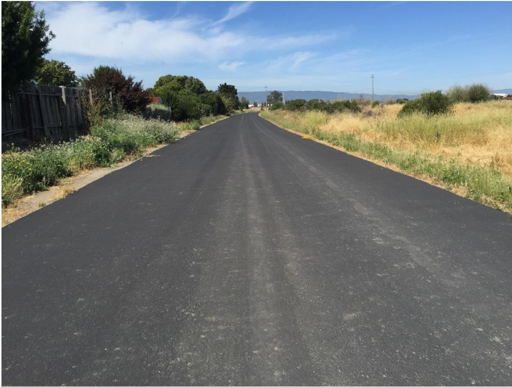
Photo 1: View of SFPUC Service Road, looking west toward University Avenue
