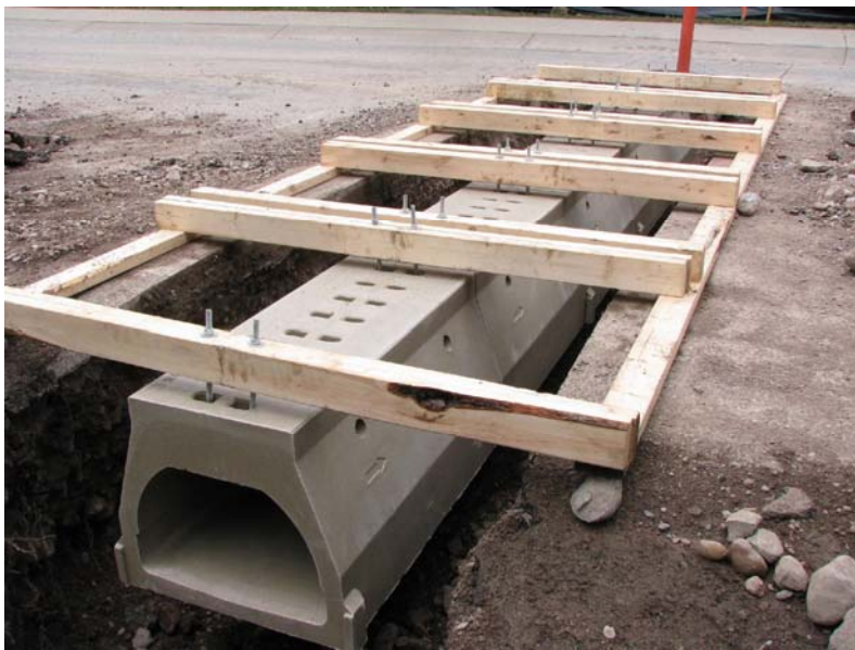
Herp (amphibian and reptile) crossing under construction - Waterton National Park, Alberta, Canada
