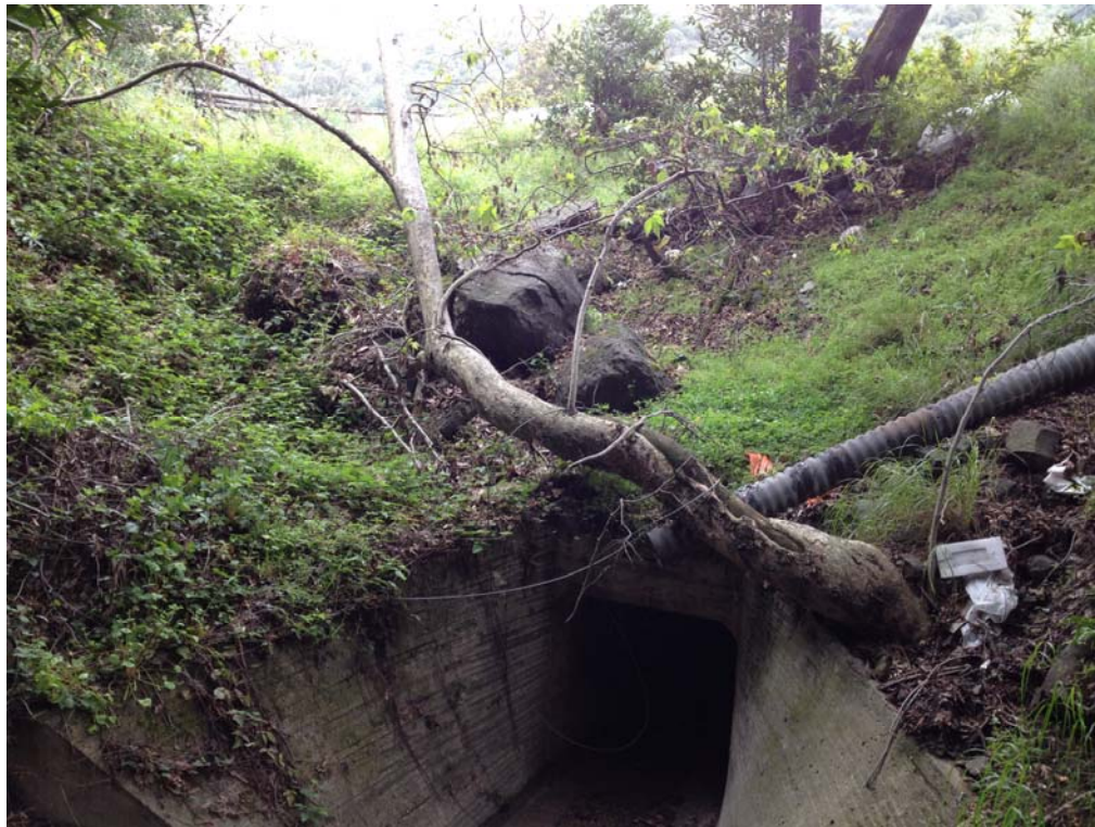
Ravine Culvert Inlet
