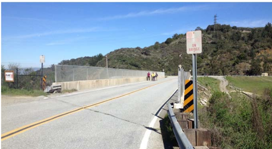
Type 4: Bridge over the spillway: a parallel bike/pedestrian bridge would be required
