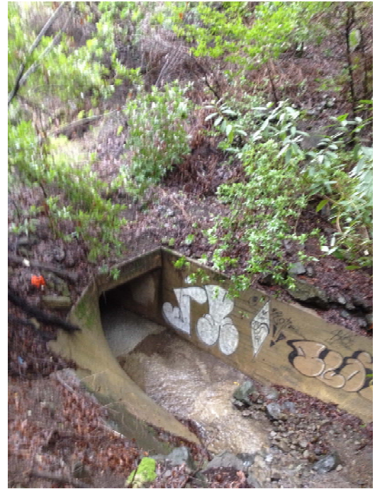
Existing culvert inlet on west side
