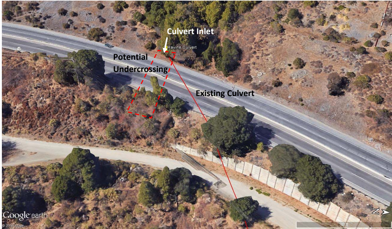
Figure 15: Ravine Culvert Site Photos
