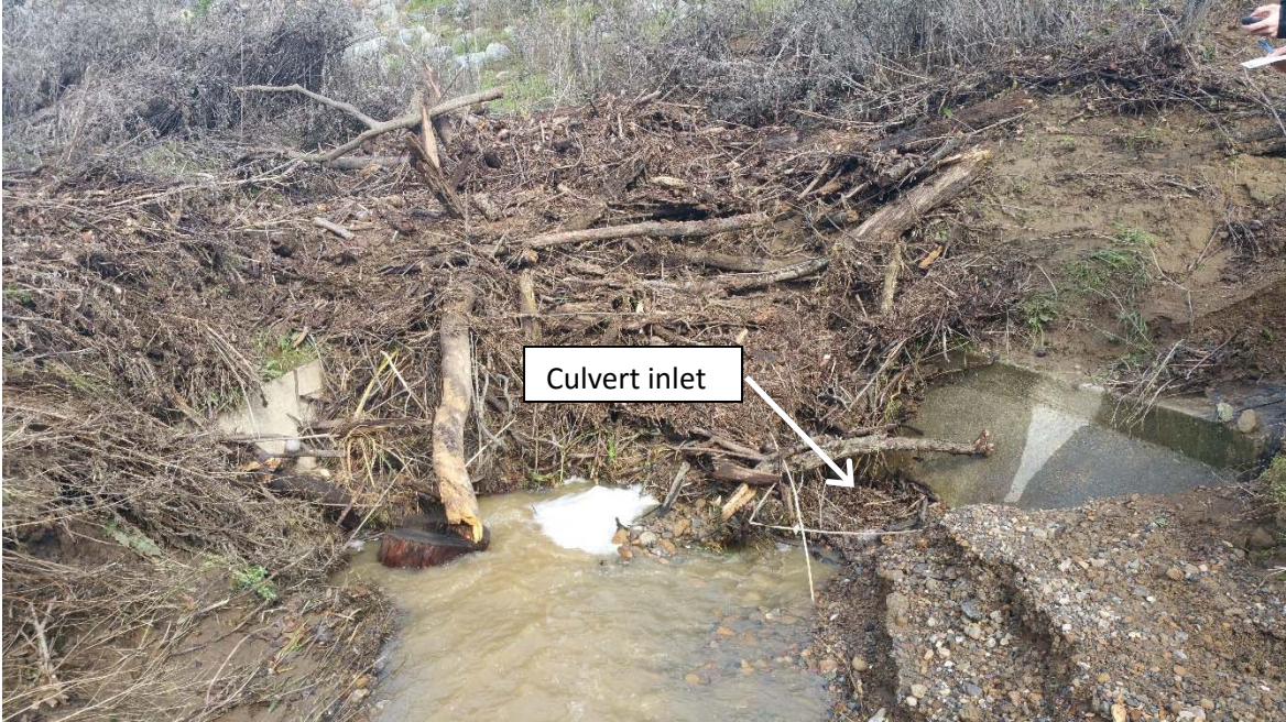
Black Creek Culvert Inlet, March 7, 2016
