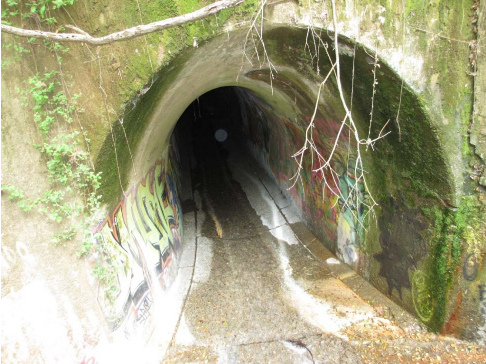
Briggs Creek culvert inlet
