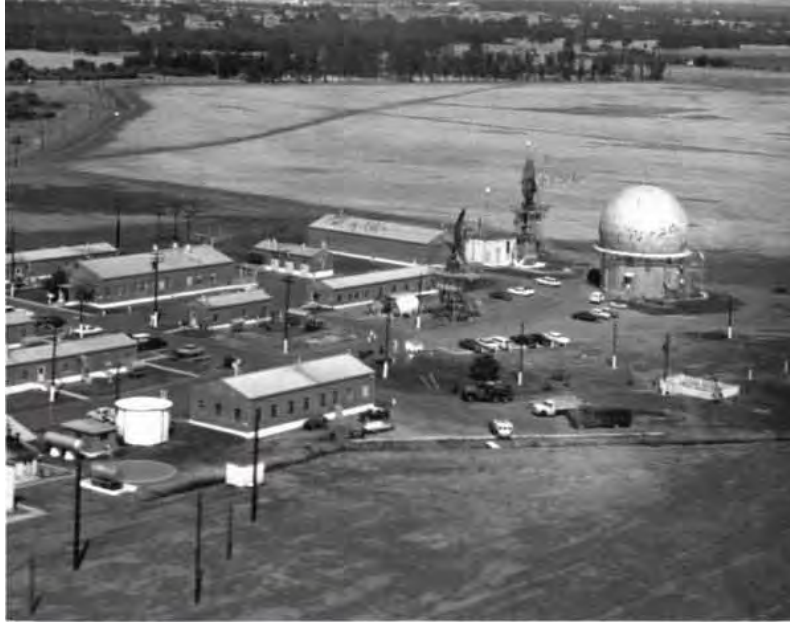
Red Bluff Air Force Station, n.d. This AFS used metal buildings for administration, logistical support, and housing.
