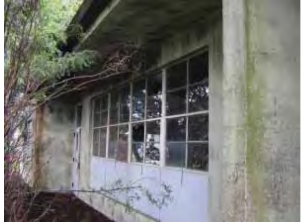
Building 245 Recreation: west wing, detail of west facade (Page & Turnbull, February 2010)
