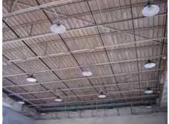
Building 245 Recreation: detail of gymnasium ceiling (Page & Turnbull, February 2010)
