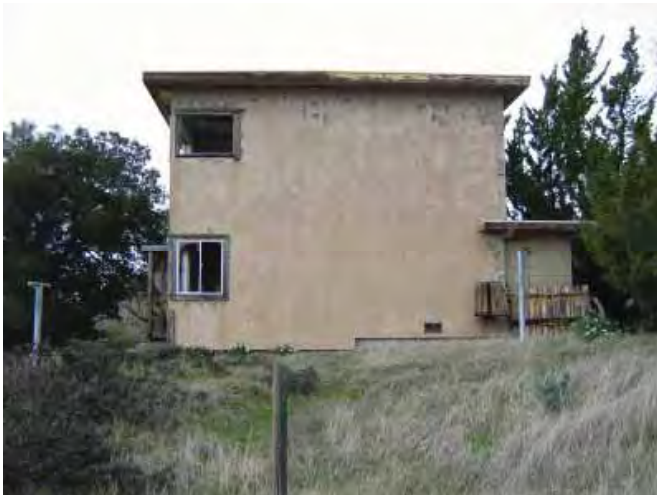
Building 515: Triplex Apartment, looking north toward south façade. (Page & Turnbull, February 2010)
