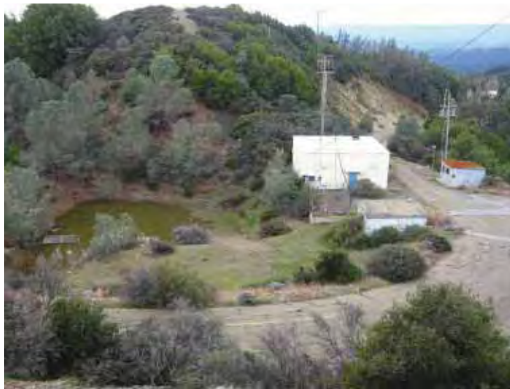
TELCO toward the right in bird's eye view, looking southwest. (Page & Turnbull, February 2010)
