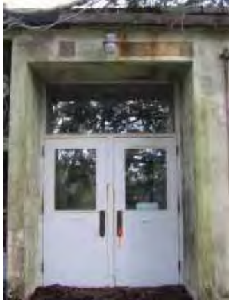
Building 245 Recreation: west wing, detail of entry (Page & Turnbull, February 2010)
