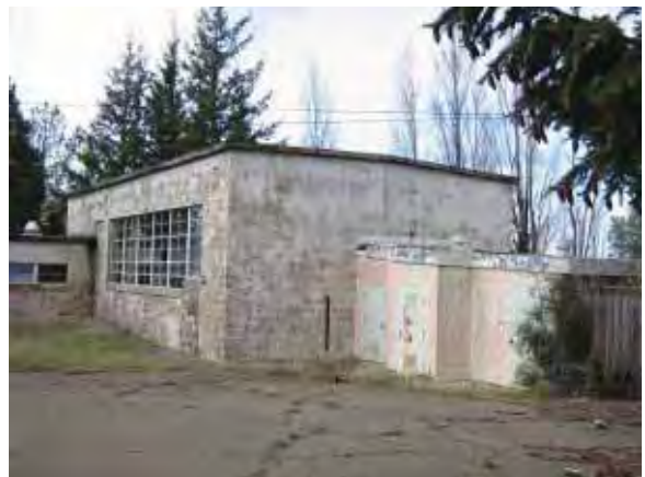
Building 245 Recreation: central (gym) wing, south and east facades. Note Building 276: Bath House is attached at lower right. (Page & Turnbull, February 2010)
