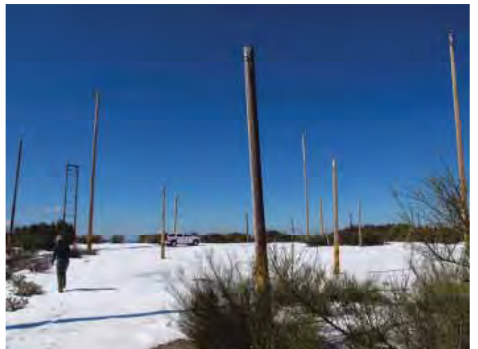
Wood poles for lower-frequency antennae surrounding Building 700 on Mt. Thayer, looking northwest. (Page & Turnbull, February 2011)
