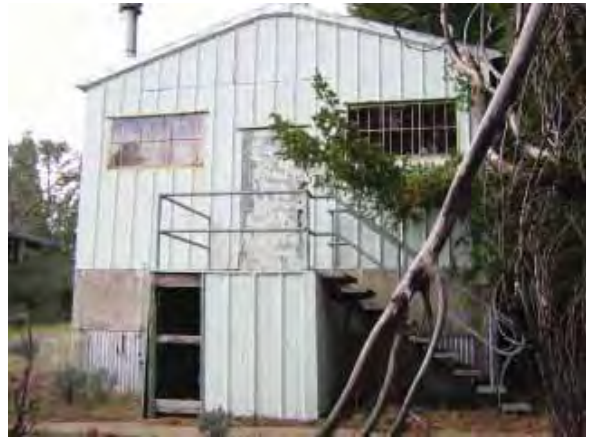
Building 233: Barracks, detail of entrance on south facade (Page & Turnbull, February 2010)
