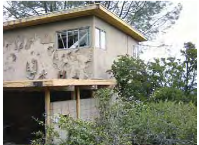
Building 517: Triplex Apartment, looking southwest toward north and east façades. (Page & Turnbull, February 2010)
