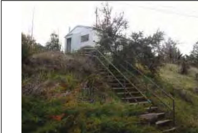
Building 213: Dispensary, view southwest of stair leading to rear (east) facade (Page & Turnbull, February 2010)
