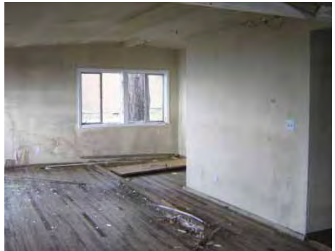
Building 516: Commander's House, interior. (Page & Turnbull, February 2010)
