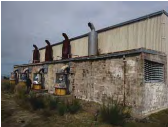
Building 112: electrical Power Station, southwest façade, looking northeast. (Page & Turnbull, February 2010)
