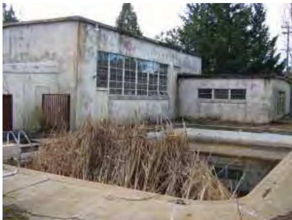
Building 245 Recreation: central (gym) wing, north facade (Page & Turnbull, February 2010)
