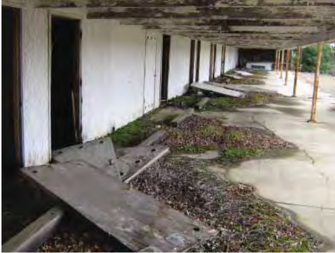
Building 505: Carport, looking southeast. (Page & Turnbull, February 2010)
