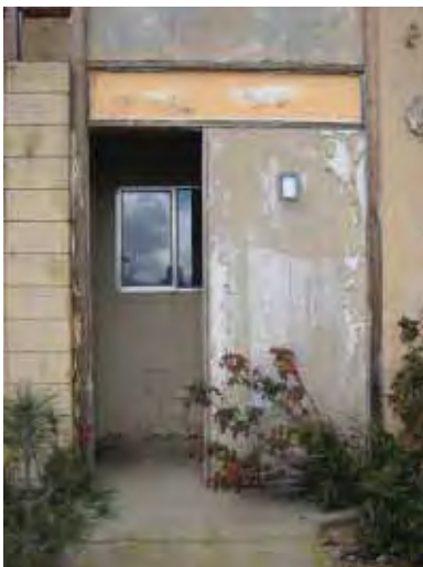
Building 512: Fourplex Apartment, looking north toward ground floor of rear façade. (Page & Turnbull, February 2010)
