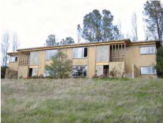
Building 512: Fourplex Apartment, looking north toward rear façade. (Page & Turnbull, February 2010)
