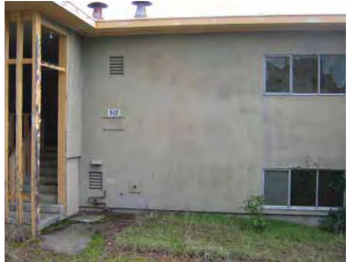
Building 512: Fourplex Apartment, looking south toward primary façade. (Page & Turnbull, February 2010)
