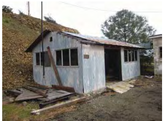
Semi-attached unnumbered building, looking northwest. (Page & Turnbull, February 2010)
