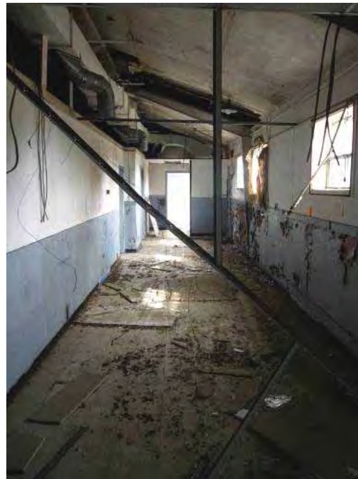
Building 119: CE Maintenance Shop interior. (Page & Turnbull, February 2010)
