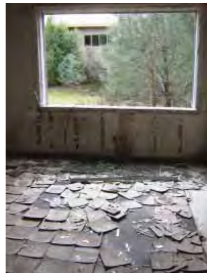
Building 511: Fourplex Apartment, interior. (Page & Turnbull, February 2010)
