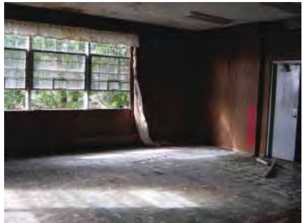
Building 245 Recreation: interior room (Page & Turnbull, February 2010)
