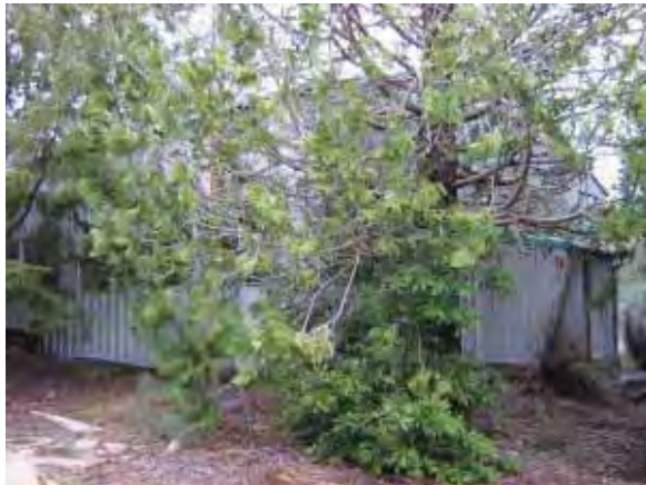
Building 225: Airman's Dining Hall, south and west facades (Page & Turnbull, February 2010)
