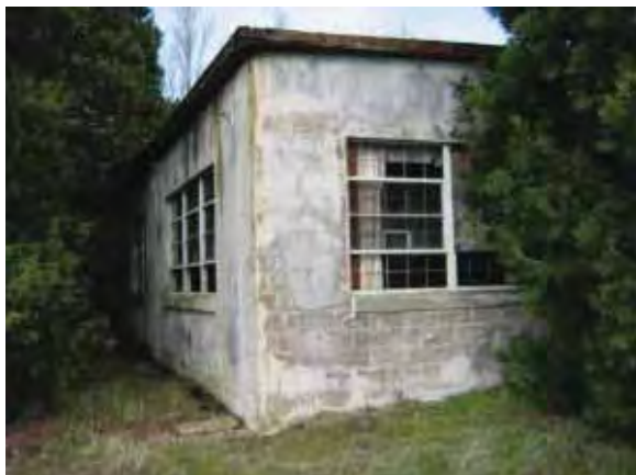
Building 245 Recreation: west wing, southwest corner (Page & Turnbull, February 2010)
