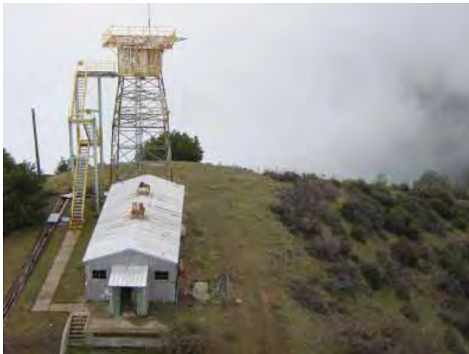
Building 108: Radar Tower MPS-14 and Building 110: Training, looking south from Building 102. (Page & Turnbull, February 2010)
