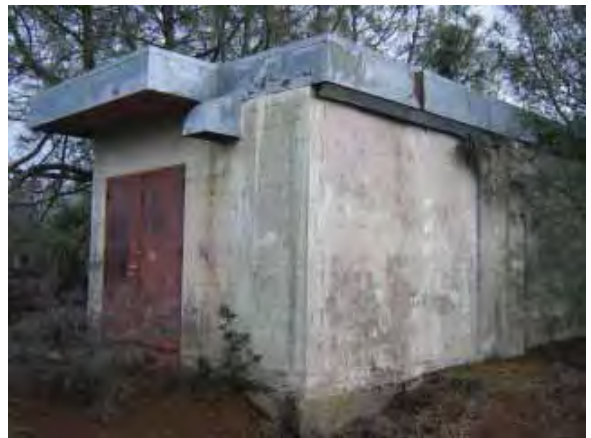
Building 217: Bowling Alley, north and west facades (Page & Turnbull, February 2010)
