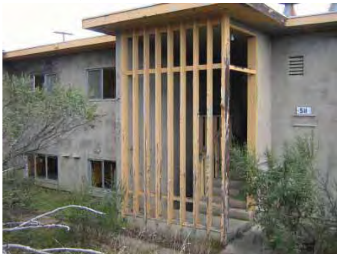
Building 511: Fourplex Apartment, looking southeast toward primary façade. (Page & Turnbull, February 2010)
