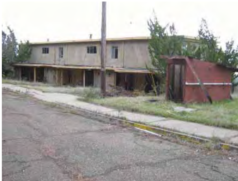
Building 508: Fire Hose House, view looking south. Note Building 515: Triplex Apartment to the southeast. (Page & Turnbull, February 2010)
