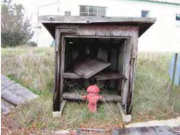
Building 215: Fire Hose House, south façade. (Page & Turnbull, February 2010)
