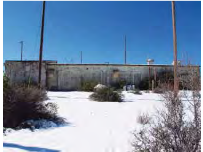
Building 700: Communications Transmitter/Receiver (GATR), northeast façade, looking southwest. (Page & Turnbull, February 2011)
