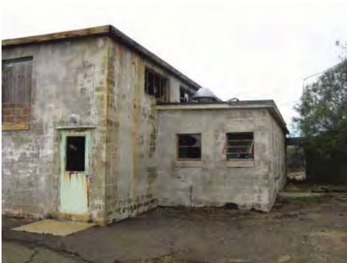
Building 120, partial view of primary façade. (Page & Turnbull, February 2010)
