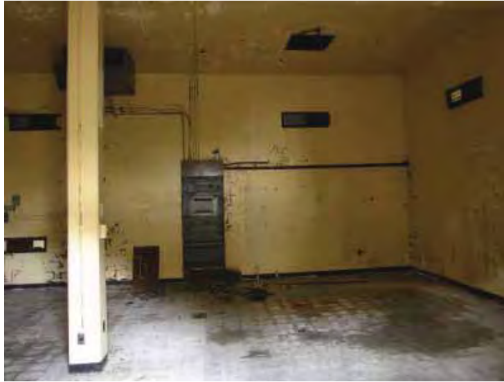
TELCO, interior. (Page & Turnbull, February 2010)
