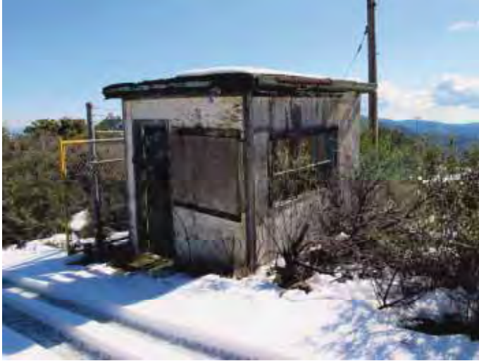
Building 715/722: Security Sentry House, north and west façades, looking southeast. (Page & Turnbull, February 2011)
