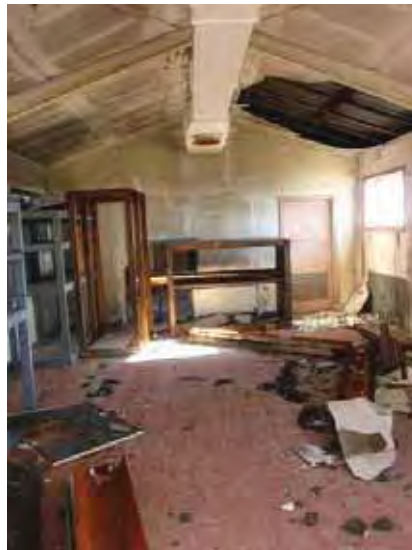
Building 110: Training, interior view looking south. (Page & Turnbull, February 2010)
