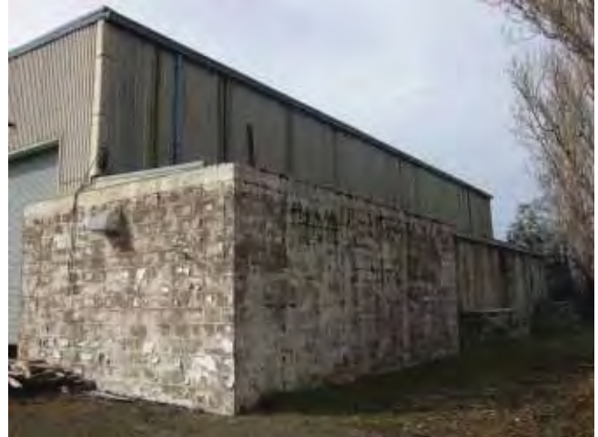
Building 112: electrical Power Station, northeast façade, looking northwest. (Page & Turnbull, February 2010)
