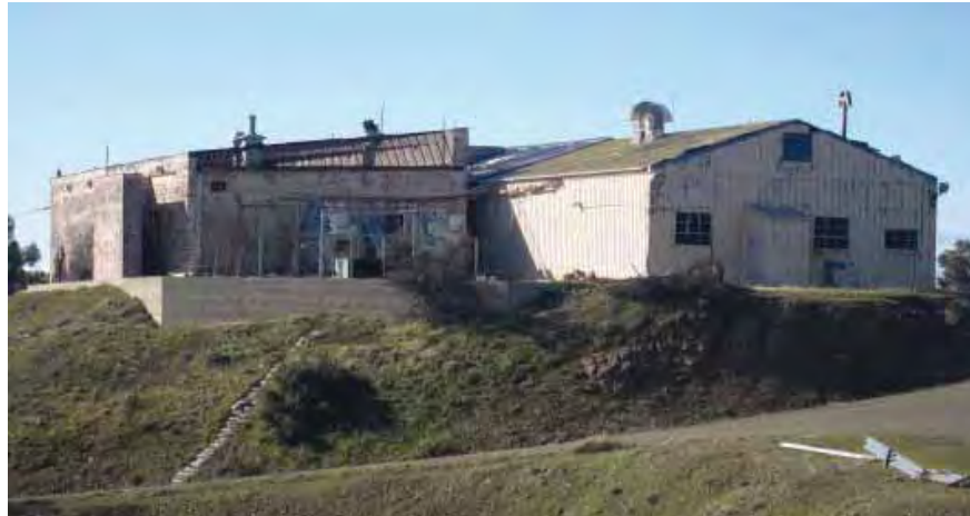
Building 100, looking northwest toward the northeast metal section and southwest CMU section prior to abatement. (Page & Turnbull, February 2010)
