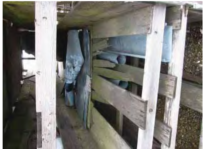
Building 114: Sheets and pipes inside. (Page & Turnbull, February 2010)
