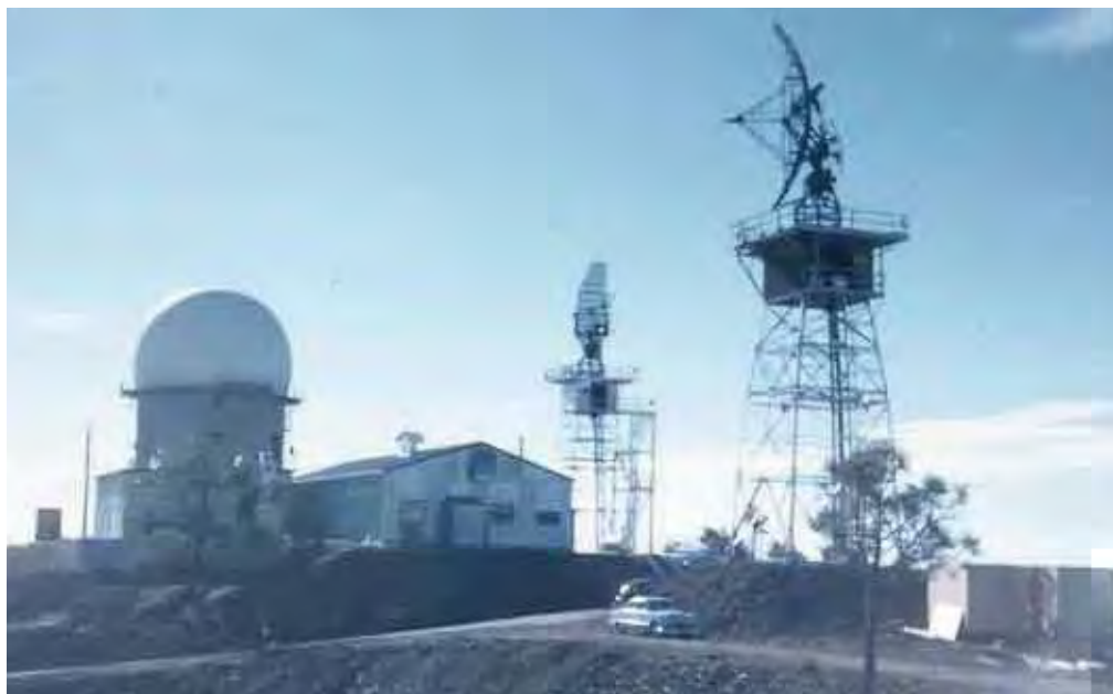
Operations (Building 100) with AN/FPS-20 radome to the left, AN/MPS-14 radar to at center, and AN/FPS-6A to the far right, ca. 1959-1960. (Source: http://www.radomes.org/museum/ )
