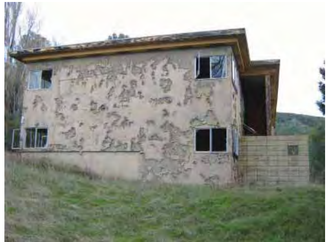
Building 511: Fourplex Apartment, looking east toward west façade. (Page & Turnbull, February 2010)
