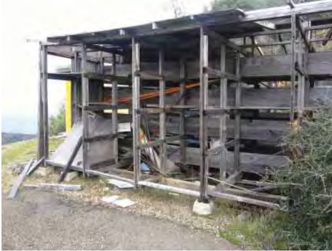
Building 114: South (primary) façade. (Page & Turnbull, February 2010)
