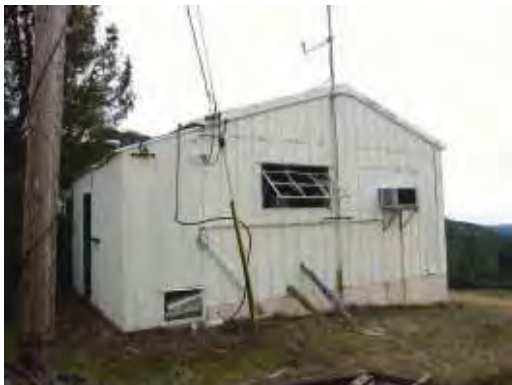
Building 205: Bachelor Officers' Quarters, detail of the west facade. Note shed-roofed section at left. (Page & Turnbull, February 2010)
