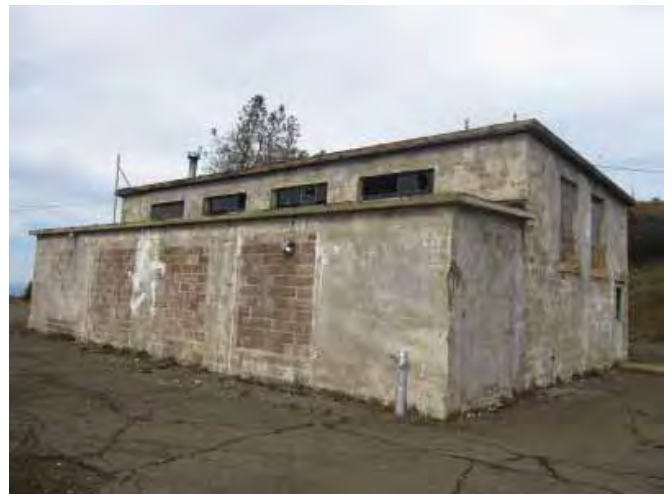
Building 120, southeast façade, looking northwest. (Page & Turnbull, February 2010)
