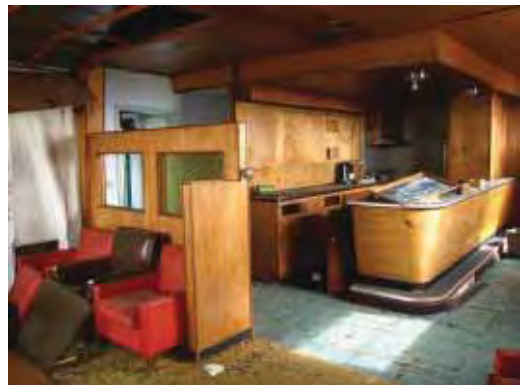
Building 205: Bachelor Officers' Quarters, interior lounge area and bar. (Page & Turnbull, February 2010)
