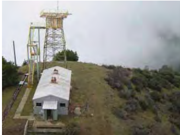
Building 110: Training, looking south from Building 102. (Page & Turnbull, February 2010)
