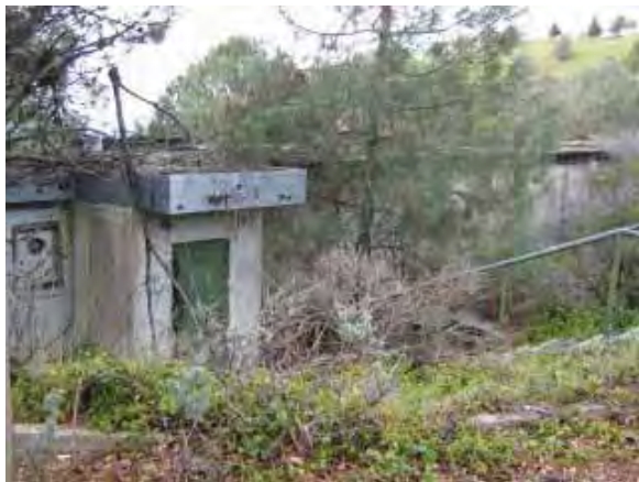
Building 217: Bowling Alley, detail of primary (east) facade (Page & Turnbull, February 2010)
