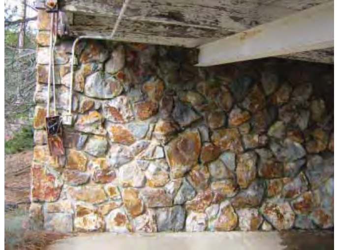
Building 505: Carport, northeast stone wall. (Page & Turnbull, February 2010)
