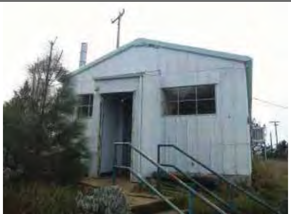
Building 213: Dispensary, rear (east) facade (Page & Turnbull, February 2010)
