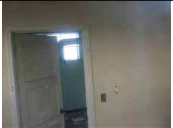
Building 213: Dispensary, view of interior door taken through window (Page & Turnbull, February 2010)
