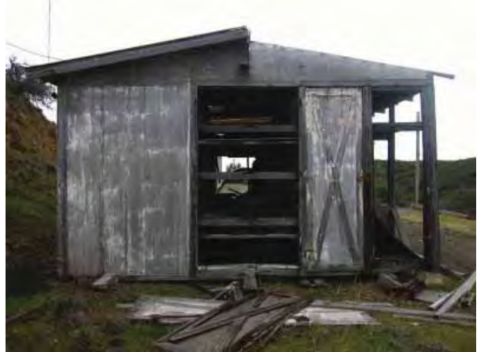
Building 114: West façade. (Page & Turnbull, February 2010)
