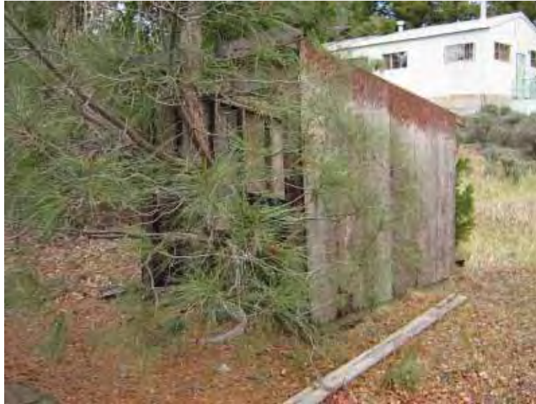
Building 232: Fire Hose House, south and west facades (Page & Turnbull, February 2010)
