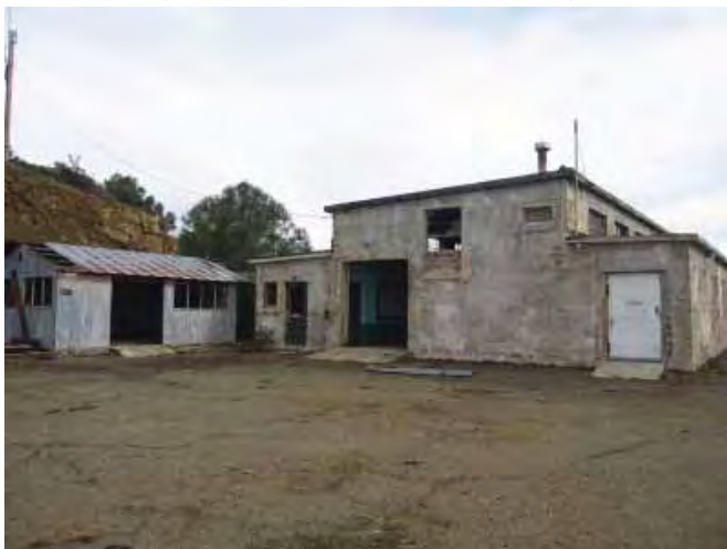
Building 120, southwest façade, looking northeast. (Page & Turnbull, February 2010)
