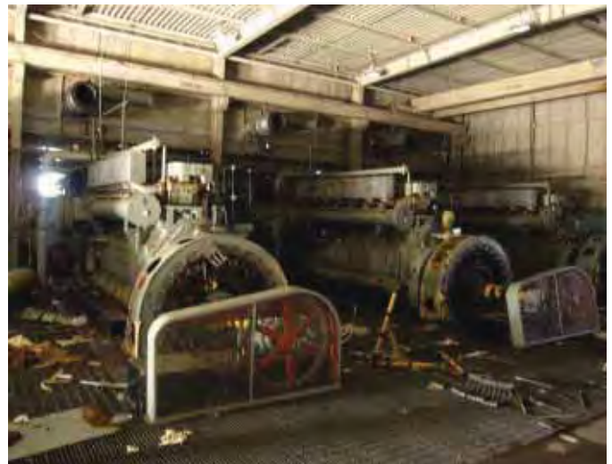
Building 112: Electrical Power Station, interior view looking northwest. (Page & Turnbull, February 2010)
