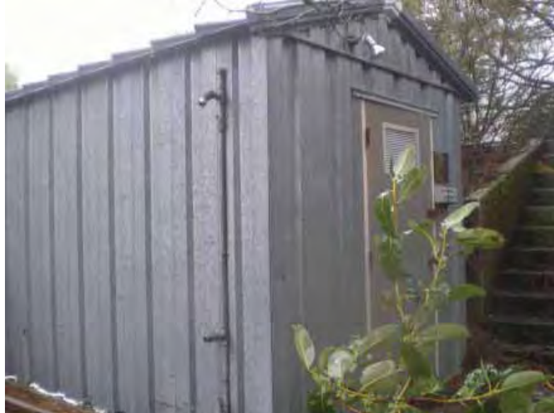
East and south façades. (MROSD, 2011)
