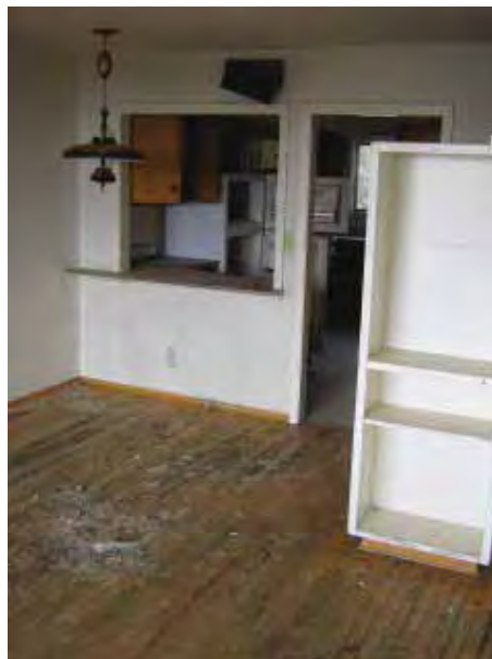
Building 514: Fourplex Apartment, interior. (Page & Turnbull, February 2010)
