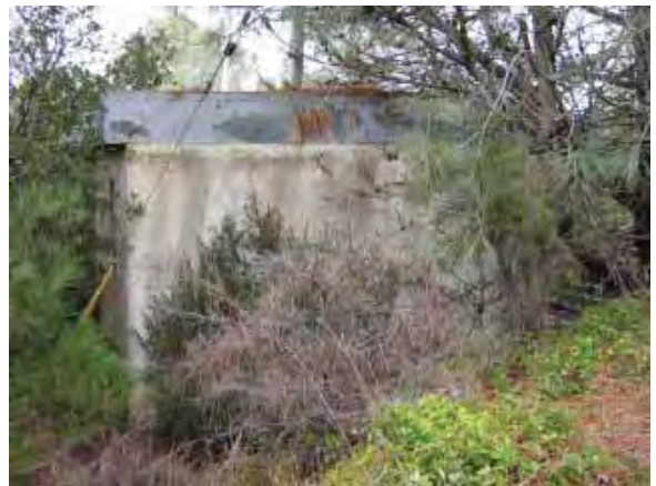
Building 217: Bowling Alley, south facade (Page & Turnbull, February 2010)
