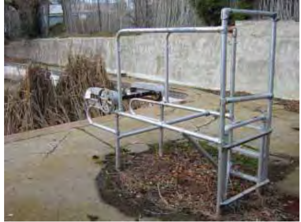
Building 275: Swimming Pool, diving platform at east end (Page & Turnbull, February 2010)
