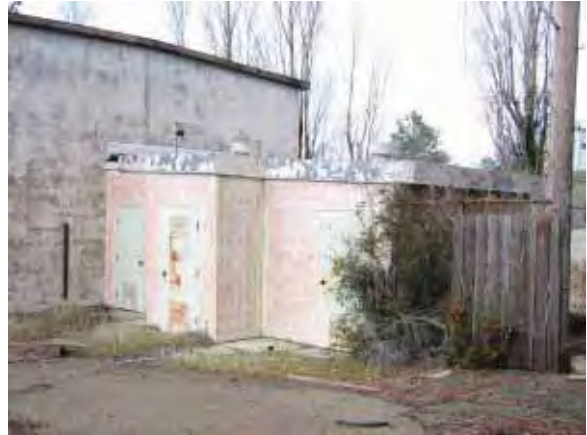
Building 276 Bath House, south façade. (Page & Turnbull, February 2010)
