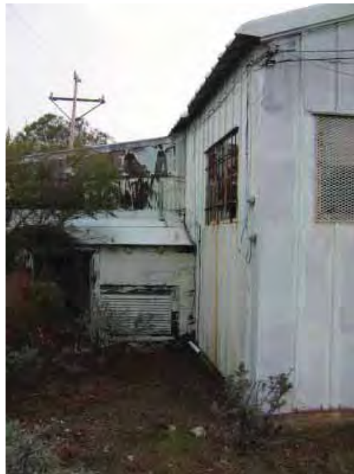
Building 212: NCO Open Mess, looking east at north addition. (Page & Turnbull, February 2010)
