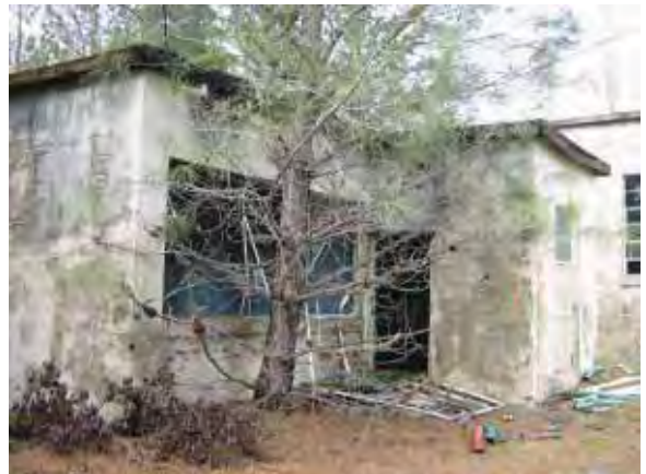
Building 245 Recreation: west wing, east facade entry (Page & Turnbull, February 2010)
