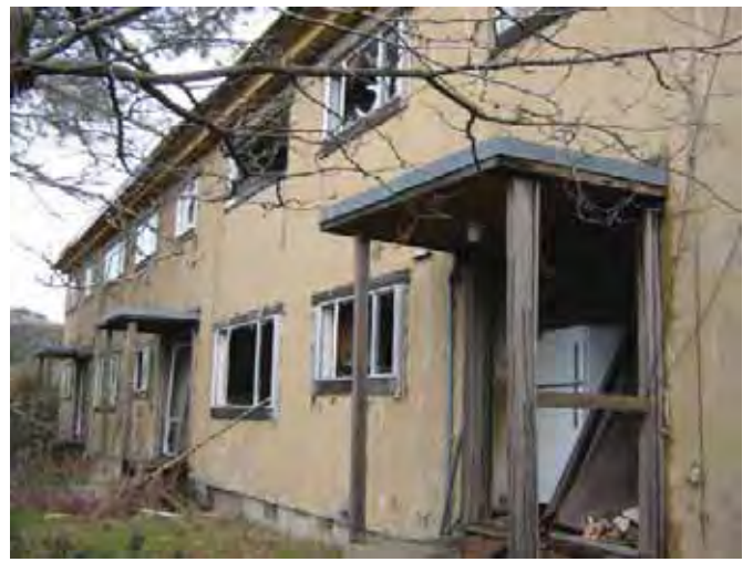
Building 517: Triplex Apartment, looking northeast toward west (rear) façade. (Page & Turnbull, February 2010)
