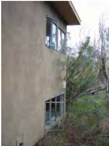
Building 510: Fourplex Apartment, looking south toward northwest façade. (Page & Turnbull, February 2010)
