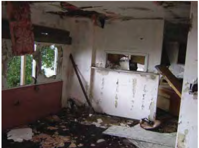
Building 515: Triplex Apartment, interior. (Page & Turnbull, February 2010)
