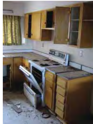
Building 510: Fourplex Apartment, kitchen. (Page & Turnbull, February 2010)
