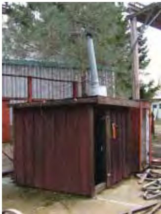
Building 275: Swimming Pool, Detail of wood enclosure for pump and water heater. (Page & Turnbull, February 2010)
