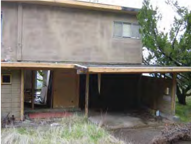
Building 515: Triplex Apartment, looking northwest toward the north end of the primary façade. (Page & Turnbull, February 2010)
