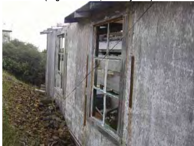
Building 114: North (rear) façade. (Page & Turnbull, February 2010)
