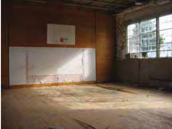
Building 245 Recreation: gymnasium interior (Page & Turnbull, February 2010)
