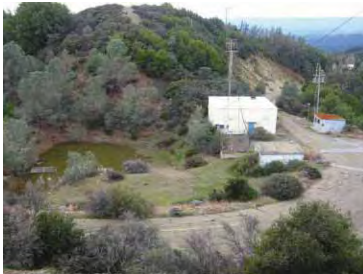
Building 115: Sentry House at right in bird's eye view, looking southwest. (Page & Turnbull, February 2010)
