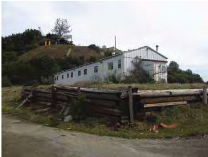
Building 119: CE Maintenance Shop, looking northeast toward south and west facades. (Page & Turnbull, February 2010)
