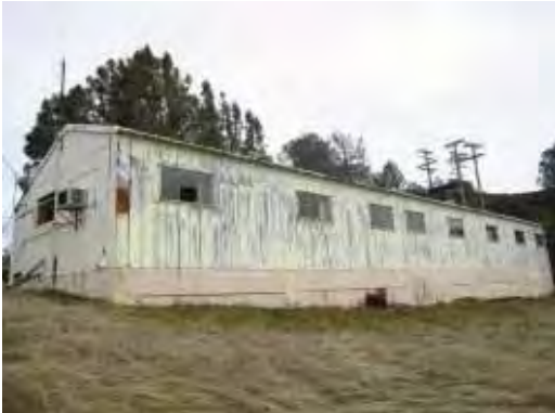
Building 205: Bachelor Officers' Quarters, looking northeast toward the west and south facades. (Page & Turnbull, February 2010)
