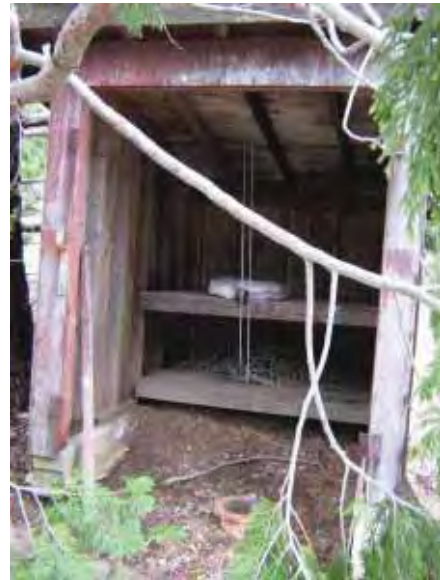
Building 234: Fire Hose House, detail of interior (Page & Turnbull, February 2010)
