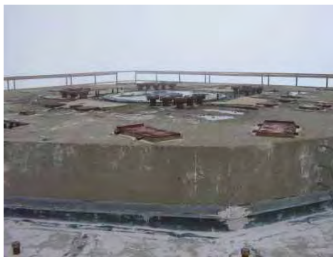
Center footing for the radar sail on the roof. (Page & Turnbull, February 2010)
