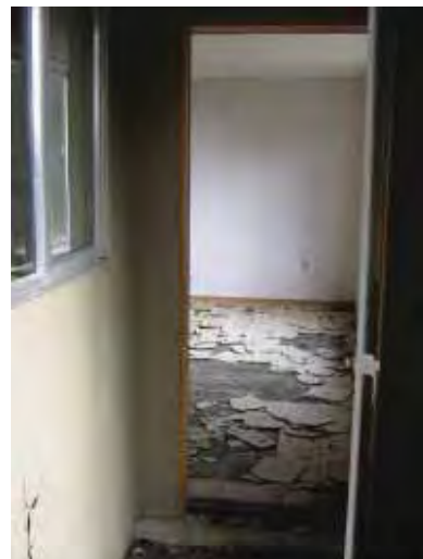
Building 512: Fourplex Apartment, interior. (Page & Turnbull, February 2010)
