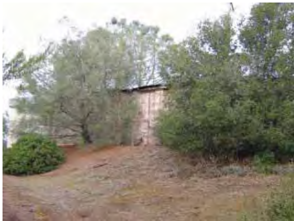
Building 217: Bowling Alley, west facade (Page & Turnbull, February 2010)
