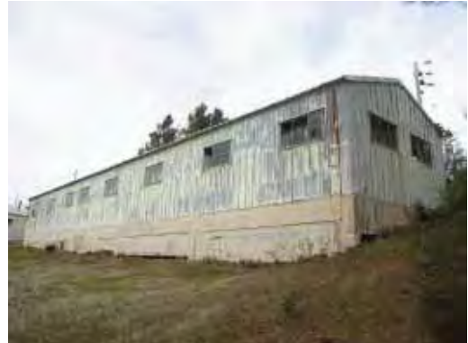
Building 205: Bachelor Officers' Quarters, view of south and east facades. (Page & Turnbull, February 2010)
