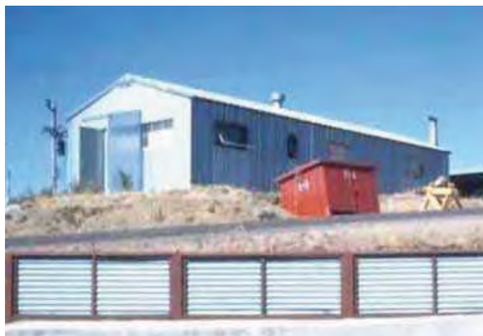
Building 213: Dispensary, ca. 1959-1960.
