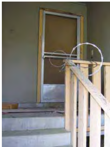
Building 513: Fourplex Apartment, looking south to unit entrance. (Page & Turnbull, February 2010)
