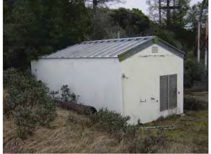
Building 200: Water Pump Station, north and east façades, looking southeast. (Page & Turnbull, February 2010)
