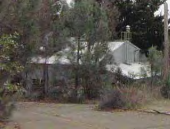
Building 225: Airman's Dining Hall, east and north facades (Page & Turnbull, February 2010)
