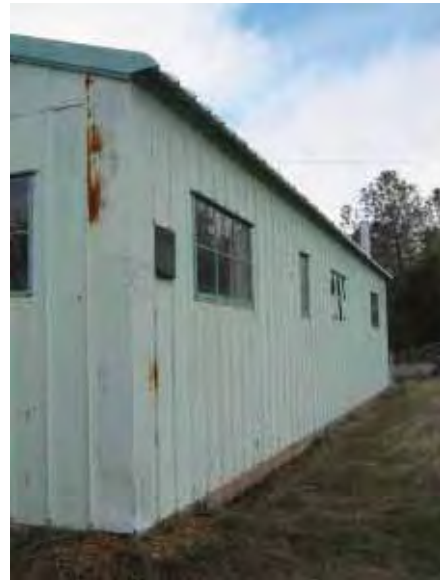
Building 213: Dispensary, north facade (Page & Turnbull, February 2010)
