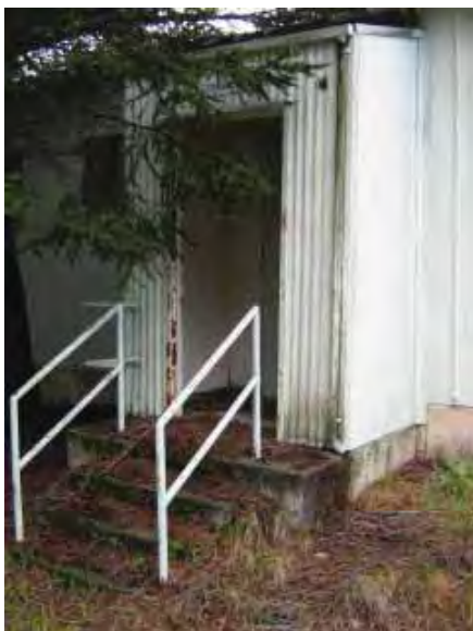
Building 233: Barracks, entry near southeast corner (Page & Turnbull, February 2010)
