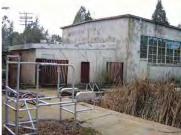
Building 276: Bath House, North and south facades adjacent to pool. (Page & Turnbull, February 2010)
