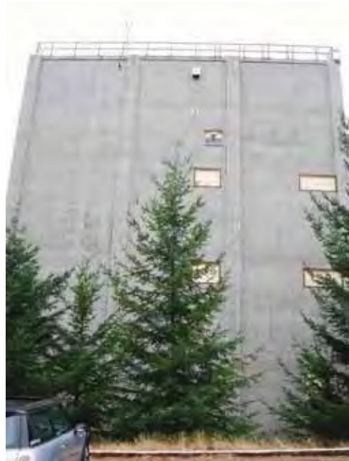
Point Arena AFS, AN/FPS-24 tower.
