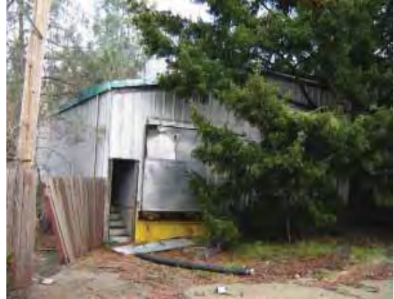
Building 225: Airman's Dining Hall, loading dock at northwest corner (Page & Turnbull, February 2010)
