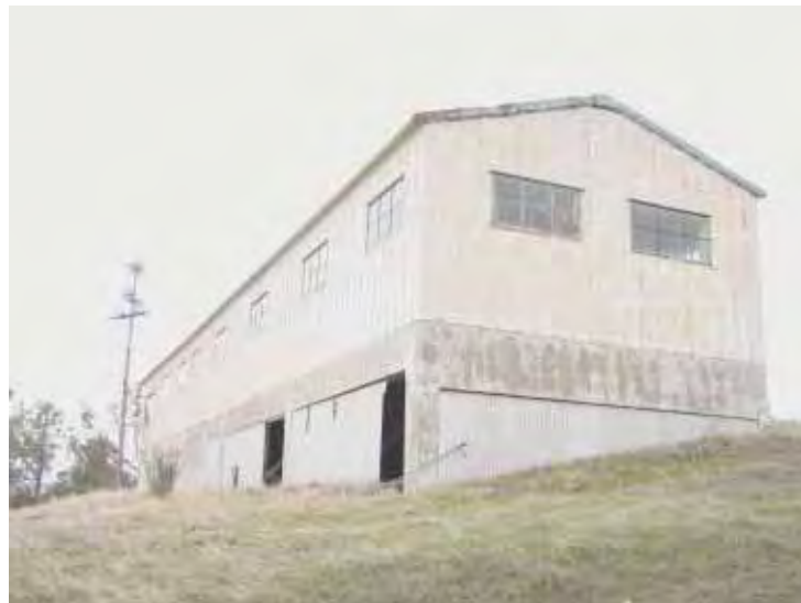
Building 207: Squadron Headquarters/Orderly Room, south and west facades. (Page & Turnbull, February 2010)
