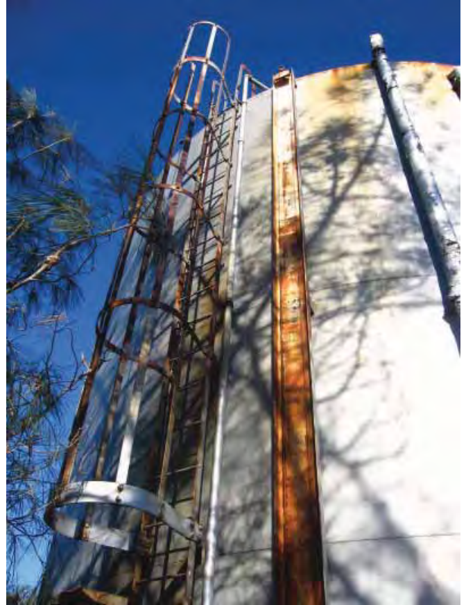
Building 884B: Water Tank, view northwest. (Page & Turnbull, February 2010)
