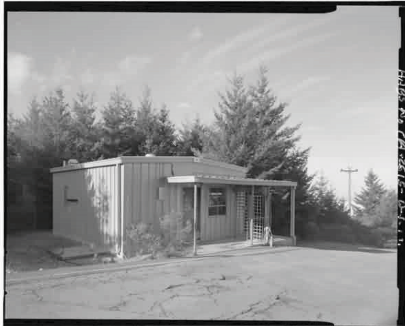
Operations Guard House at Mill Valley AFS, n.d. (Source : Radomes. http://www.radomes.org/museum/recent/MillValleyAFSCA.html )
