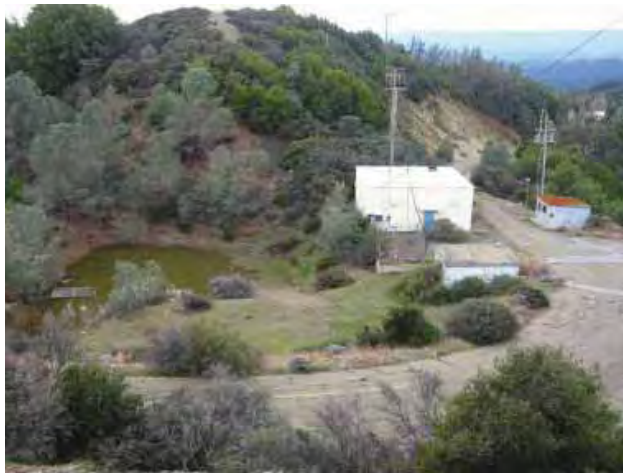
Building 118: Diesel Fuel Pump toward the right (in front of TELCO building) in bird's eye view, looking southwest. (Page & Turnbull, February 2010)
