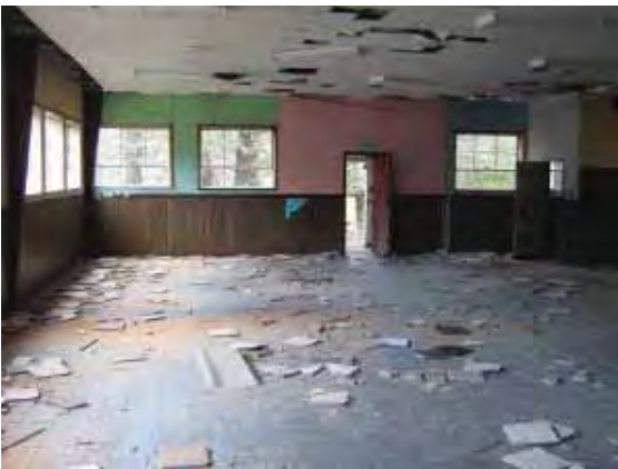
Building 225: Airman's Dining Hall, dining hall interior (Page & Turnbull, February 2010)
