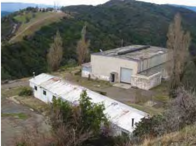
Building 112: electrical Power Station, looking southwest. (Page & Turnbull, February 2010)
