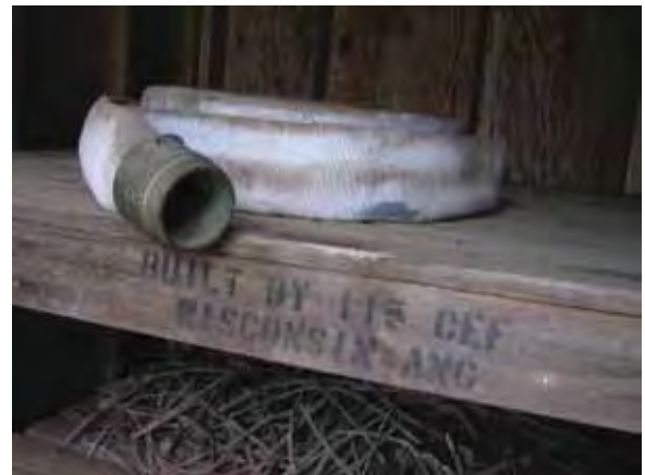
Building 234: Fire Hose House, detail of interior shelf (Page & Turnbull, February 2010)
