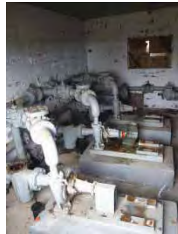
Building 118: Diesel Fuel Pump, interior. (Page & Turnbull, February 2010)
