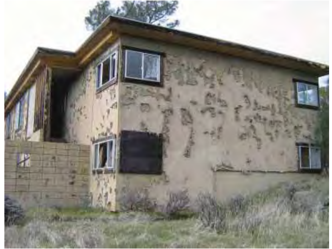
Building 513: Fourplex Apartment, looking west toward east façade. (Page & Turnbull, February 2010)
