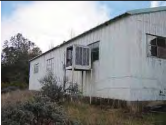
Building 213: Dispensary, south facade (Page & Turnbull, February 2010)
