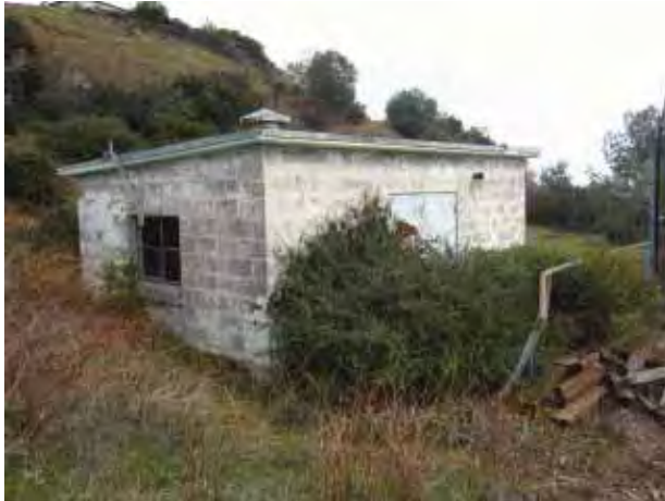
Building 118: Diesel Fuel Pump, looking southeast toward northwest and southwest (primary) façades. (Page & Turnbull, February 2010)
