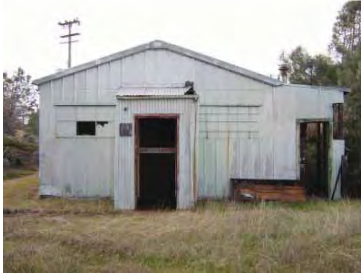
Building 212: NCO Open Mess, looking west toward east facade. (Page & Turnbull, February 2010)
