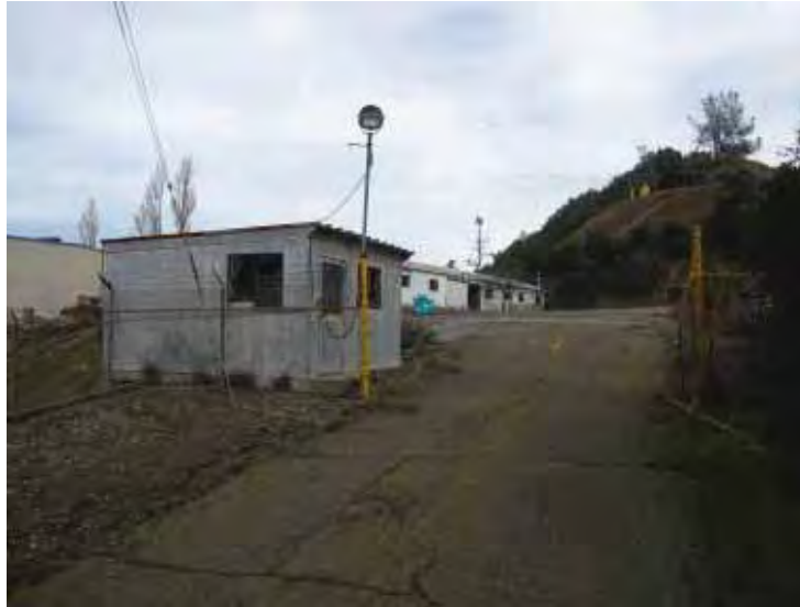
Building 115: Sentry House, looking northeast. (Page & Turnbull, February 2010)
