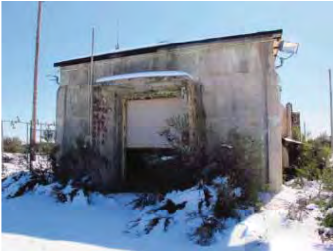
Building 700: Communications Transmitter/Receiver (GATR), northwest façade, looking southeast. (Page & Turnbull, February 2011)
