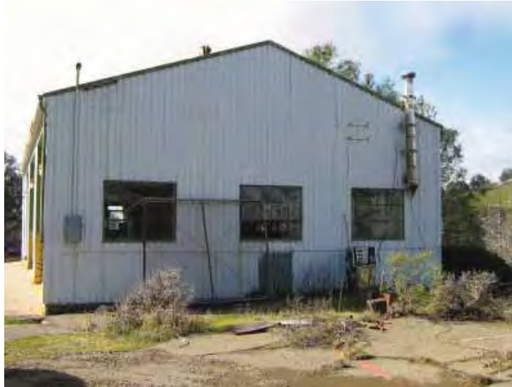
Building 211: Auto Maintenance Shop, looking west. (Page & Turnbull, February 2010)
