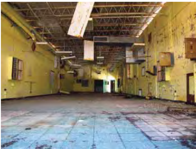
Building 700: Communications Transmitter/Receiver (GATR), interior, looking southeast. (Page & Turnbull, February 2011)
