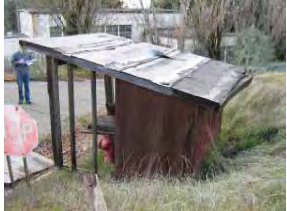
Building 215: Fire Hose House, east façade. (Page & Turnbull, February 2010)
