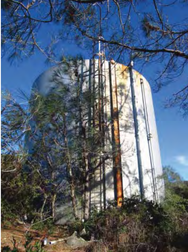
Building 884B: Water Tank, view north. (Page & Turnbull, February 2010)
