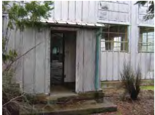
Building 225: Airman's Dining Hall, detail of primary entrance on south facade (Page & Turnbull, February 2010)
