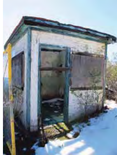
Building 715/722: Security Sentry House, north and east façades, looking southwest. (Page & Turnbull, February 2011)
