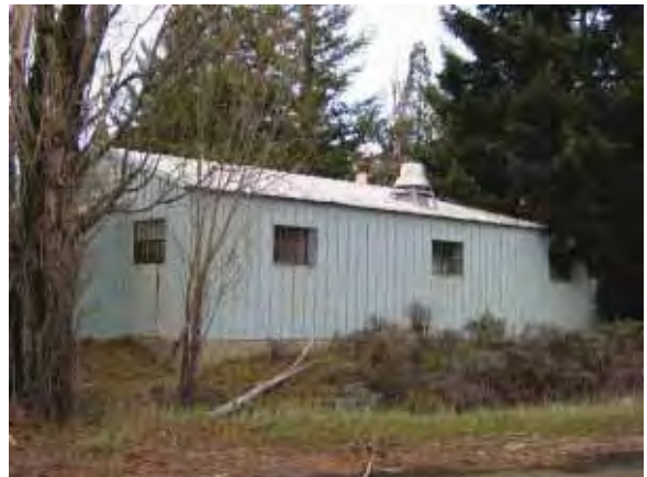
Building 230: Commissary, south facade (Page & Turnbull, February 2010)
