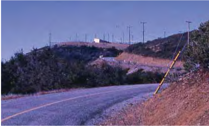
GATR (Building 700) with tall poles for lower-frequency antennae and shorter FRT-49 horizontal array visible, ca. 1964-1965. (Source: N. McKiethan via B. Jaber Archives)
