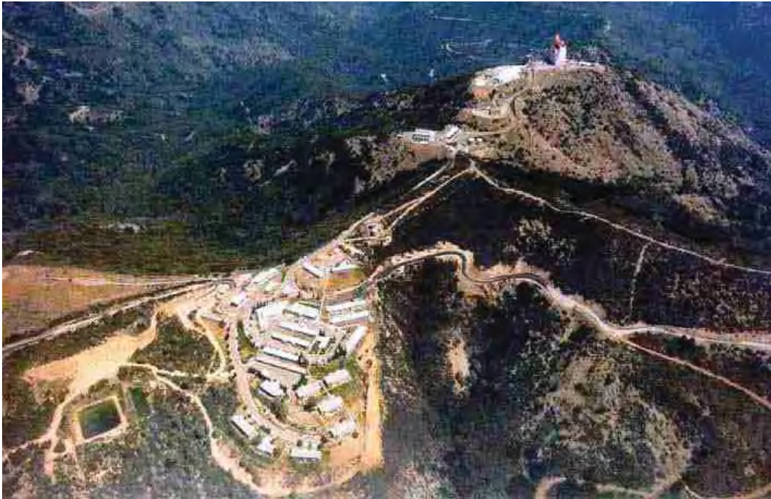
Aerial, Almaden Air Force Station, ca. 1960s. Cantonment in the western foreground and radars to the east (several steel barracks buildings were removed in the 1970s). (Source: http://www.radomes.org/museum/ )
