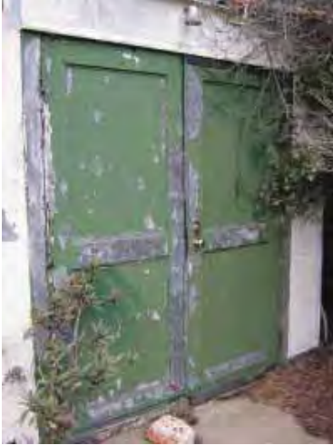
Building 200: Water Pump Station, view of entrance. (Page & Turnbull, February 2010)
