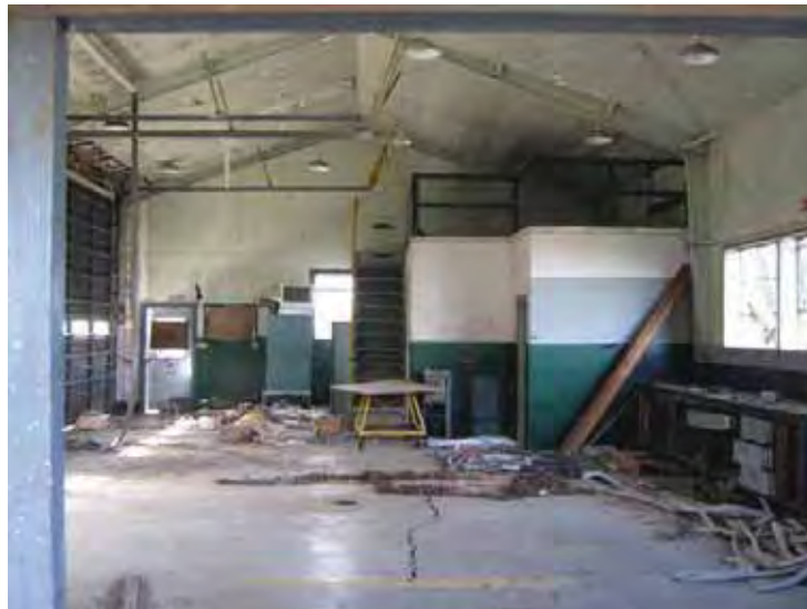
Building 211: Auto Maintenance Shop interior, looking west. (Page & Turnbull, February 2010)
