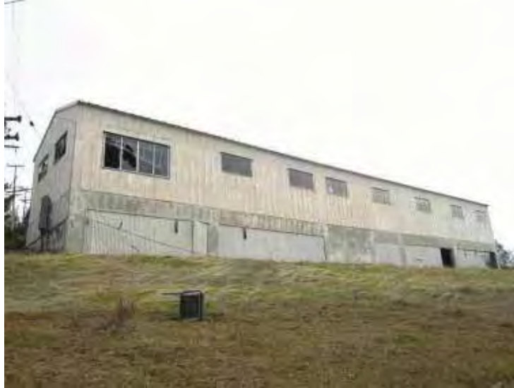
Building 207: Squadron Headquarters/Orderly Room, west facade. (Page & Turnbull, February 2010)
