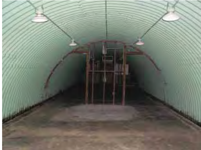
Building 105: Fallout Shelter, interview view. (Source: MROSD, 2011)
