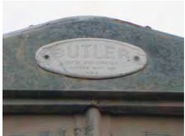
Building 250: Auto Maintenance Storage, detail of Butler Mfg. Company badge (Page & Turnbull, February 2010)
