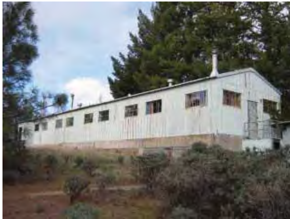
Building 233: Barracks, south and west facades (Page & Turnbull, February 2010)
