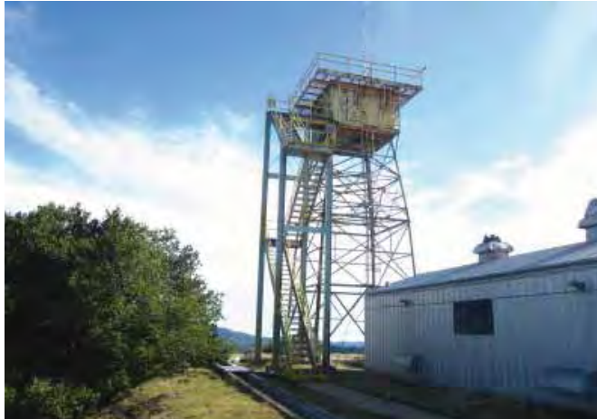
Building 108: Radar Tower MPS-14, looking southwest. Building 110: Training is at right. (Page & Turnbull, February 2010)
