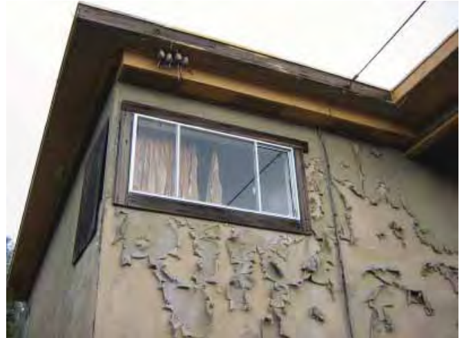
Building 510: Fourplex Apartment, looking southwest toward primary façade. (Page & Turnbull, February 2010)
