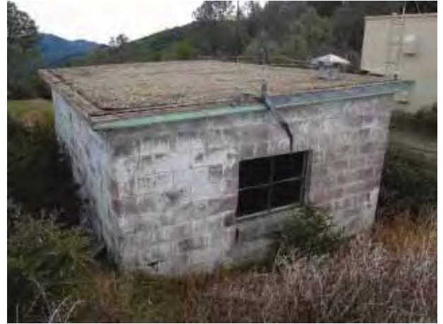
Building 118: Diesel Fuel Pump, looking southwest toward northwest façade. (Page & Turnbull, February 2010)
