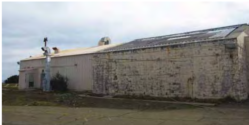
Building 100, looking southeast toward the north façade of the building prior to abatement. (Page & Turnbull, February 2010).
