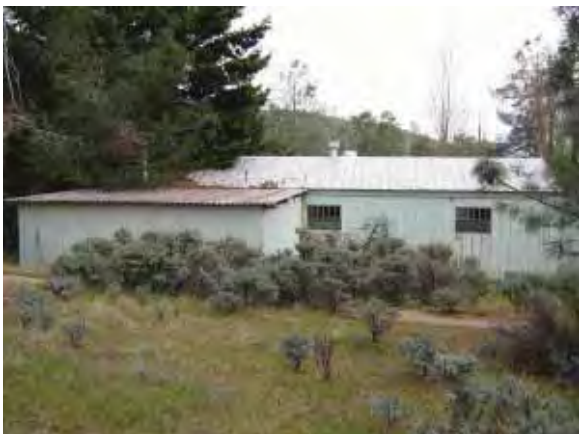
Building 230: Commissary, north facade with addition (Page & Turnbull, February 2010)
