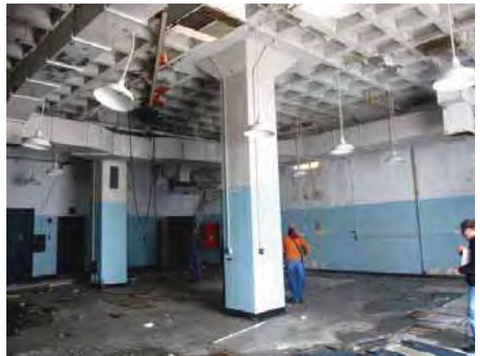
Fourth floor interior prior to abatement. (Page & Turnbull, February 2010)
