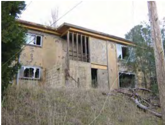
Building 511: Fourplex Apartment, looking north toward rear façade. (Page & Turnbull, February 2010)
