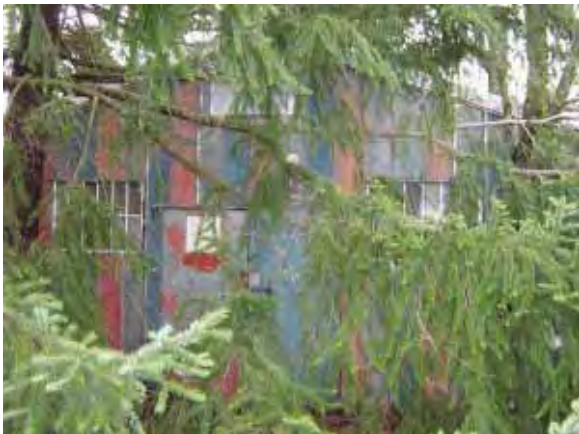
Building 230: Commissary, detail of primary entrance (Page & Turnbull, February 2010)
