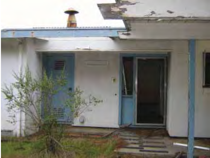
Building 516: Commander's House, looking west toward the primary entrance. (Page & Turnbull, February 2010)
