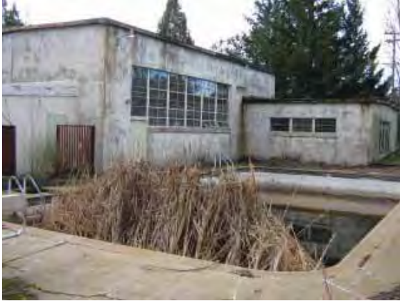
Building 275: Swimming Pool, view to the east with Building 245: Recreation adjacent. (Page & Turnbull, February 2010)
