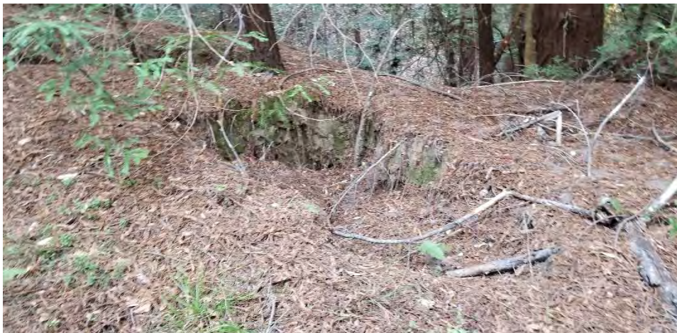
Photo 6: Sinkhole due to subsurface soil piping
