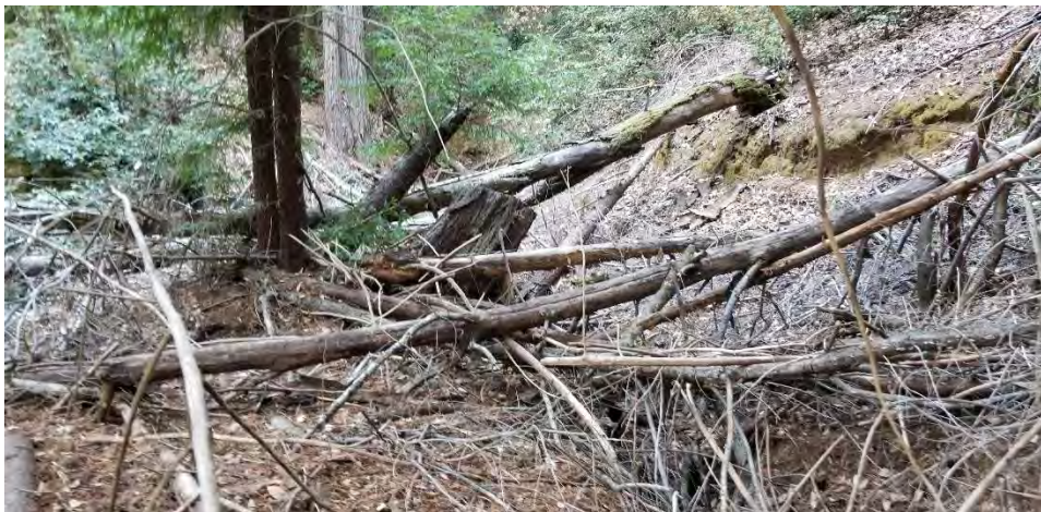
Photo 8: Looking upstream and slide debris deposited in the crossing. The stream is located right of center in the photo.
