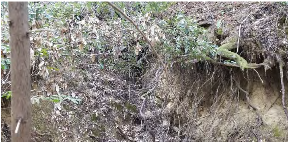
Photo 5: Gully in steep cutbank from diverted stream flow originating from MP 1 and MP2
