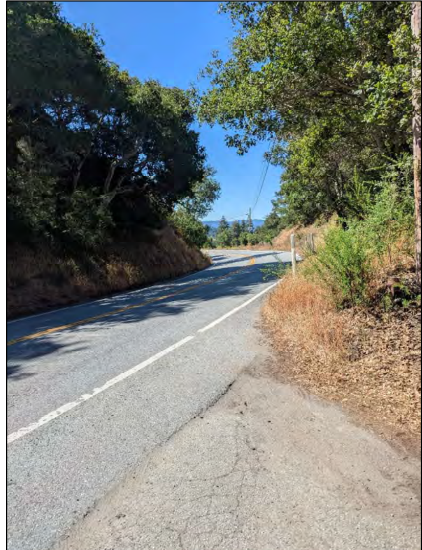
Figure 3 (continued) Looking Right from Site E3 North Driveway
