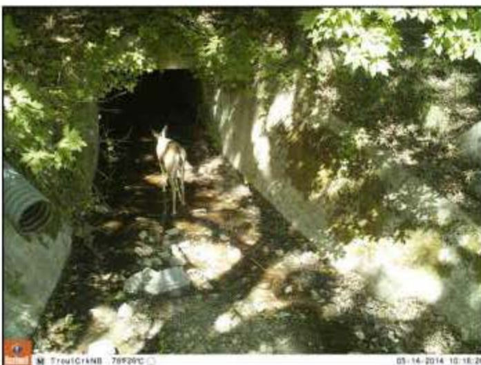
Deer investigating Trout Creek Culvert
