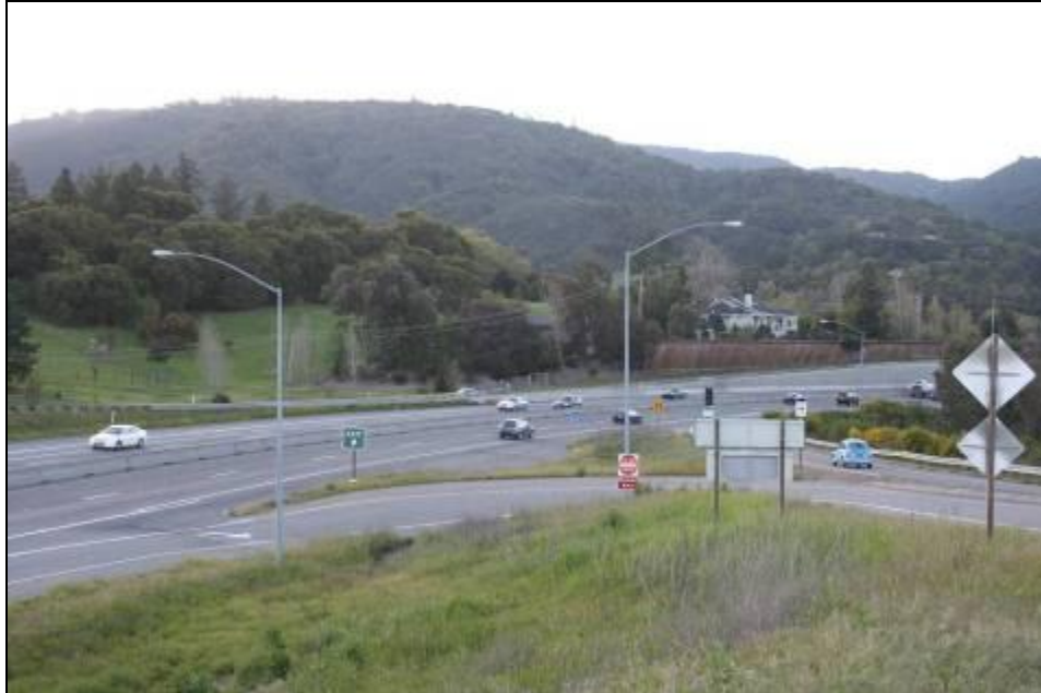
Figure A1: Concrete median in Highway 17, north view.
