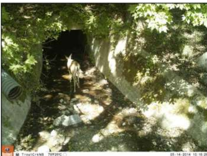
Deer investigating Trout Creek Culvert
