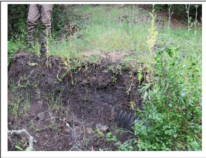
Photo 3. Culverted stream crossing, before restoration
