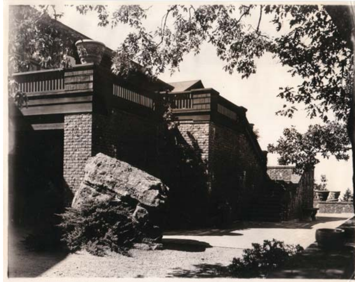
Figure 32: East Façade of the Main House after 1920. Again, note the location of the rock. (Western Archives of the Society of Jesus).
