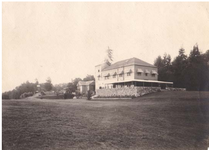
Figure 4: Tevis Alterations to Flood House, 1906-1909 (Western Archives of the Society of Jesus).
