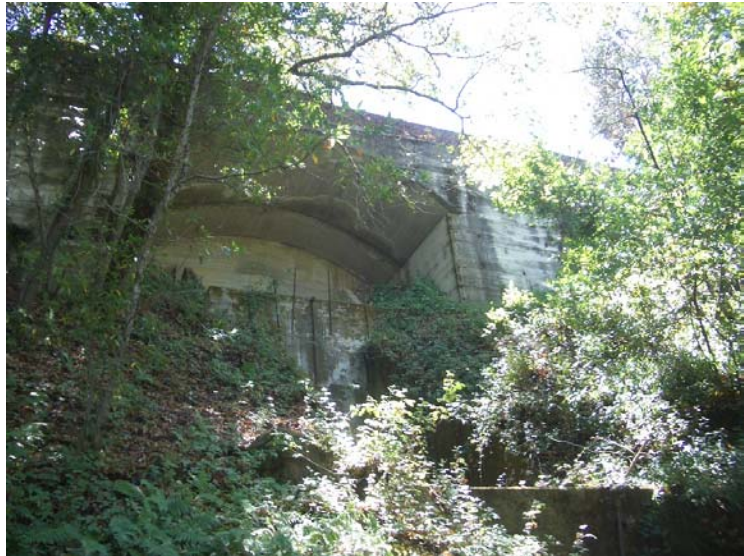
Figure 38: Retaining Wall and Water System at North Side of Complex, 2005 (Page & Turnbull).
