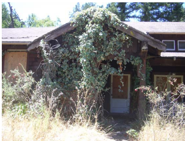
Figure 29: North Facade, Classroom Building, 2005 (Page & Turnbull).
