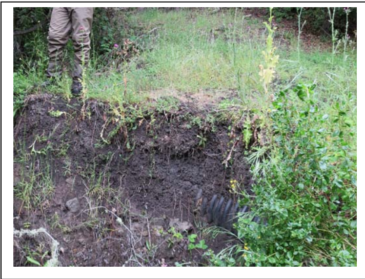
Photo 3. Culverted stream crossing, before restoration
