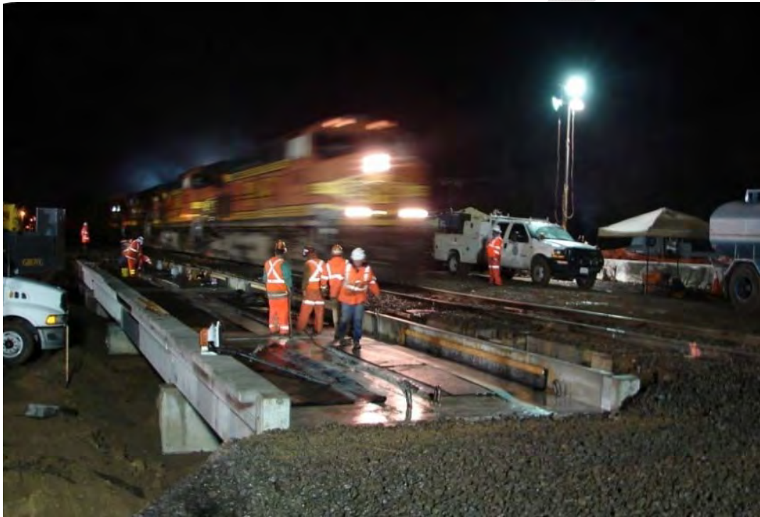
BNSF / G Street Underpass Night Construction (Client: City of Merced)
