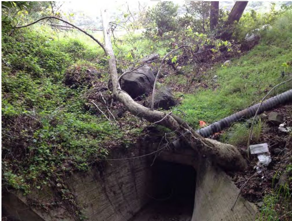
Ravine Culvert Inlet
