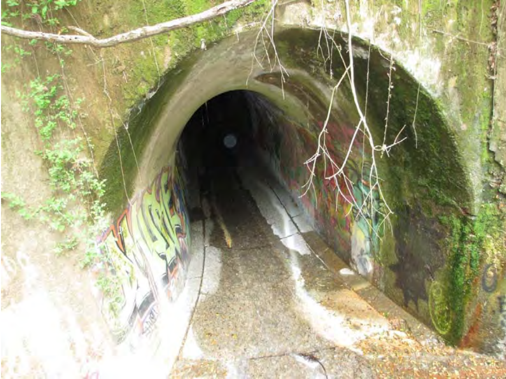
Briggs Creek culvert inlet
