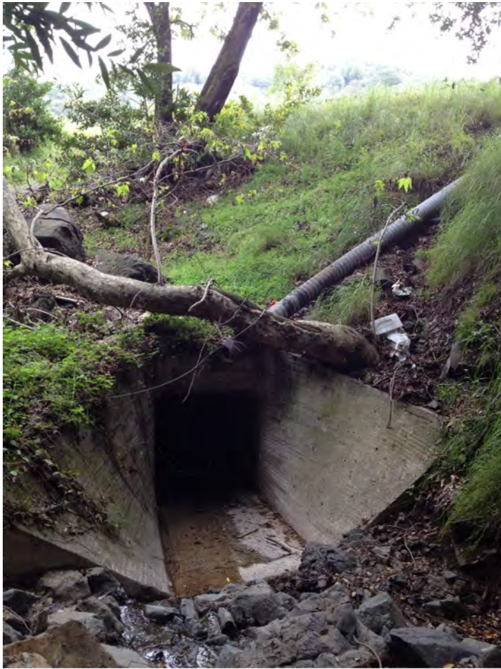
Ravine Culvert inlet (Ravine Culvert outlet could not be found)
