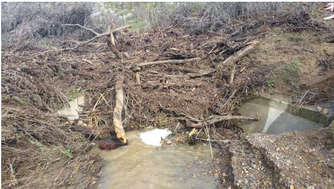
Black Creek Culvert Inlet, March 7, 2016
