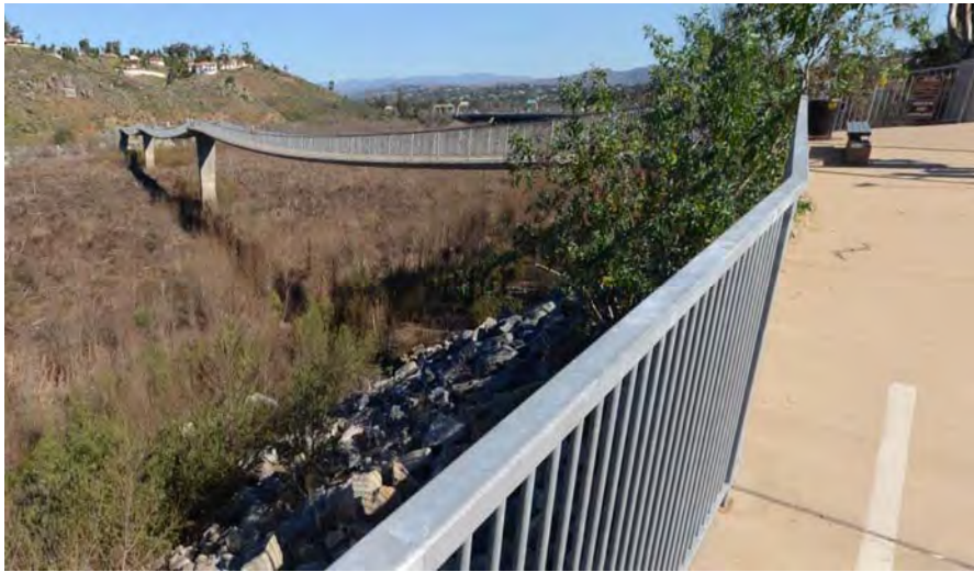
Trail suspension bridge in San Diego County (photo J. Falkowski)
