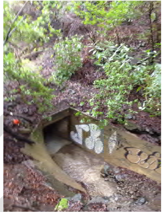
Existing culvert inlet on west side
