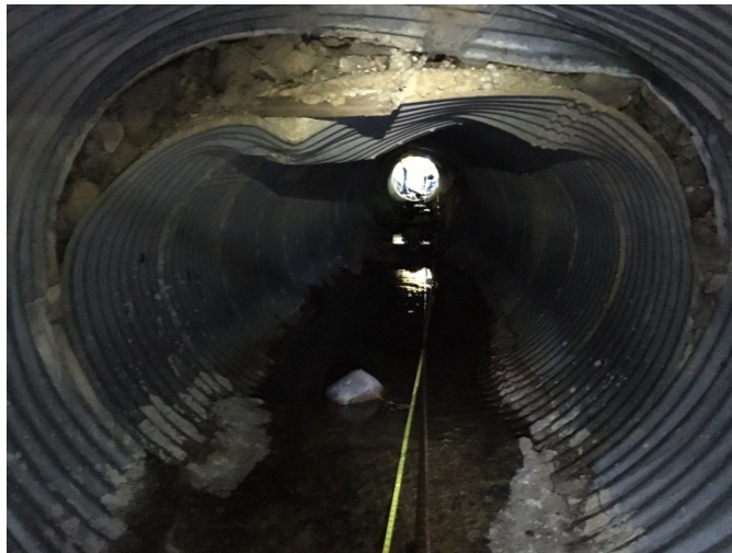
Figure 7. Pipe joint separation at 66 feet from the culvert inlet (looking towards culvert inlet)
