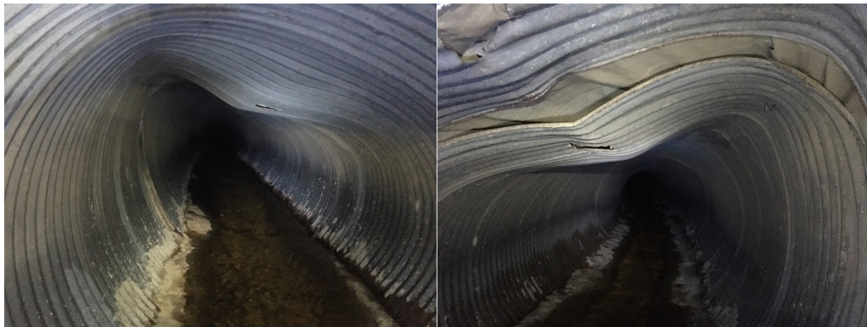
Figure 9. Left: Distorted CMP pipe 422 feet from inlet along BCR (looking towards inlet). Right: The 9-inch gap (looking towards outlet along Alma College Road).
