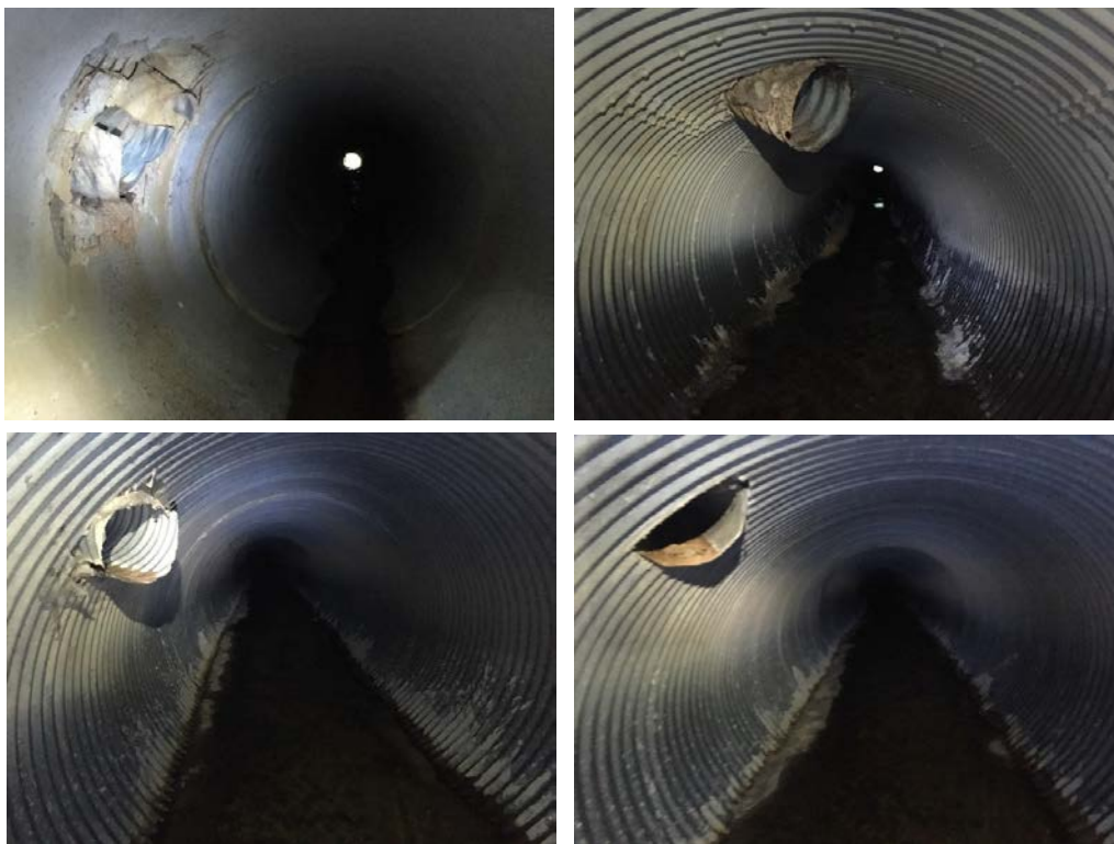
Figure 10. Four piped inlets. Starting top left: Clockwise: 24-inch, 12-inch, 12-inch, 8.5-inch
