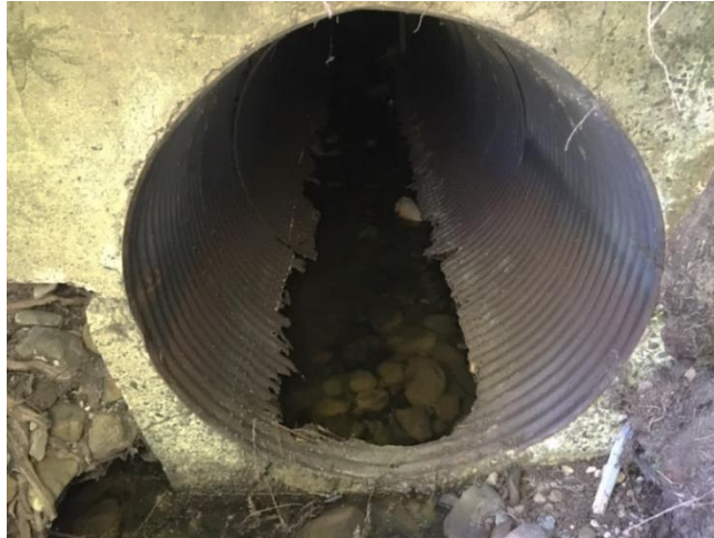
Figure 4. Damaged culvert inlet on the southwestern side of BCR at Webb Creek
