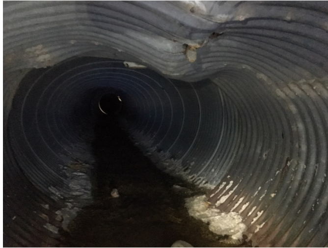
Figure 6. Roof collapse at 62 feet from entrance at Webb Creek (looking towards culvert outlet)
