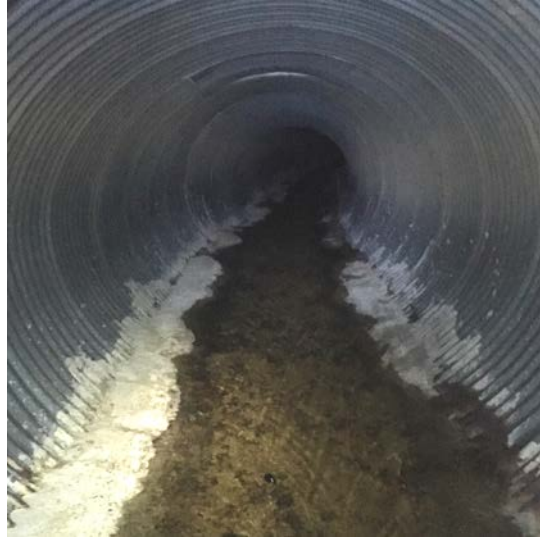
Figure 8. Typical section of concrete slurry lined CMP
