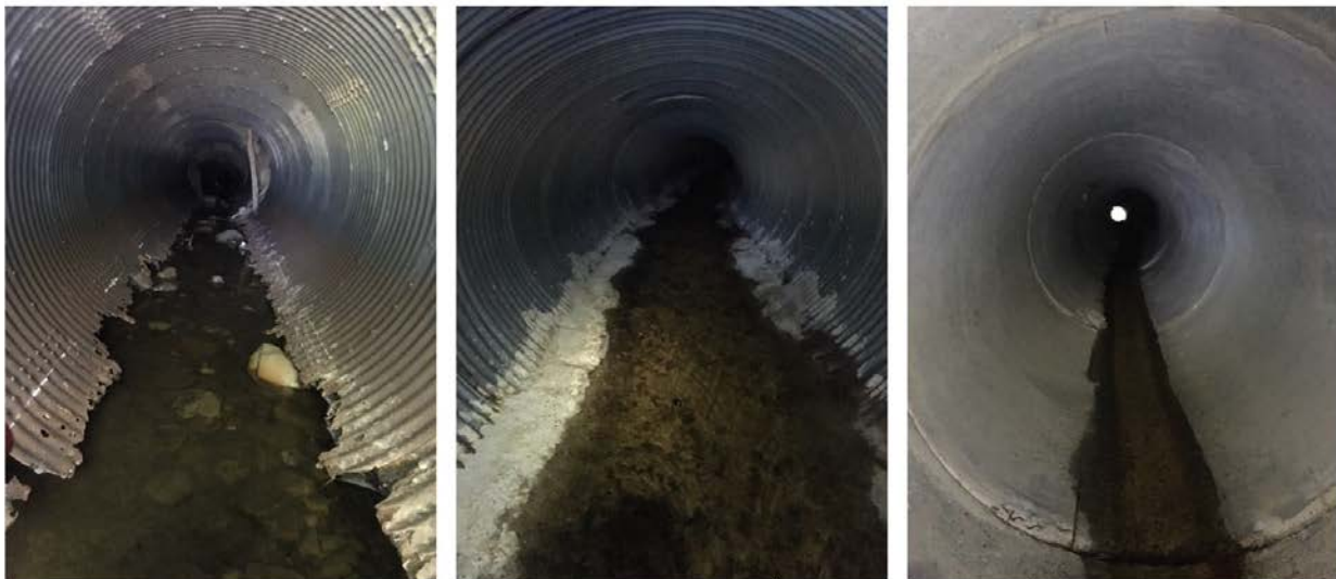
Figure 2. Pipe culvert materials. Left to right: highly corroded CMP, concrete lined CMP, and concrete
