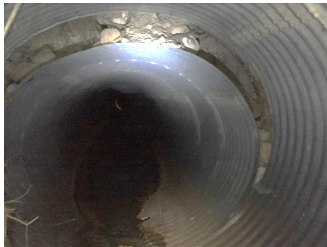
Figure 5. Separation at CMP pipe joint (looking into culvert from Webb Creek Inlet)
