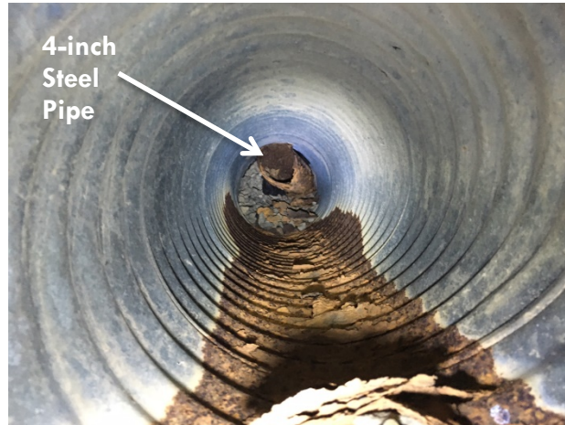
Figure 11. 12-inch piped inlet with steel pipe in center.
