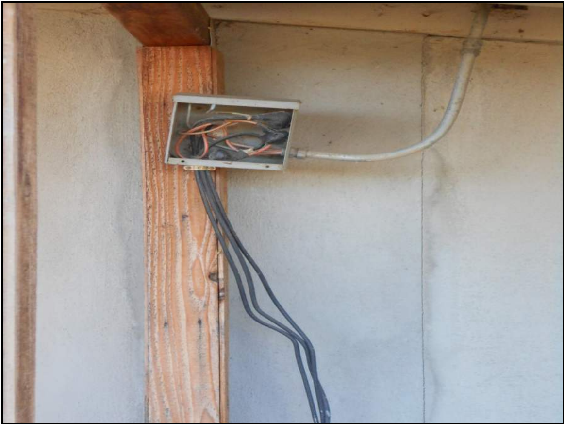
Photo 19 - Exposed Electrical Wiring
