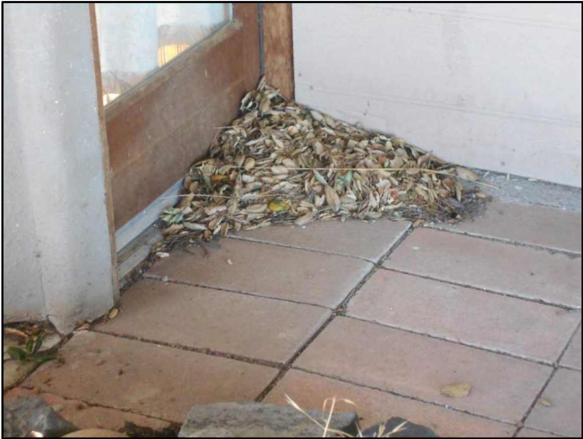
Photo 21 - Patio Pavers Slope into Family Room Door
