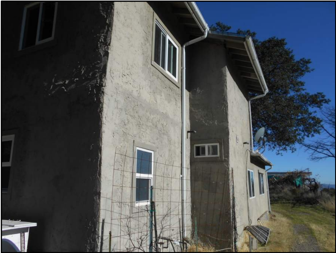
Photo 13 - South Exterior, Non-Plumb Wall
