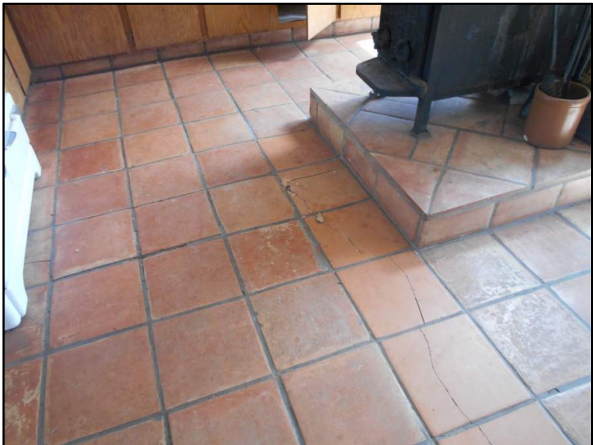
Photo 16 - Cracks in Kitchen Floor
