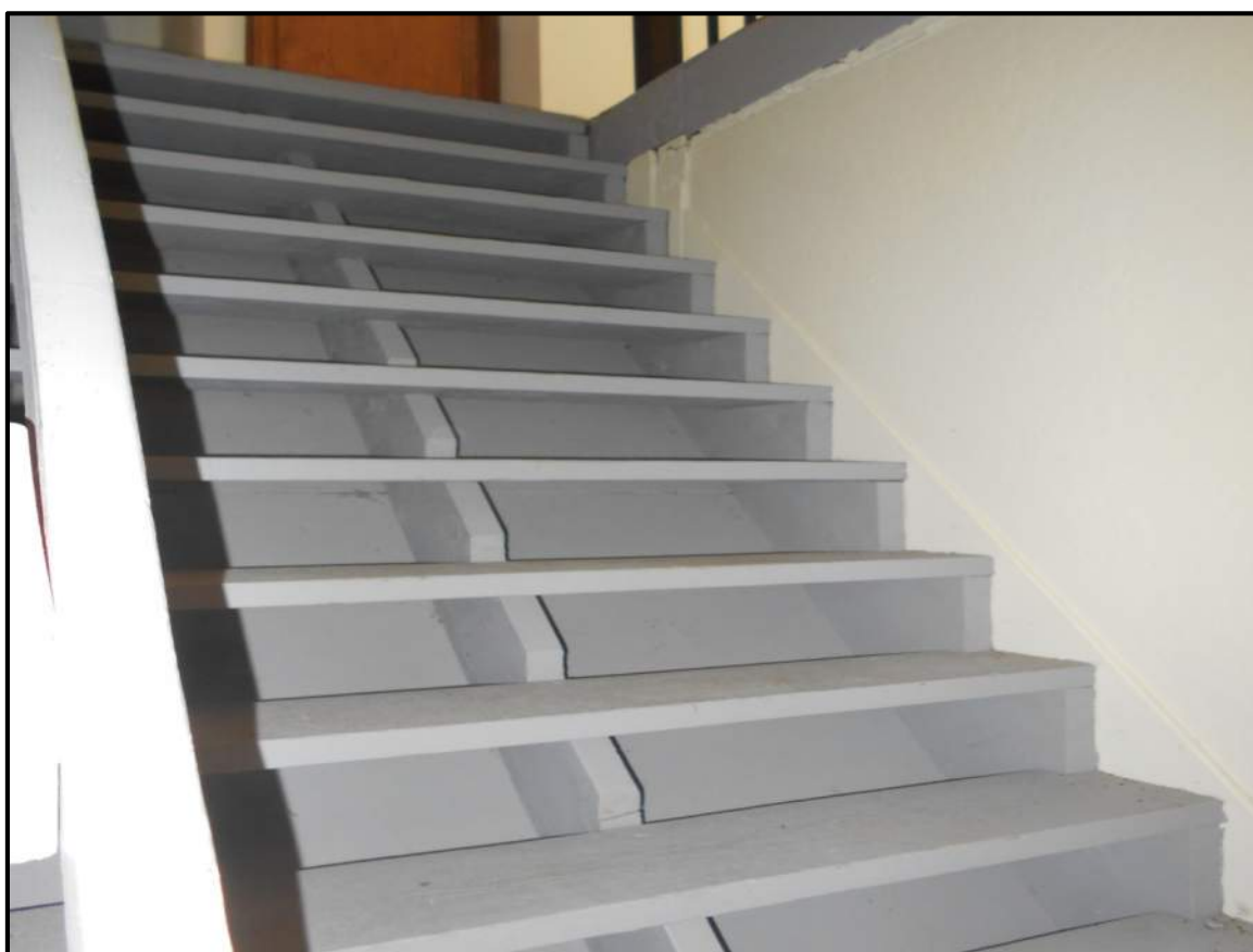
Photo 18 - Ship's Ladder, Not Acceptable Fire Exit
