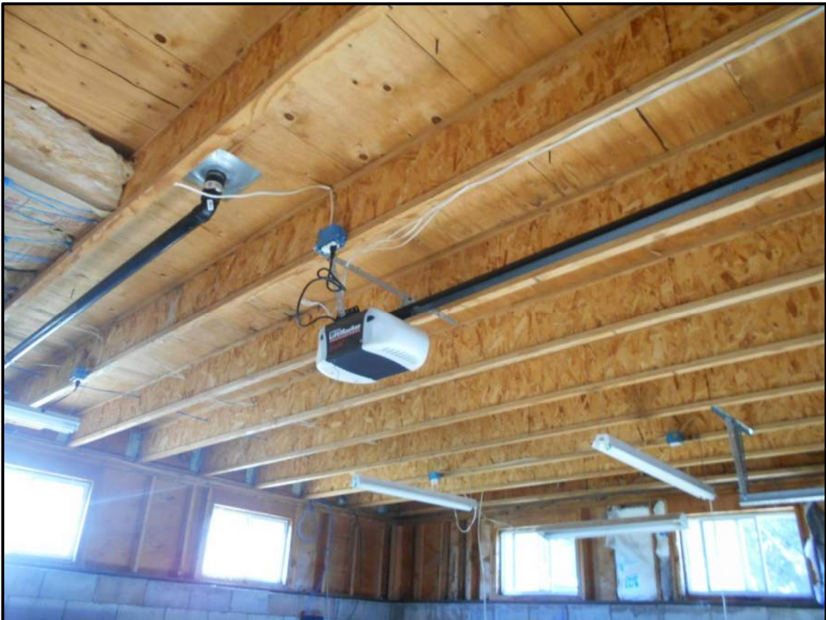
Photo 36 - Plywood and TJI Roof Rafters
