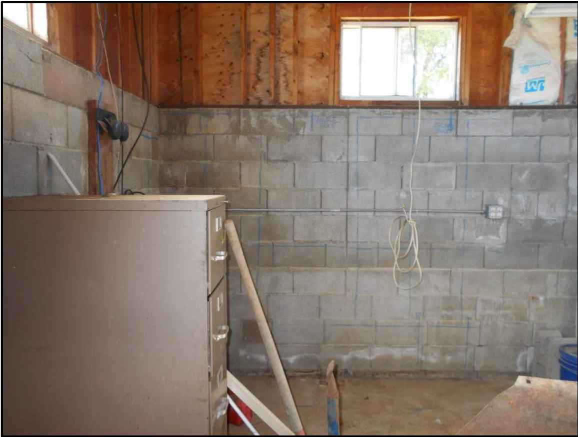
Photo 37 - CMU Retaining Wall and Wood Framed Pony Wall
