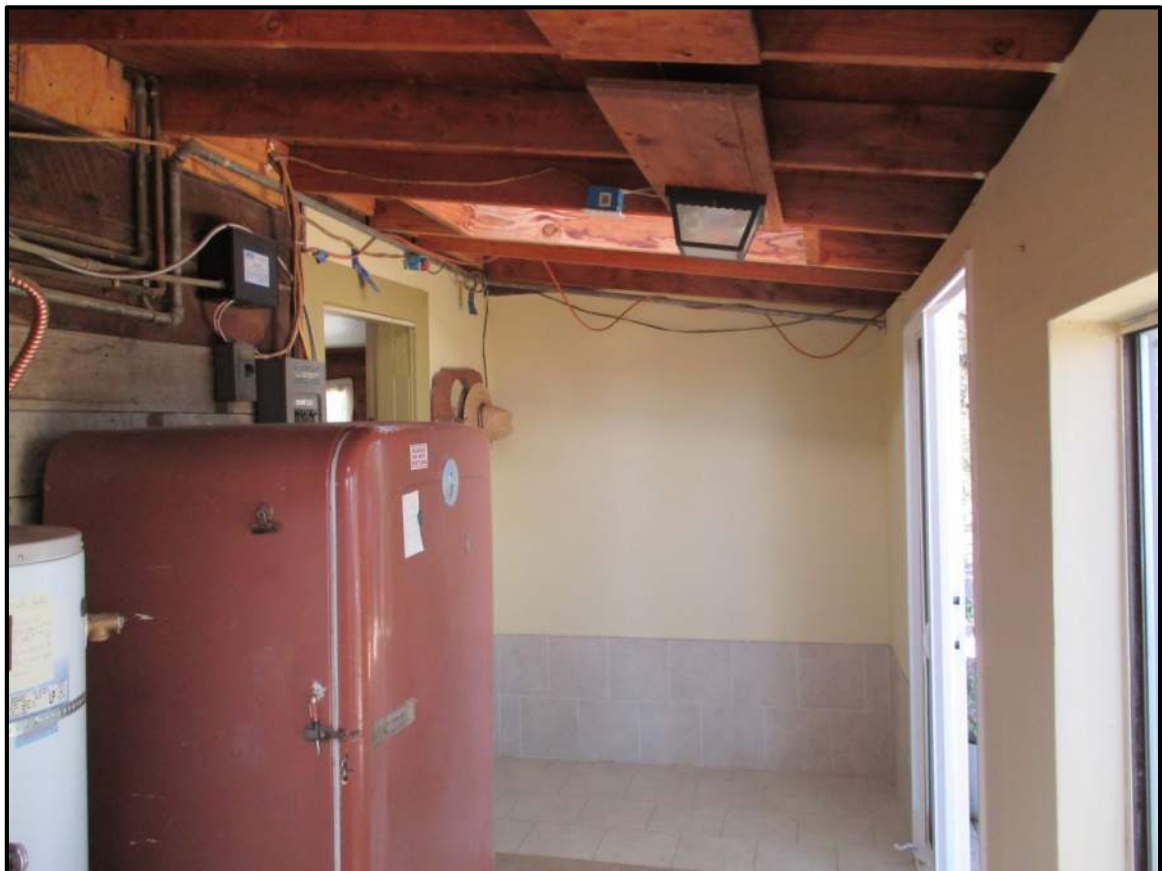
Photo 20 - Exposed Electrical Wiring
