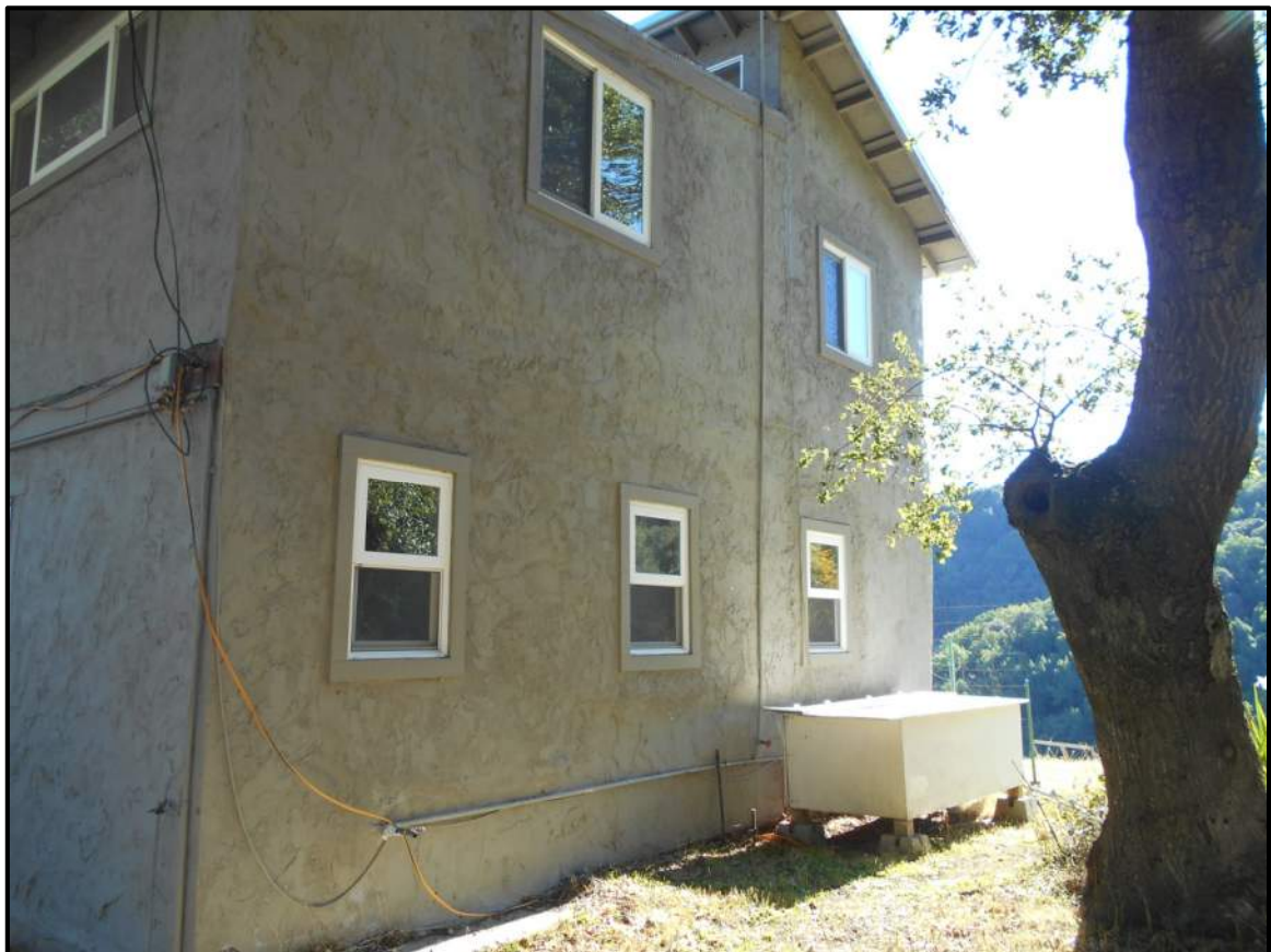
Photo 12 - West Exterior, Non-Plumb Wall
