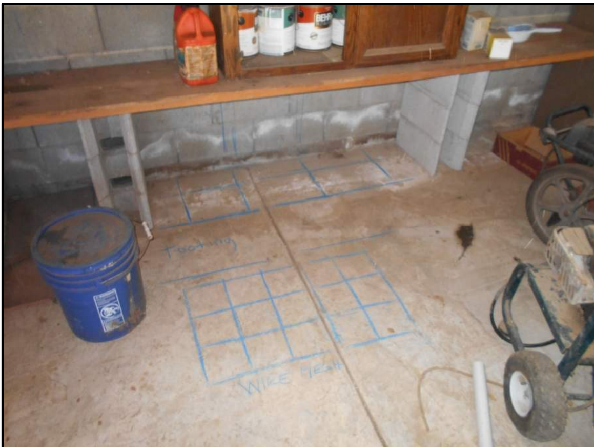
Photo 38 - CMU Retaining Wall Footing and 5" Thick Slab-on-Grade
