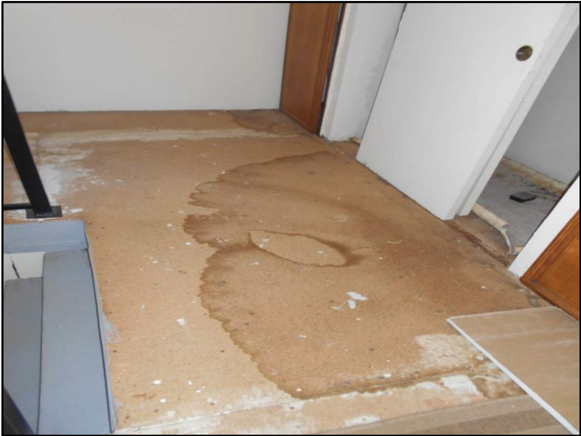
Photo 11 - Water Damage at 2nd Floor
