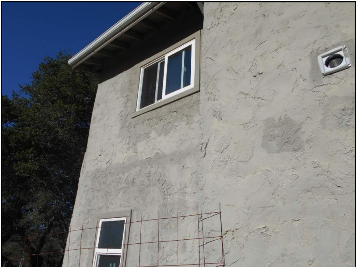
Photo 14 - South Exterior, Non-Plumb Wall
