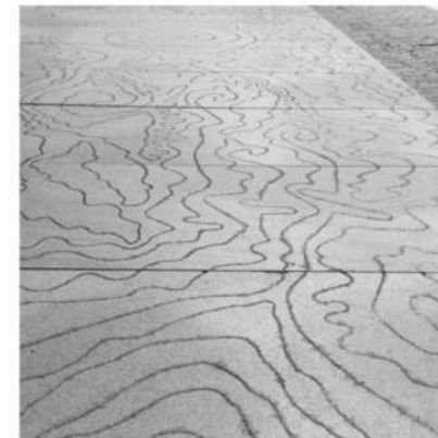
Concrete paving with etched contour pattern
