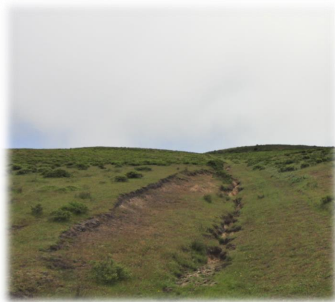
Figure-8: Gully/rutting activity along an insloped road just south of the Agricultural Lease. Large gully caused by surface water flow during winter storm events. Road should be re-graded and water diversion points installed to relieve surface flow to protect the integrity of the road.
