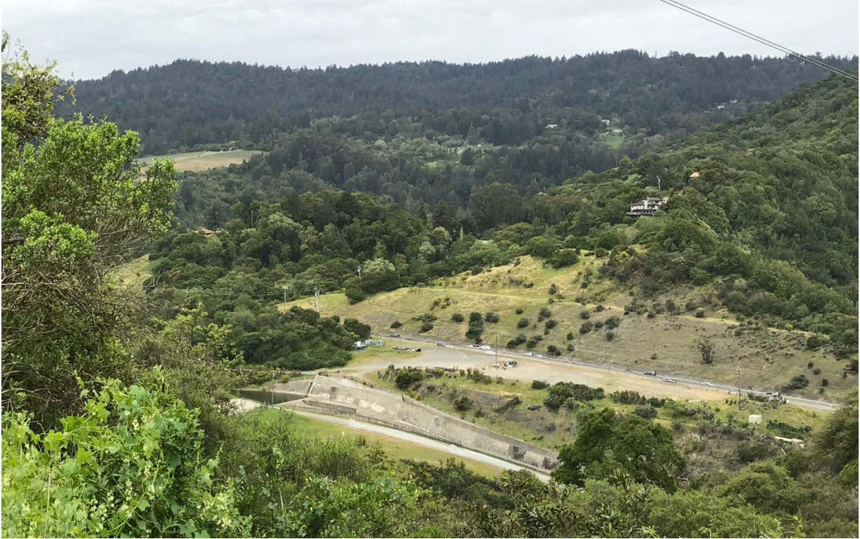
Photo 6. Taken from Jones Trail in St. Joseph’s Hill OSP, looking west. View of the Lenihan Dam spillway and service road at Lexington Reservoir and Highway 17 in the vicinity of Southern Overcrossing (3).
