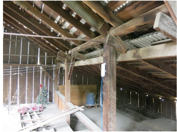
Figure 15. Horizontal steel tie rod attached to the top of the wood post.
