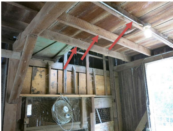
Figure 20. Wood attic joists (arrows) in the center section supported by a wood beam and the exterior wall.
