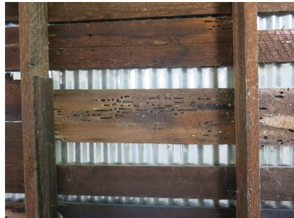
Figure 37. Damage to the skip sheathing from wood-boring insects.
