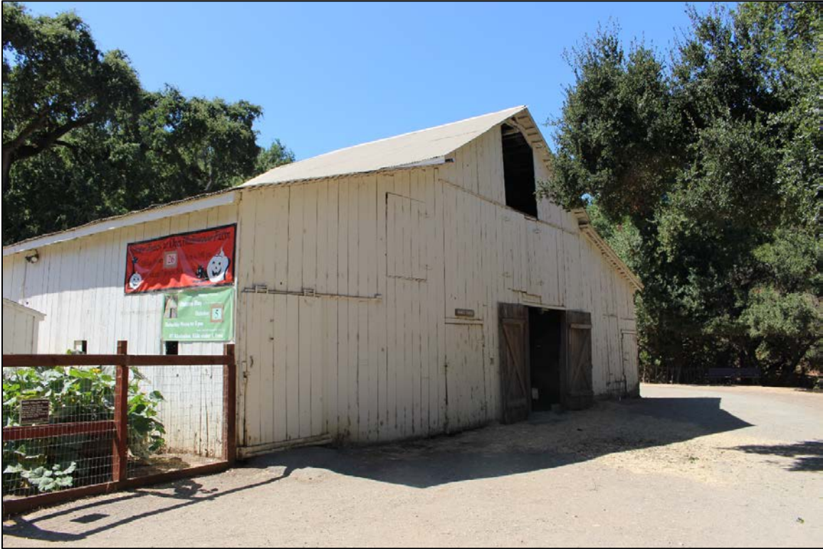
Photo 1. White Barn front facade, view west.
