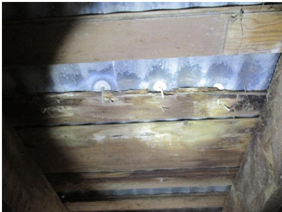
Figure 36. Deteriorated skip sheathing.
