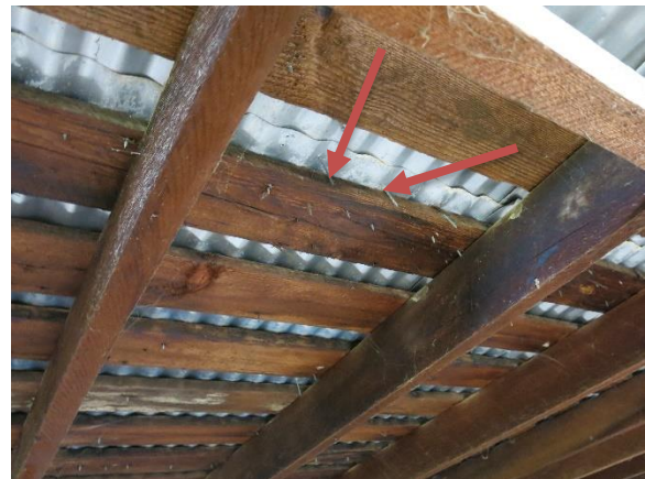
Figure 13. Fasteners not attached to the wood skip sheathing (arrows).
