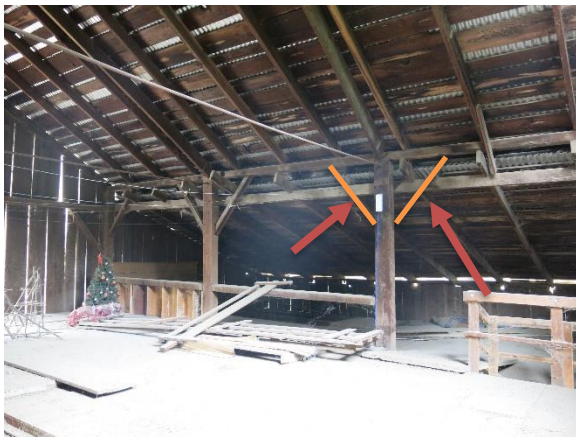
Figure 39. Locations where diagonal knee braces are missing (arrows)
