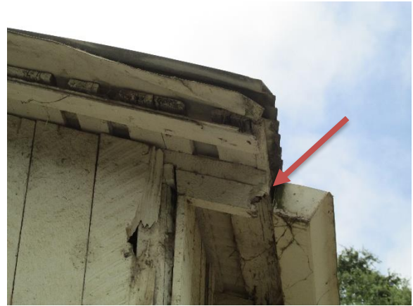
Figure 31. Deteriorated rafter tail on west side.
