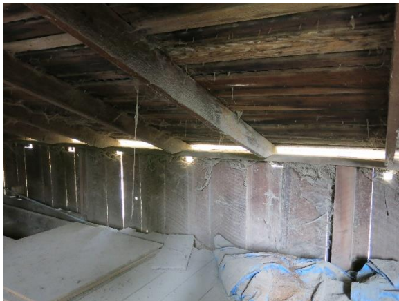
Figure 16. Roof rafters for the west side supported on the exterior wall.
