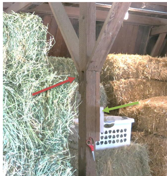
Figure 44. Column mortise (Red arrow) and wood reinforcing plate (green arrow)
