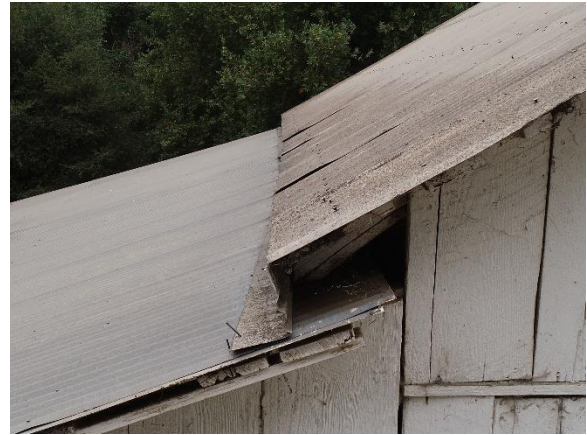
Figure 29. Protruding fasteners at roof transition.
