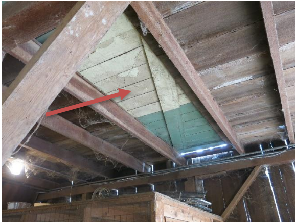
Figure 22. Attic floor opening covered with wood boards (arrow).
