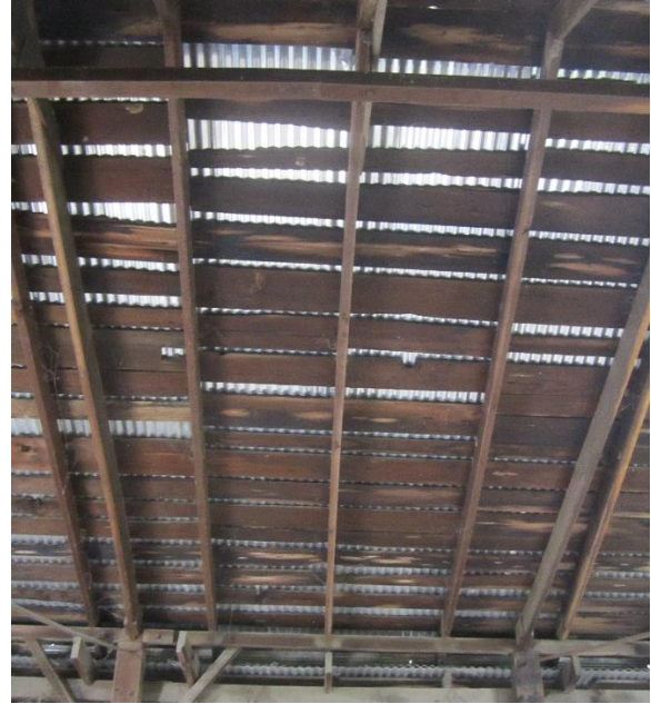
Figure 11. View of wood skip sheathing showing the various sizes and spacing typical at the center gable.
