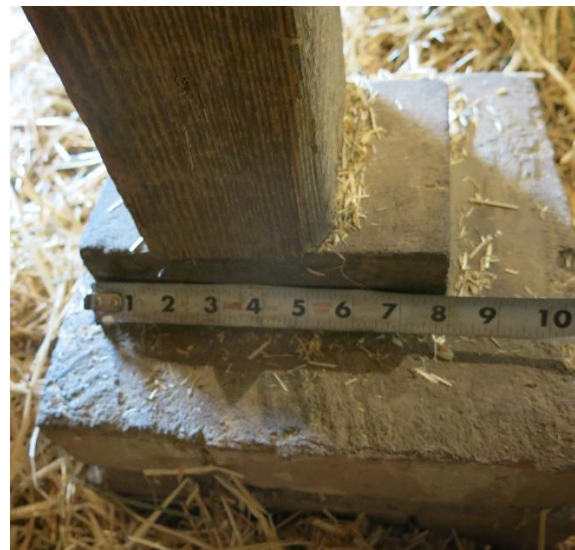
Figure 46. Wood shim between the column and the brick footing.
