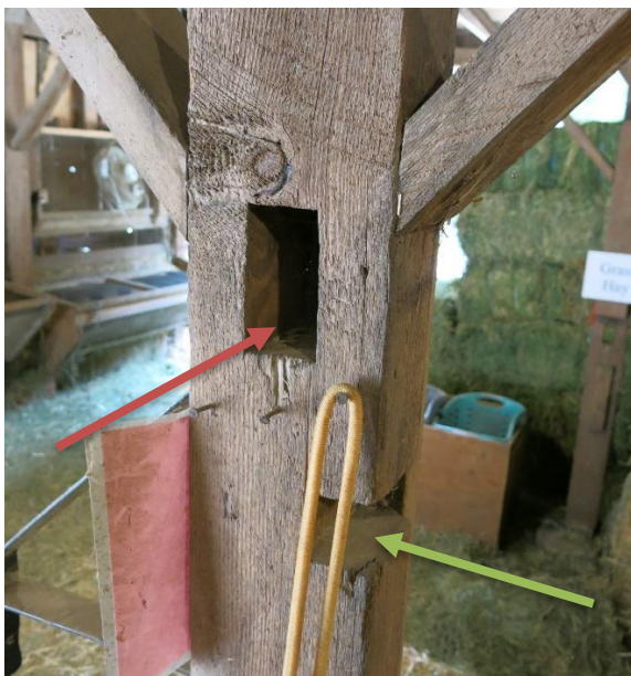
Figure 43. Mortising of wood column (red arrow) and notch in column (green arrow).
