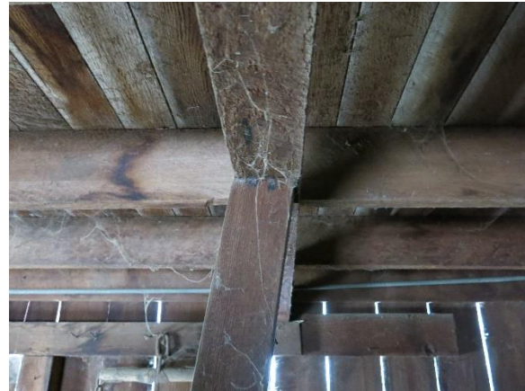
Figure 48. Sloped wood column supporting attic beam.
