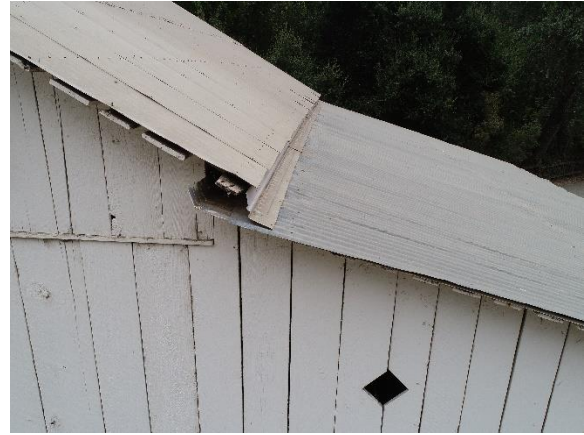
Figure 7. Break in roof plane where transitions from gable to shed roof.
