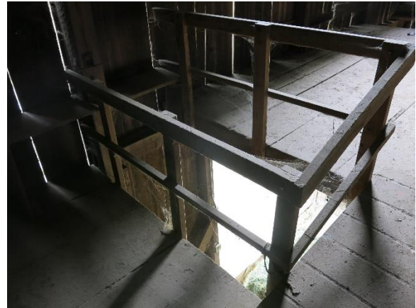
Figure 23. Attic floor opening surrounded by wood guardrail.
