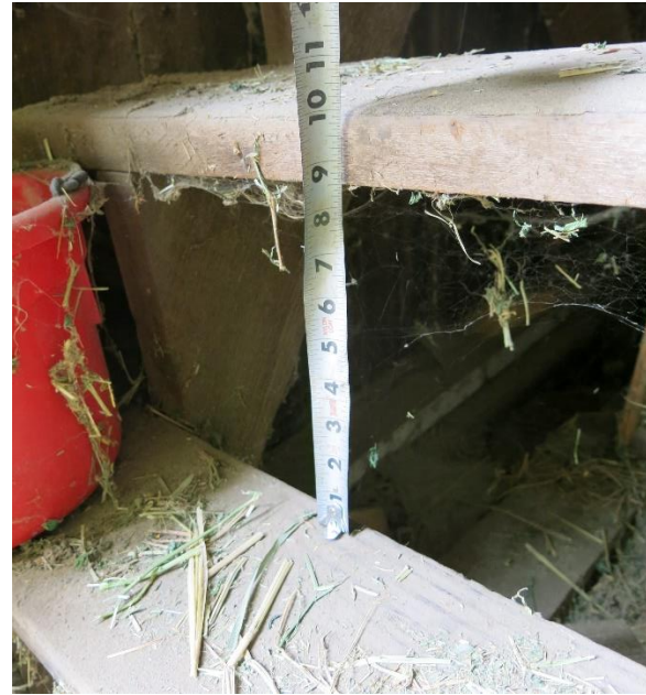
Figure 52. Vertical rise of attic stair.
