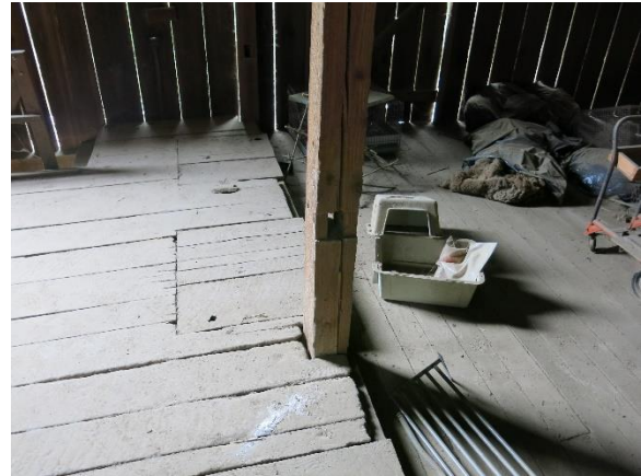
Figure 5. Attic over the east side to the right and over the center section to the left.
