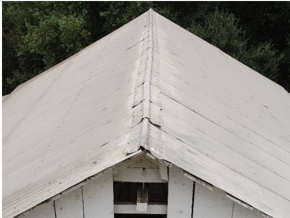
Figure 30. Distressed ridge flashing.
