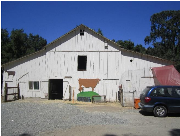
Figure 2. South elevation of the barn.
