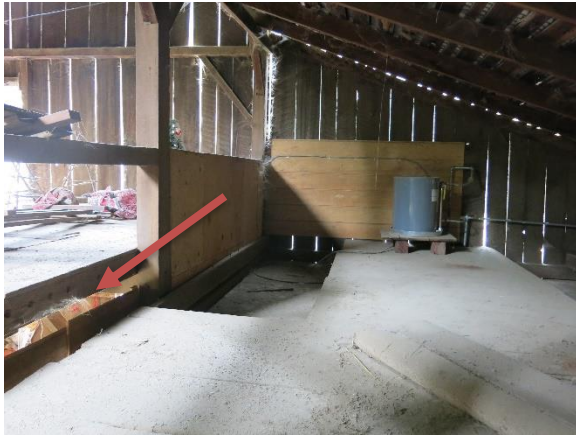
Figure 4. Attic above the west side. Arrow shows the vertical offset at the attic over the center section.
