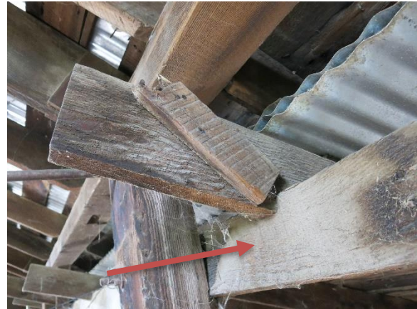
Figure 19. Wood beam (arrow) supporting east side shed roof rafters.
