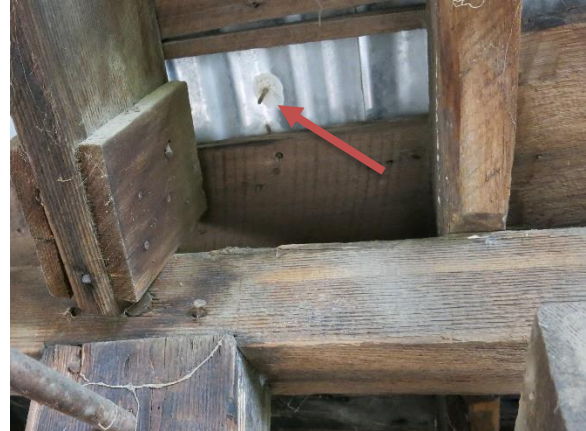
Figure 35. Corrosion at fastener that did not penetrate skip sheathing.
