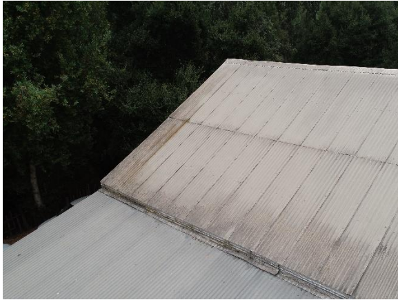
Figure 28. Corrosion, biological growth, and soiling on roofing panels on the west side.
