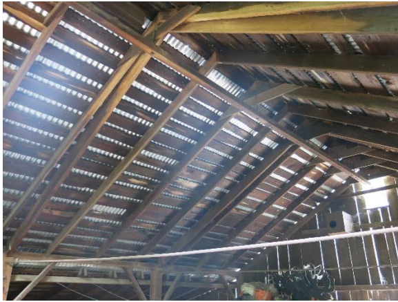
Figure 14. Wood rafters supporting the center section of roof with wood skip sheathing and corrugated metal deck.
