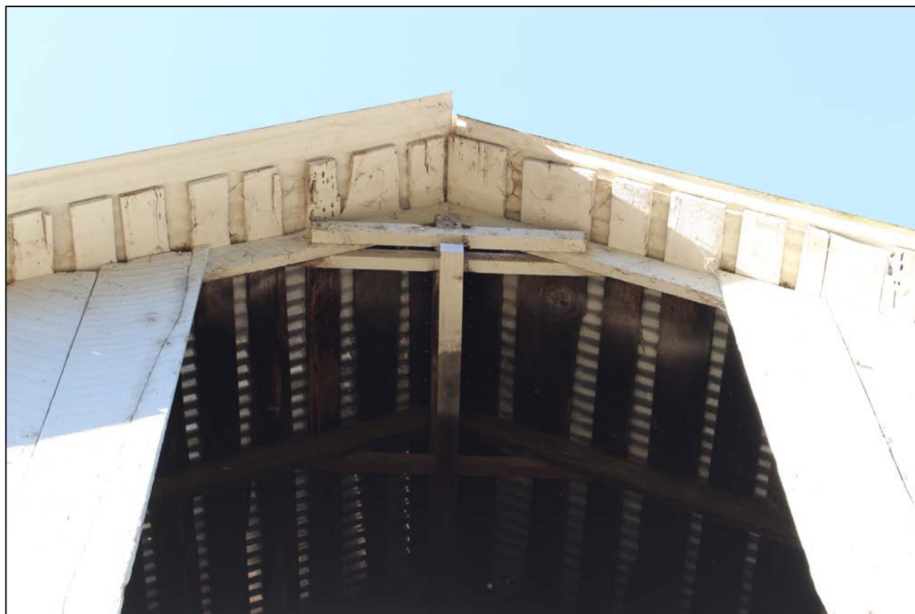
Photo 5. Detail of main gable exposed eaves, view south.
