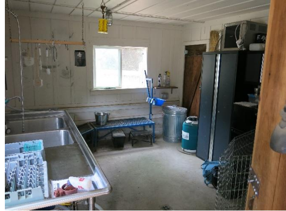
Figure 27. Concrete floor slab in the milk room.
