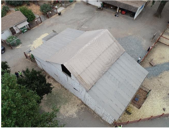
Figure 6. Aerial view of corrugated, galvanized sheet metal roofing panels.
