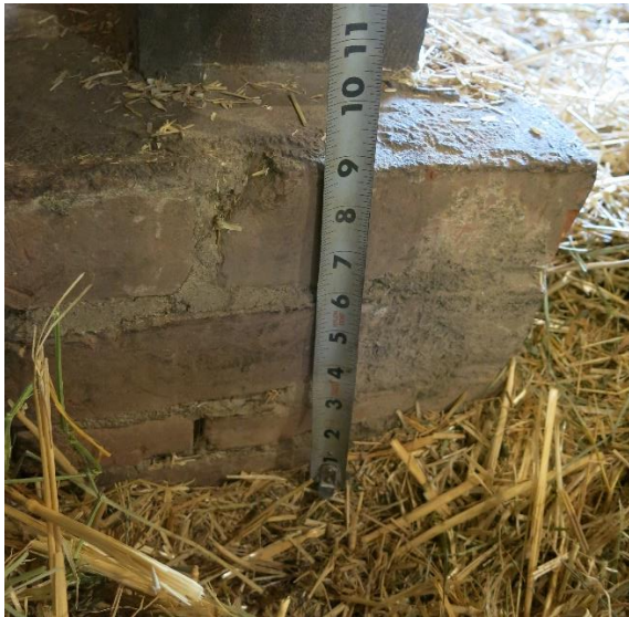
Figure 45. Brick footing extending above the adjacent ground.
