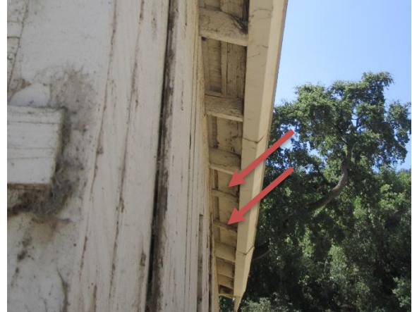
Figure 9. Two rafter tails have been cut and are half the depth of other rafter tails.
