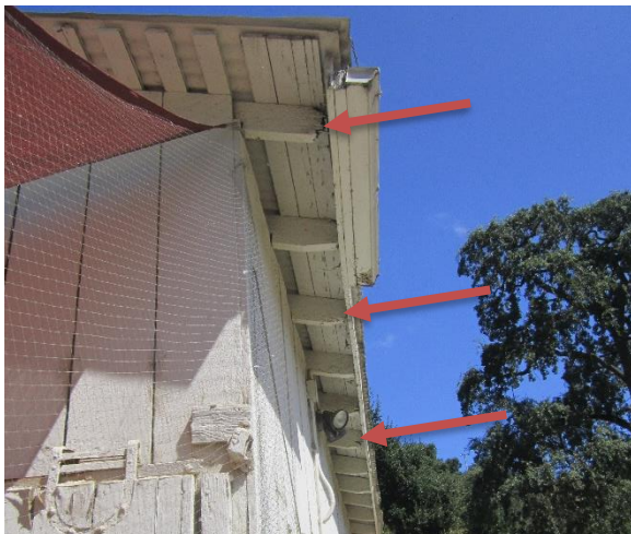
Figure 32. Deteriorated rafter tails on east side.
