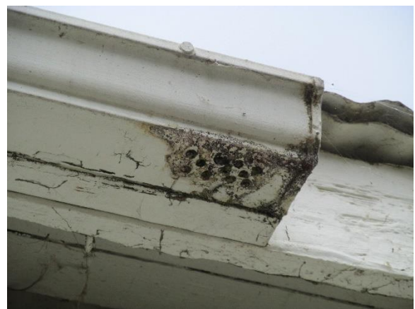
Figure 33. Soiling and corrosion at the underside of the gutter on the east side.
