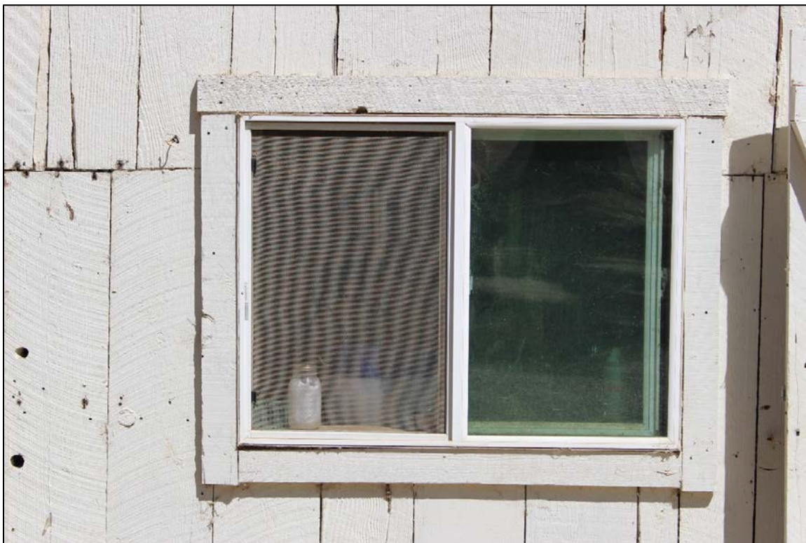
Photo 9. Detail of vinyl window installed during milk room renovation, view southeast.
