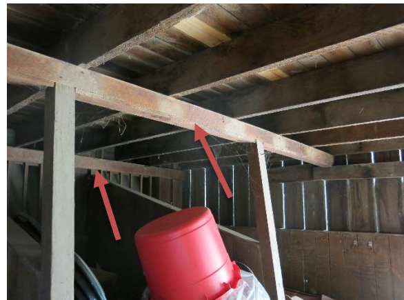
Figure 21. Wood attic rafters in the east section supported on north-south wood beams (arrows).
