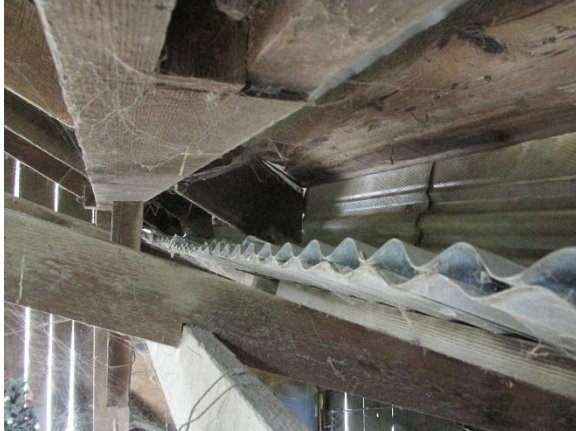
Figure 34. “L” flashing from the interior.
