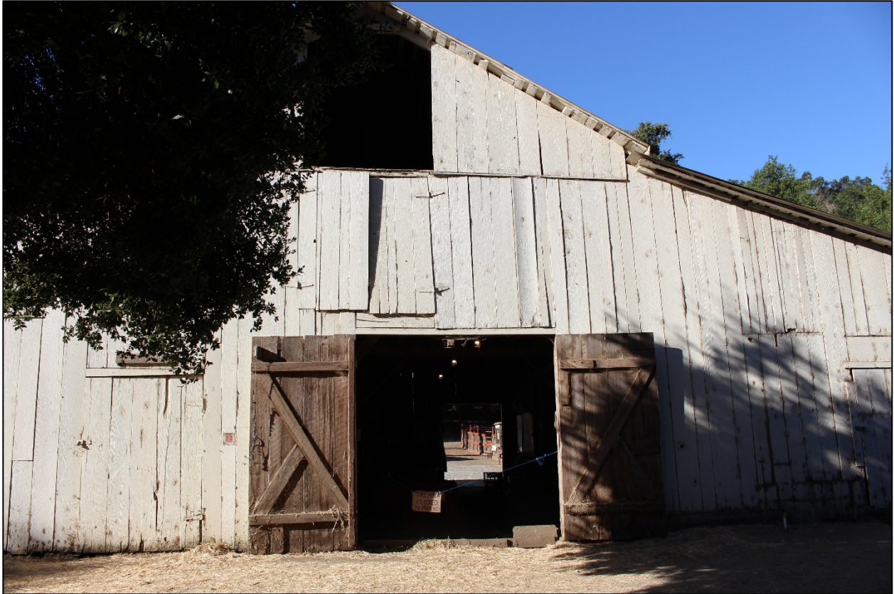
Photo 7. White Barn main gable detail with "ghost" entryways, view south.
