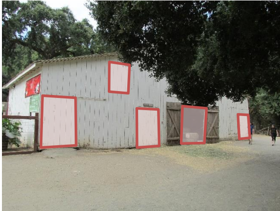
Figure 49. Door openings in north side (red boxes)
