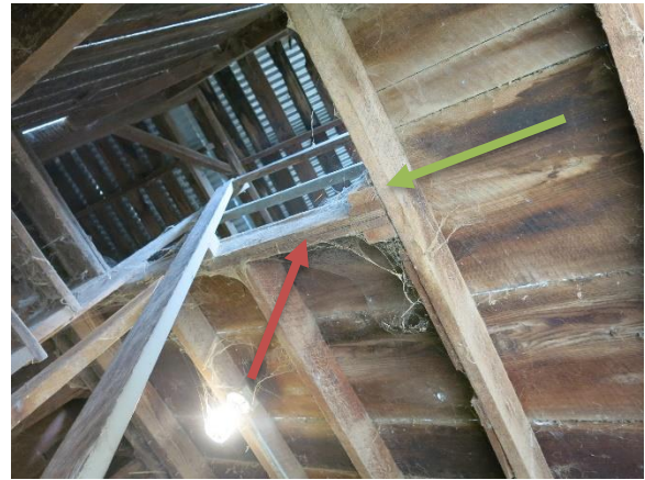
Figure 42. Attic joists supported by beam (red arrow) along the side of the stair opening. Joist (green arrow) supporting beam is overstressed.
