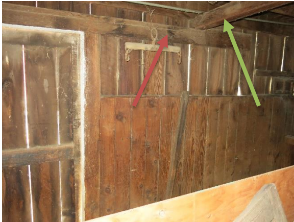
Figure 47. Door header beam (red arrow) supporting attic support beam (green arrow).
