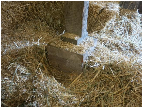
Figure 24. Wood post supported on square brick footing.
