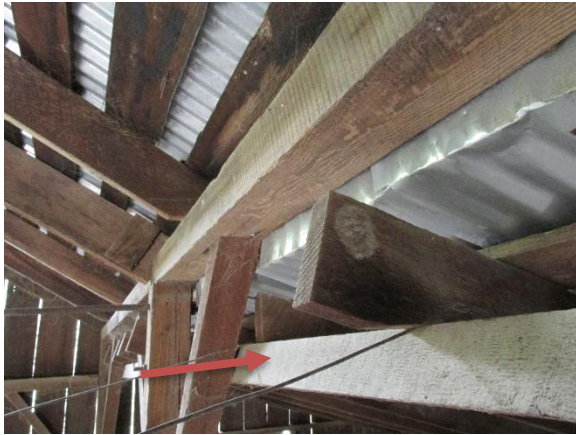
Figure 18. Wood beam (arrow) supporting west side shed roof rafters.
