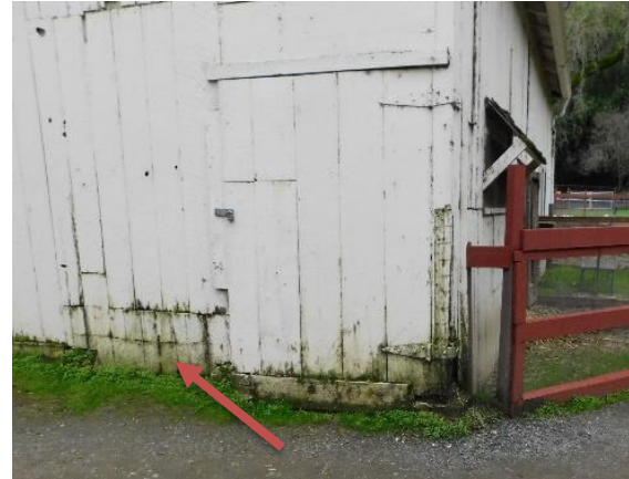
Figure 50. Deteriorated wood sheathing at the base of the north side wall (arrow).
