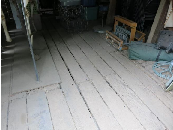
Figure 26. Wood floor in the east side of the barn.
