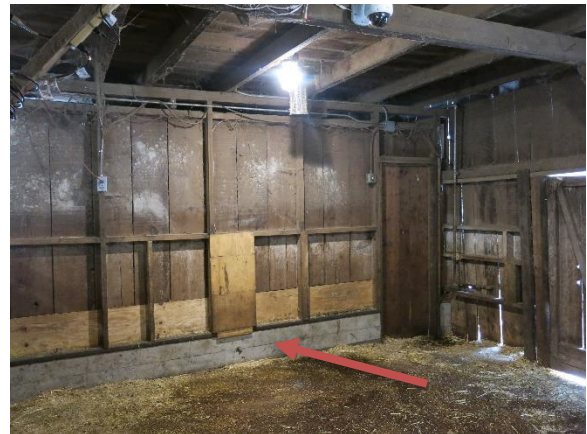
Figure 25. Concrete footing (arrow) supporting wall of the milk room.
