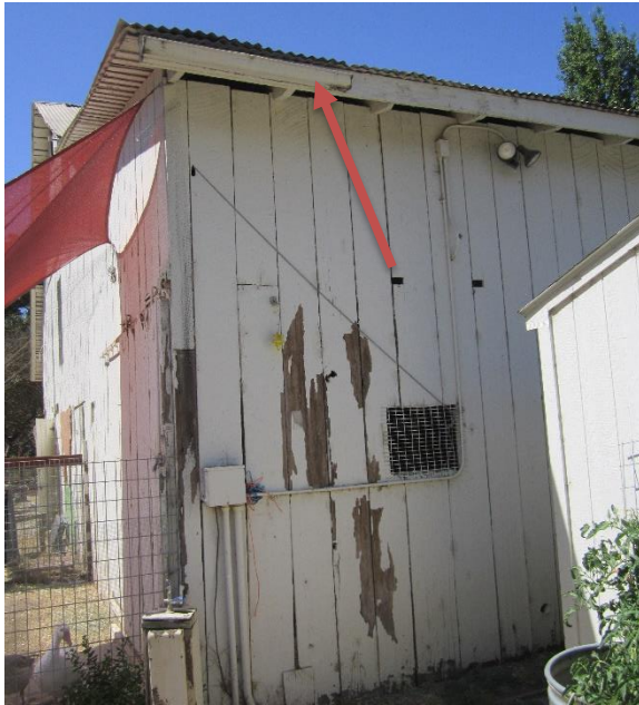
Figure 10. Short gutter at east side of the barn.
