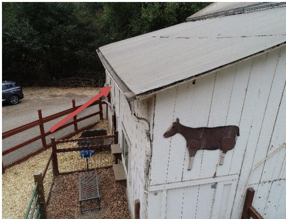
Figure 8. Gutter on the west side of the barn.
