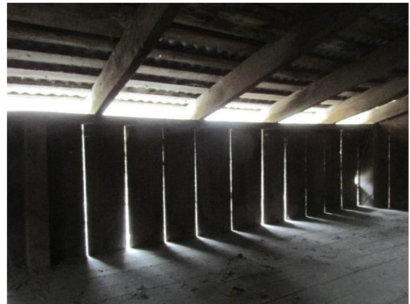
Figure 17. Roof rafters for the east side supported on the exterior wall.
