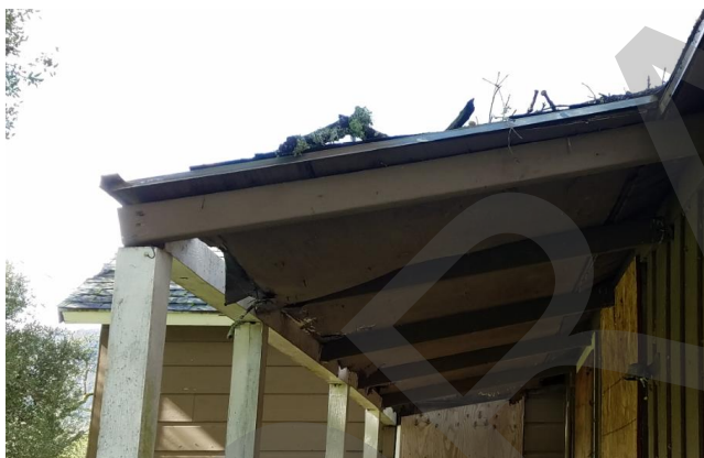
Photo 9. Partially collapsed portion of shed roof
