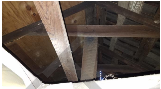
Photo 8. Hole in ceiling exposing collar ties, rafters, and 1x planking at roof
