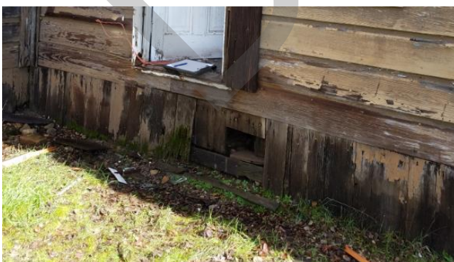
Photo 11. Moisture damage at exterior wall
