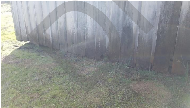
Photo 5. Deterioration of exterior siding
