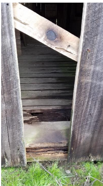
Photo 7. Deterioration at base of exterior wall
