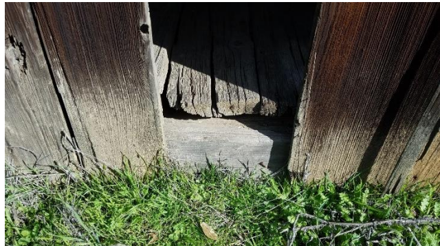
Photo 6. Deterioration at floor sheathing
