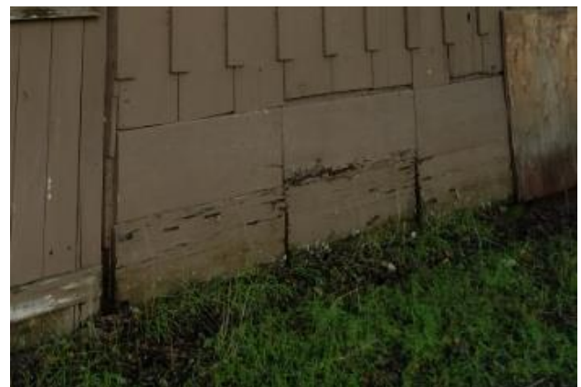
Photo 12. Moisture damage at exterior wall
