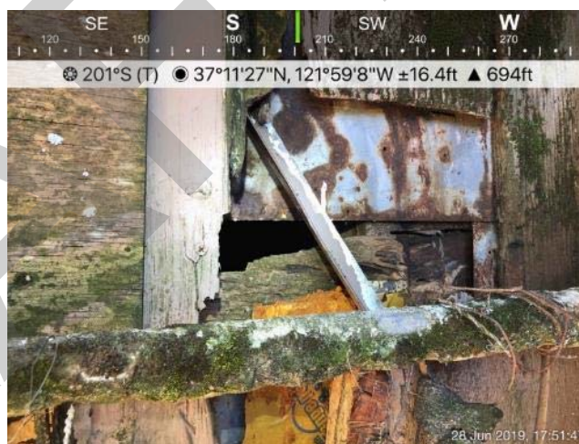
Photo 32. Hole on wall that could provide bat access.
