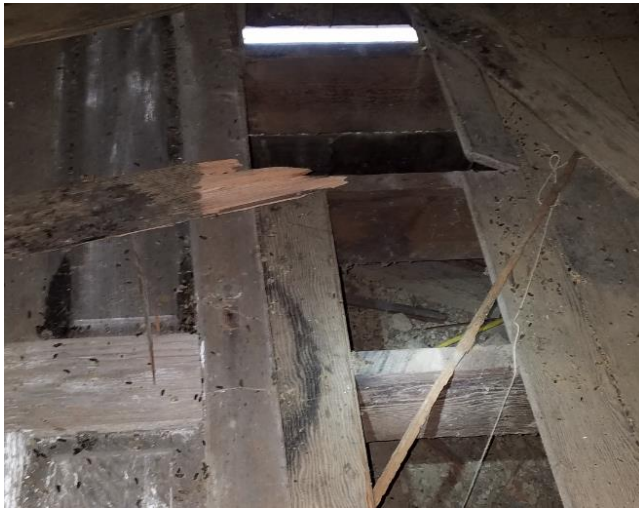
Photo 7. Missing wood planking at interior floor
