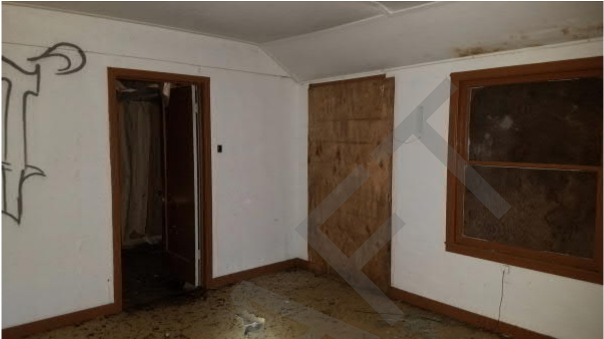
Photo 5 Material 201 ACM vinyl sheet flooring in the Beatty House
