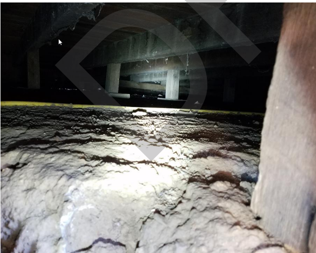
Photo 5. Interior crawlspace framing, showing posts bearing on grade or on wood sleepers
