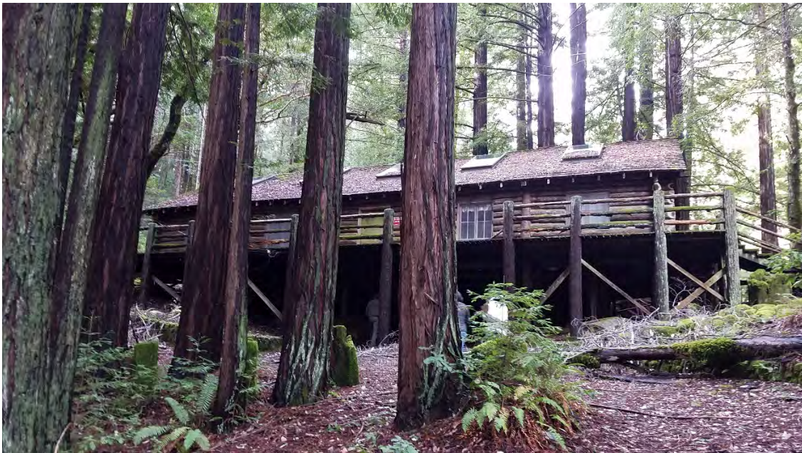
Figure 3. Primary (east) façade, facing southwest from the circular driveway.
