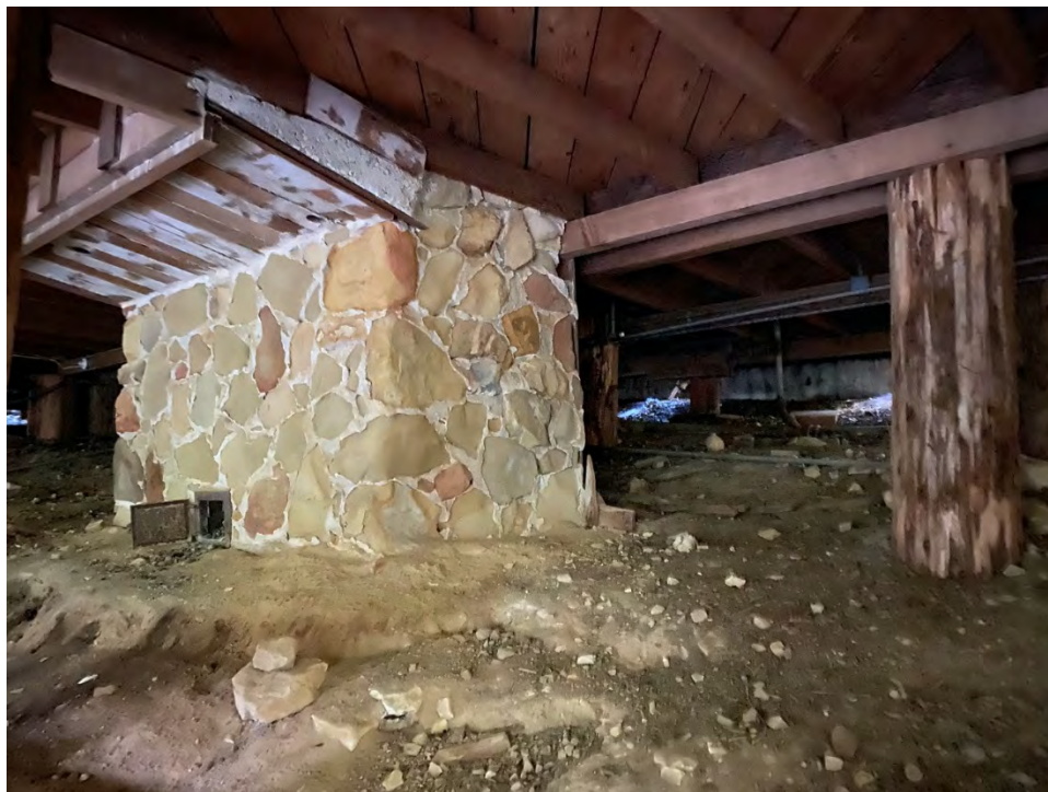
Figure 5. View of stone chimney foundation and on-grade cabin piers.
