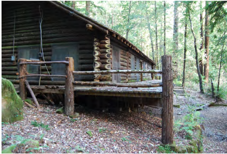
Figure 6. View of terrain, site features, and primary façade (right) and partial view of the south façade (left), facing north.
