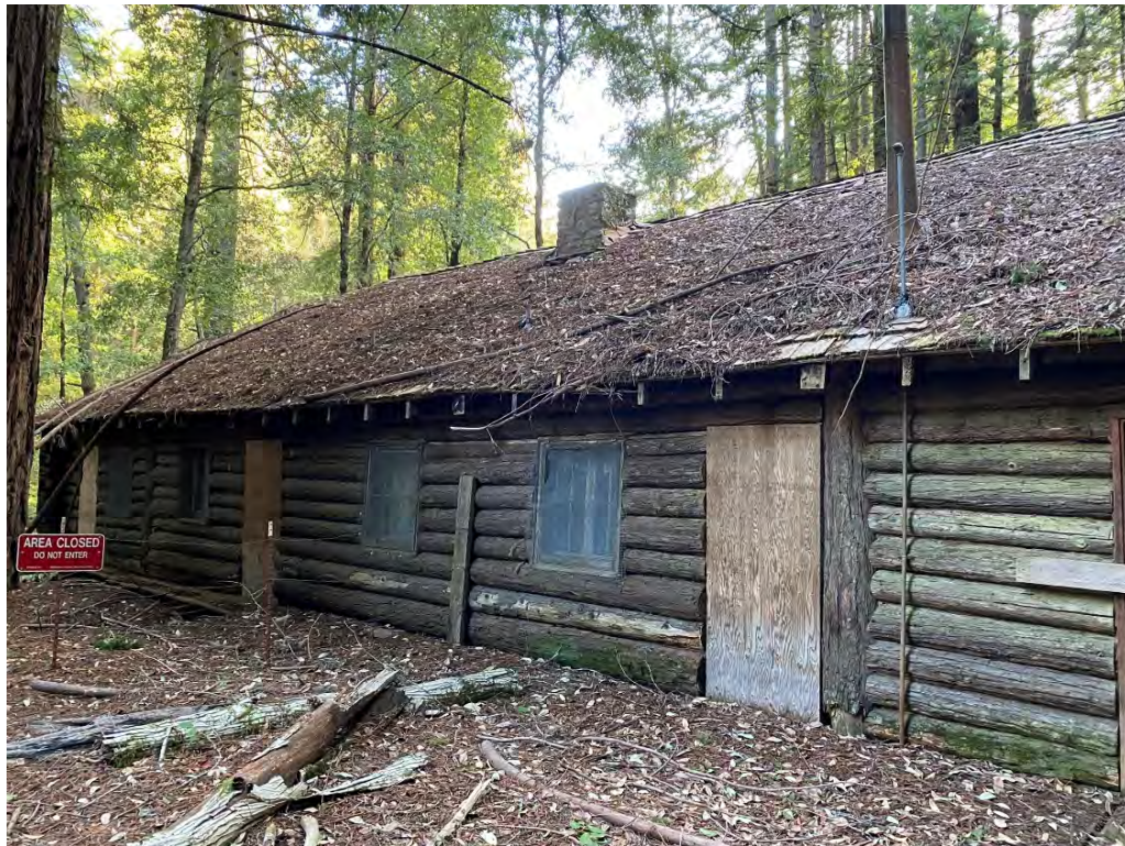
Figure 15. North half of west façade, facing north. Wraparound porch planks are located on grade, below ground cover.
