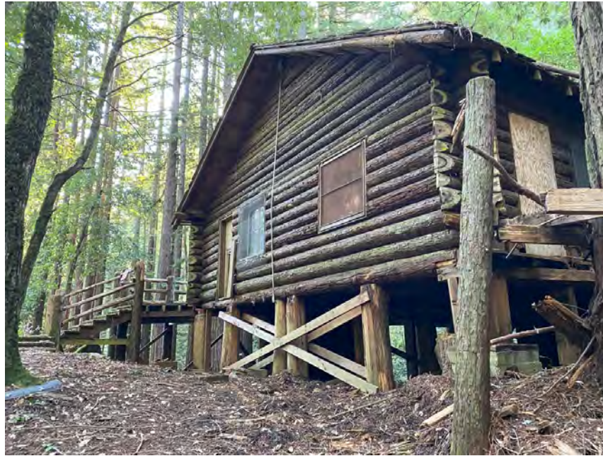
Figure 16. North façade, facing east. The wraparound porch along this façade and the porch projection (right) are no longer extant.
