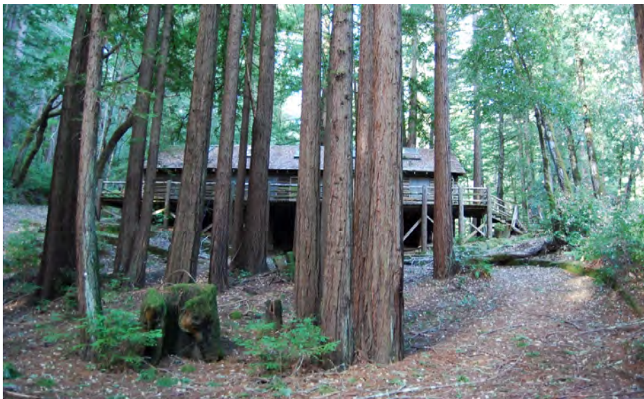
Figure 20. View of the Redwood Cabin from the dirt driveway approach, facing west.
