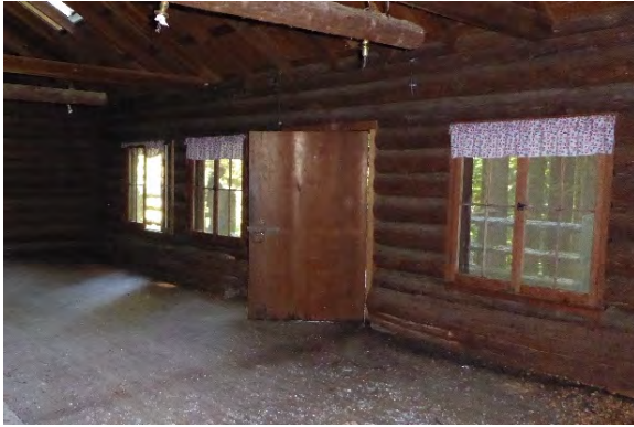
Figure 8. Front entry door and three typical wood casement windows, as seen from the interior, facing east.
