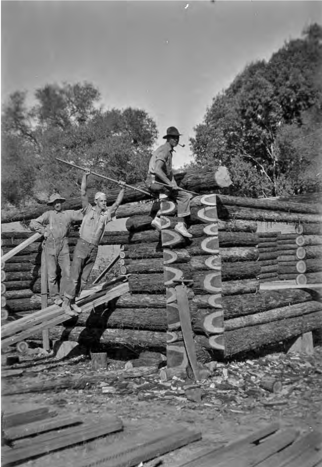
Figure 43. Antone Bordi, Lee Erickson and sons constructing the Bordi Cabin, ca. 1920s. Source: George and Mary Bordi, "Meet George and Mary Bordi," The La Honda Voice , January 29, 2011.
