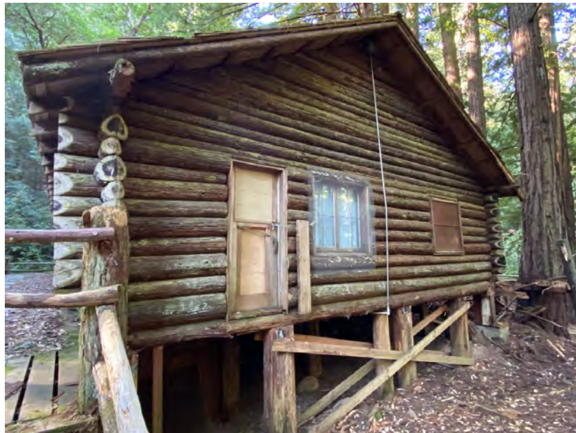
Figure 17. North façade, facing southwest from entry staircase.
