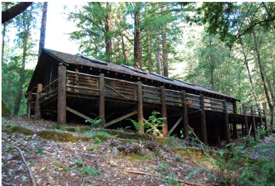
Figure 7. Primary (east) façade, facing northwest. Driveway stone walls are in the forefront.
