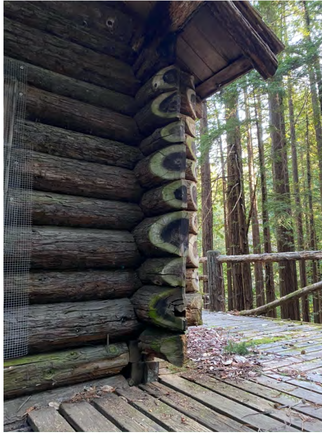
Figure 4. Close up of the cabin's typical saddle notching, facing northeast.
