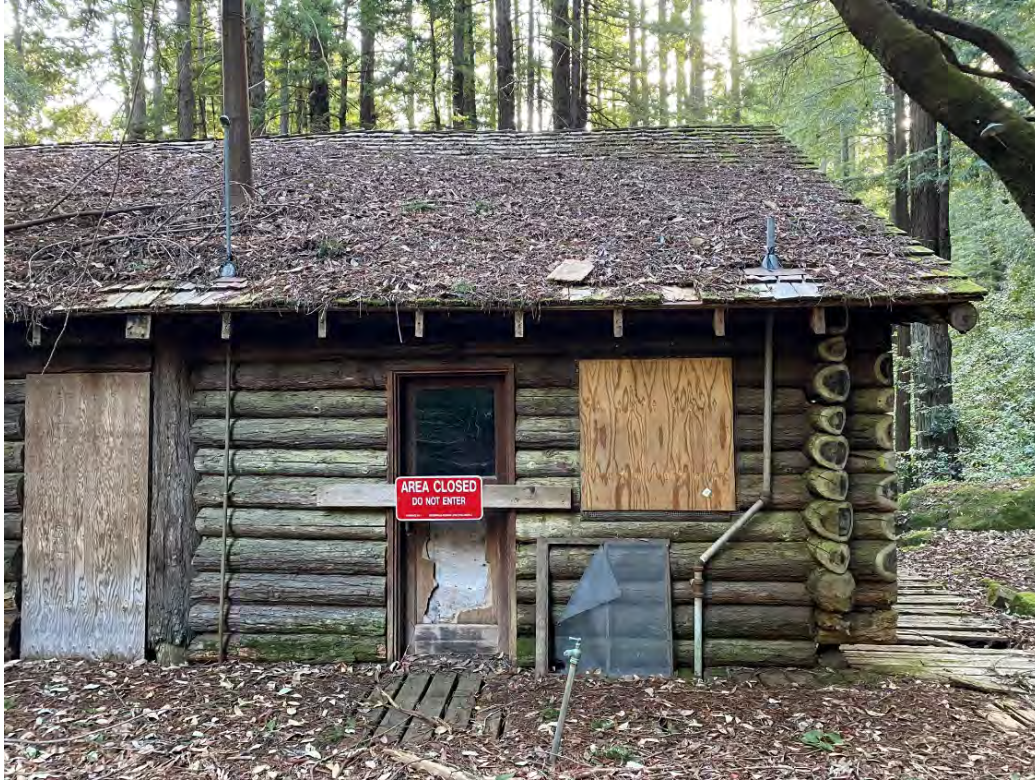
Figure 14. Close-up of south end of west façade, facing southeast.
