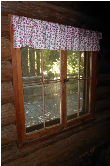
Figure 10. Typical wood sash casement window, as seen from the interior, facing southeast.
