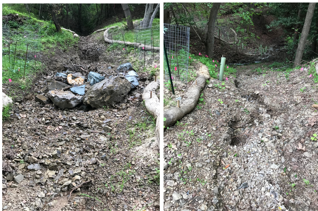
Photos 3 and 4 – Tributary 8 and 9 flows combine above the rock grade check (left) and then flow to Hendrys Creek (right). Modest erosion is noted along the banks of the tributary.
