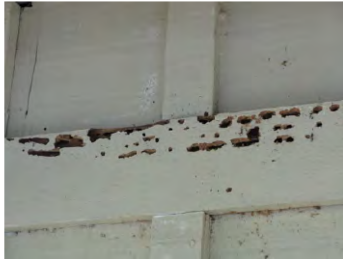
DAMAGE ON EXTERIOR
