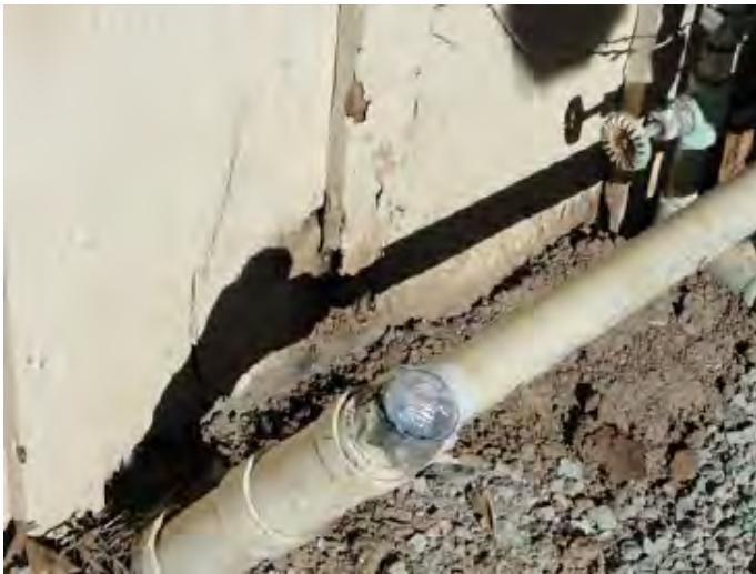
PIPES AT FOUNDATION
