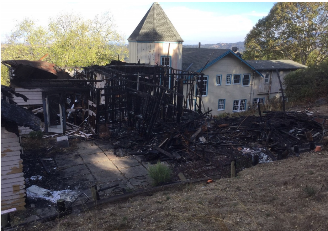
Damage to Guest House Thornewood Open Space Preserve
