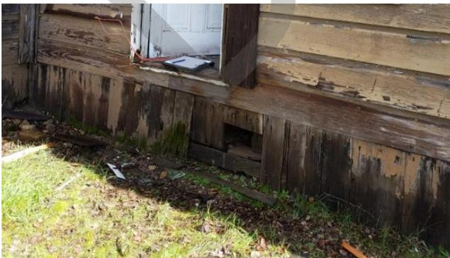
Photo 11. Moisture damage at exterior wall
