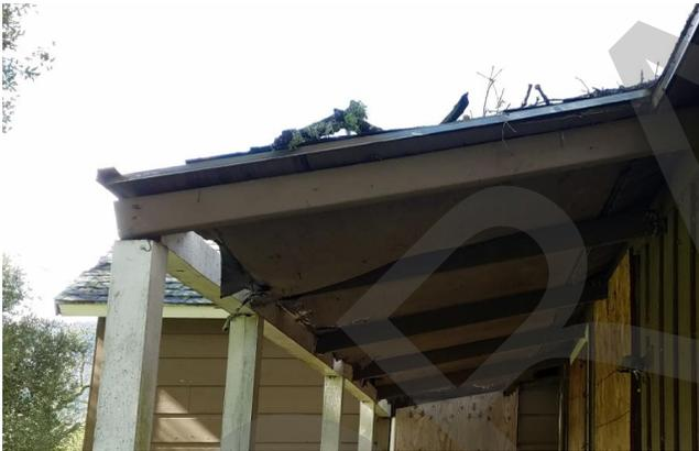
Photo 9. Partially collapsed portion of shed roof
