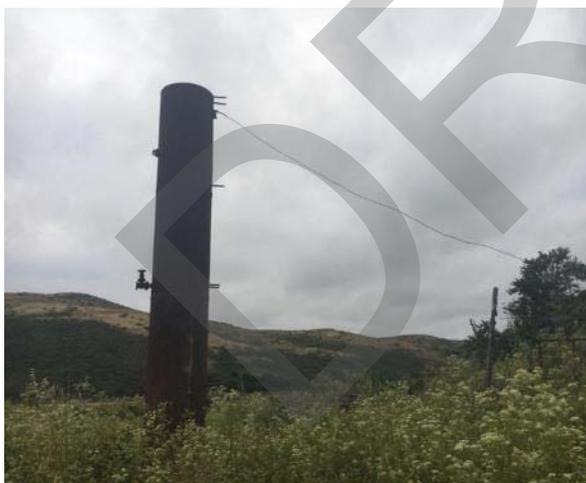
**Photo 43.** Area B – the distillation column was sealed on top but appeared to have a small opening on the left-hand side near the valve connection.
