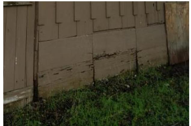
Photo 12. Moisture damage at exterior wall
