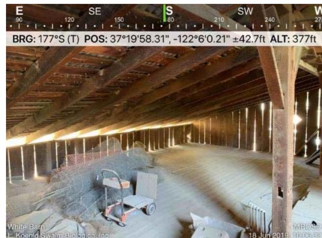
**Photo 52.** Interior of hayloft with wooden slat openings
