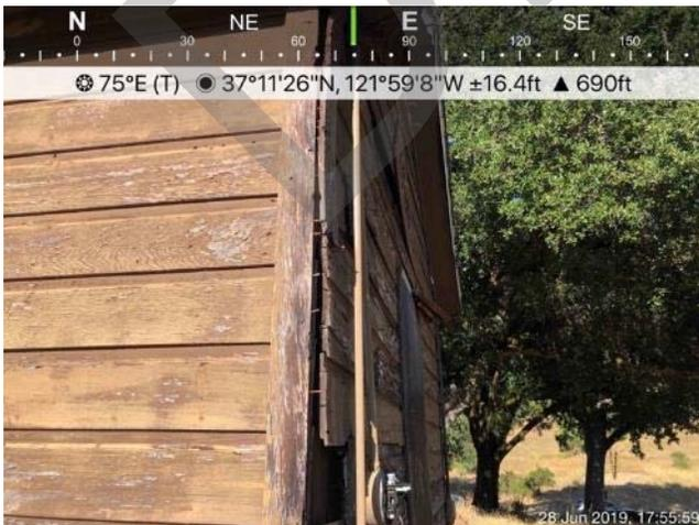
**Photo 33.** Wooden slats peeling away from the wall.
