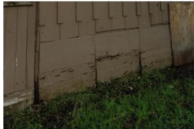
Photo 12. Moisture damage at exterior wall
