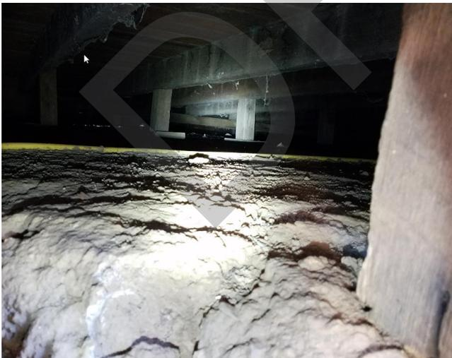
Photo 5. Interior crawlspace framing, showing posts bearing on grade or on wood sleepers
