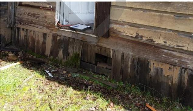
Photo 11. Moisture damage at exterior wall
