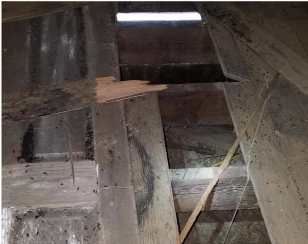
Photo 7. Missing wood planking at interior floor
