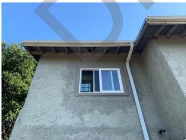
**Photo 21.** Ventilation holes under the eave of Structure A.
