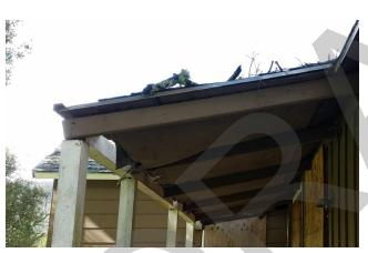
Photo 9. Partially collapsed portion of shed roof
