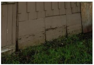
Photo 12. Moisture damage at exterior wall
