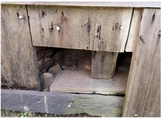
Photo 6.Missing siding on exterior wall, and lack of concrete foundation below bearing wall
