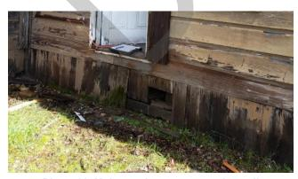
Photo 11. Moisture damage at exterior wall
