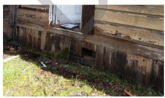
Photo 11. Moisture damage at exterior wall
