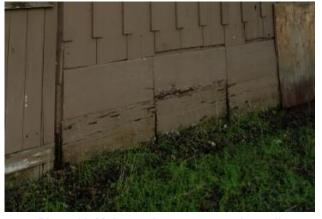
Photo 12. Moisture damage at exterior wall
