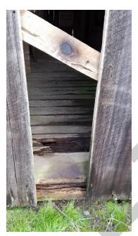
Photo 7. Deterioration at base of exterior wall
