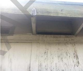
**Photo 48.** Area E – openings underneath the roofline of the hunting cabin.
