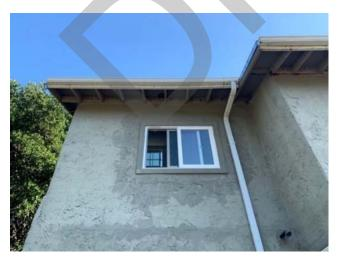
Photo 21. Ventilation holes under the eve of Structure A.
