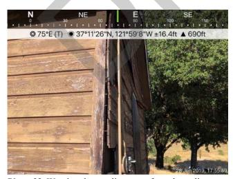
Photo 33. Wooden slats peeling away from the wall.
