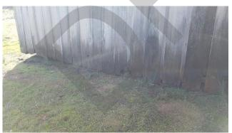
Photo 5. Deterioration of exterior siding
