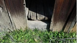
Photo 6. Deterioration at floor sheathing
