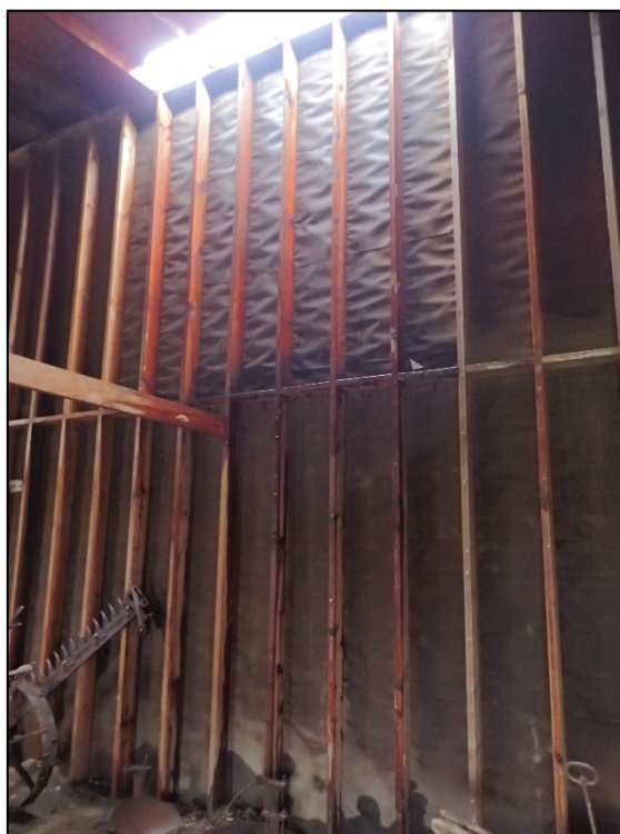
Smith Barn – interior wall, east façade. LSA photograph, 12/22/2021.
