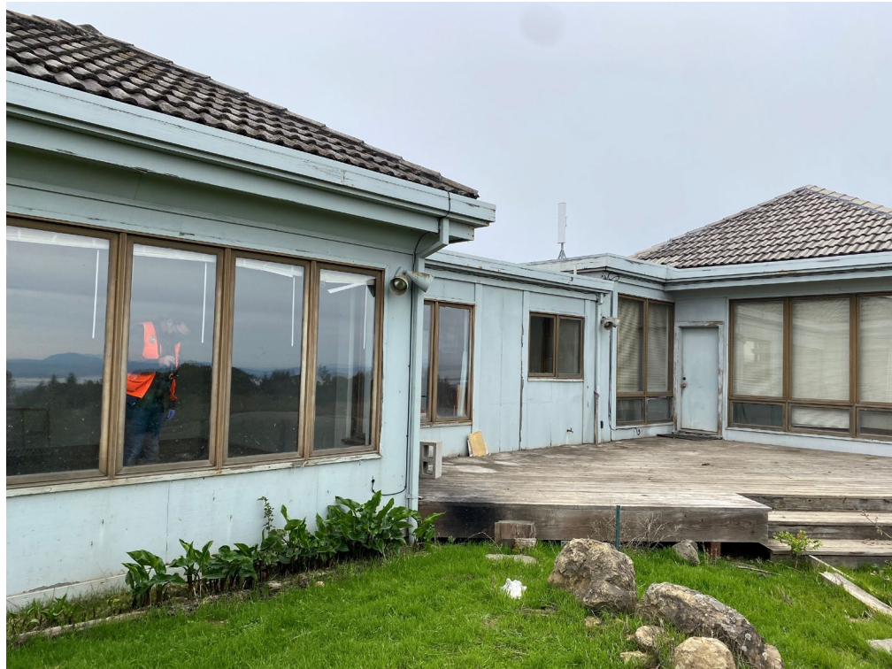
Smith House, North Elevation.
