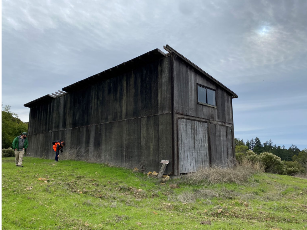
Smith Barn Exterior, East Elevation.
