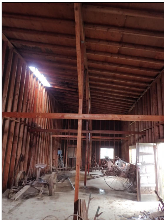
Smith Barn – interior. View south through interior space. LSA photograph, 12/22/2021.
