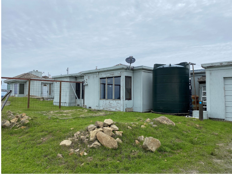
Smith House Exterior, South Elevation.
