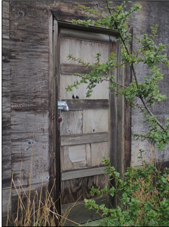
Smith Barn – west façade, primary entrance. LSA photograph, 12/22/2021.
