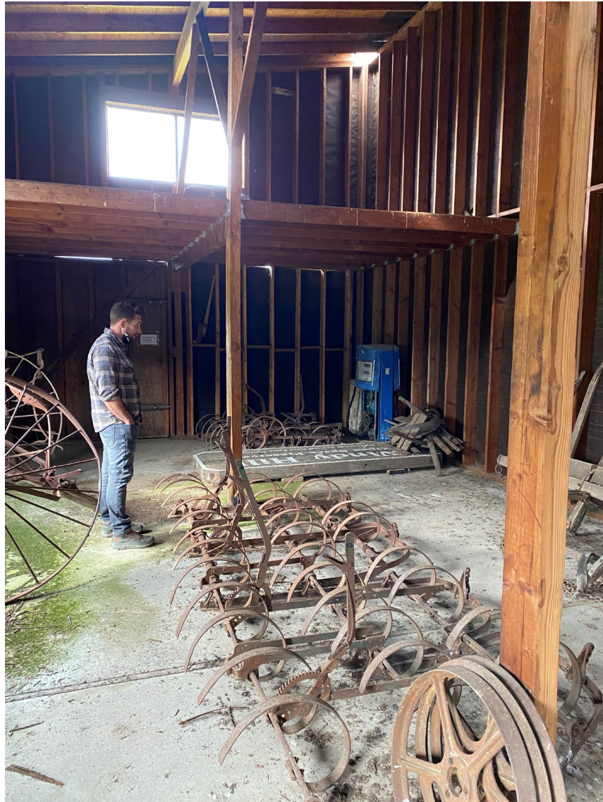
Smith Barn, Interior.
