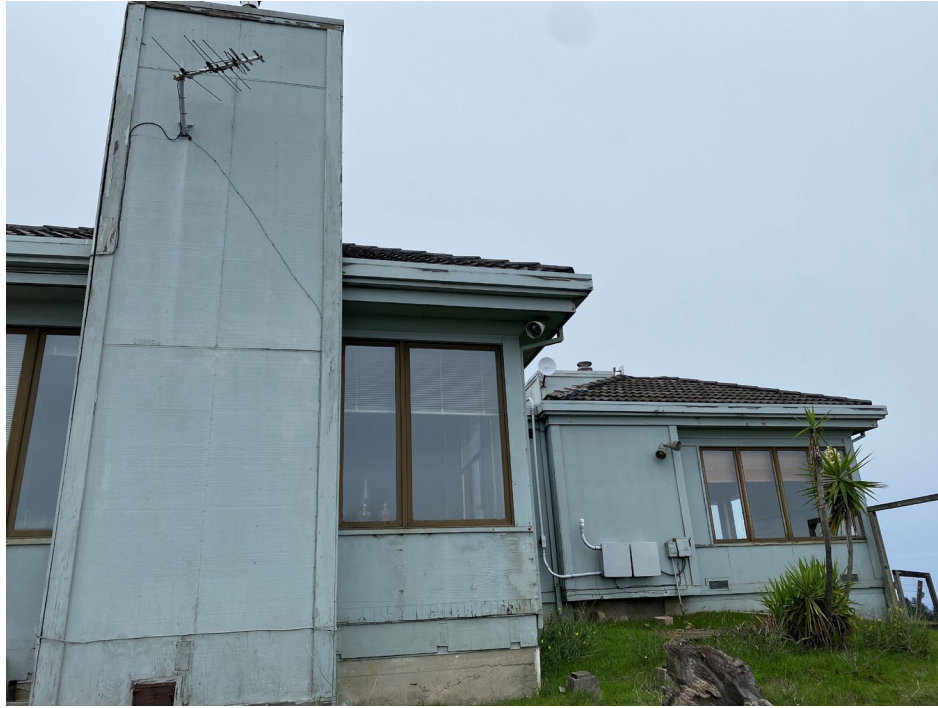
Smith House Exterior, West Elevation.
