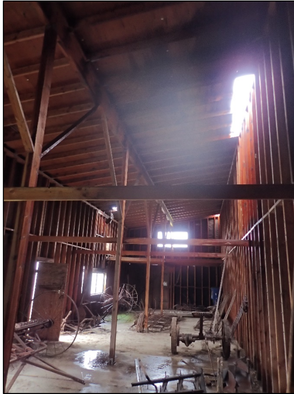
Smith Barn – interior. Southeast corner view northwest. LSA photograph, 12/22/2021.
