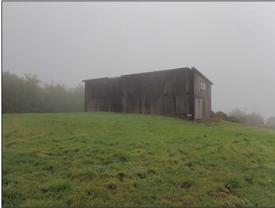
Smith Barn – east and north façades, view to the southwest. LSA photograph, 12/22/2021.
