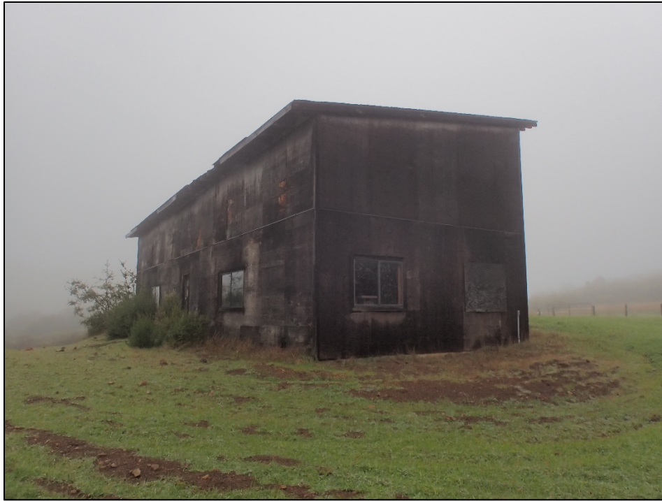
Smith Barn – south and west façades, view to the northeast. LSA photograph, 12/22/2021.
