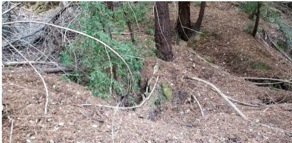
Photo 7: Two gullies at partially washed out watercourse crossing. The upper gully is from diverted stream flow coming down from MP8. The lower gully is from the watercourse.
