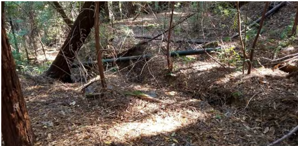
Photo 3: Partial washed out fill crossing
