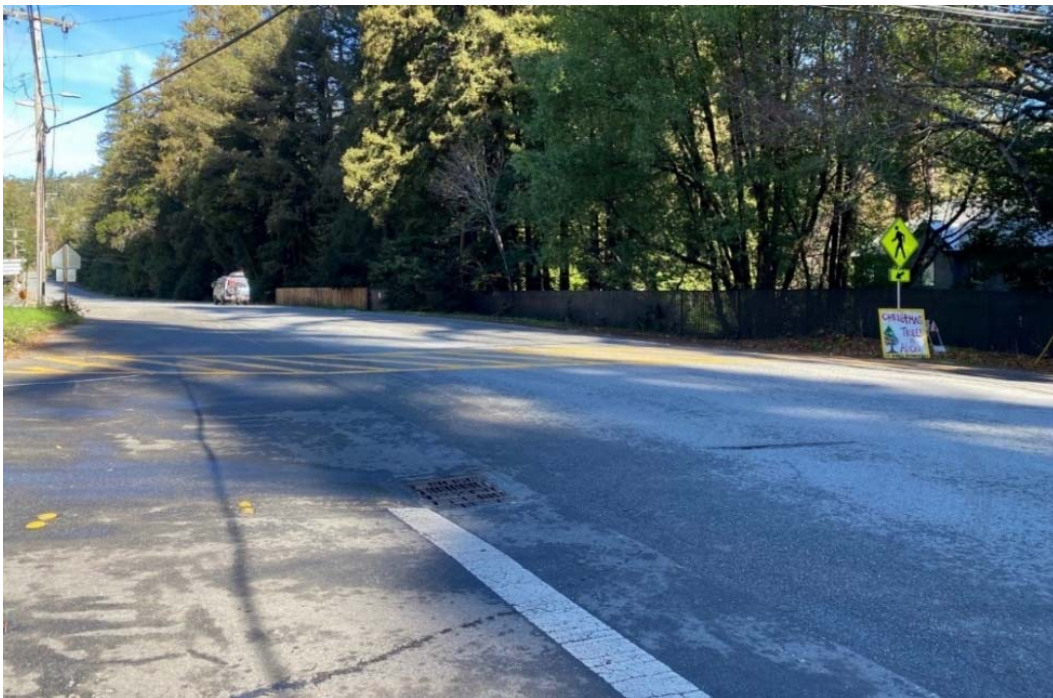
Figure 3-B2-5 SR-84 at Sears Ranch Road facing north
