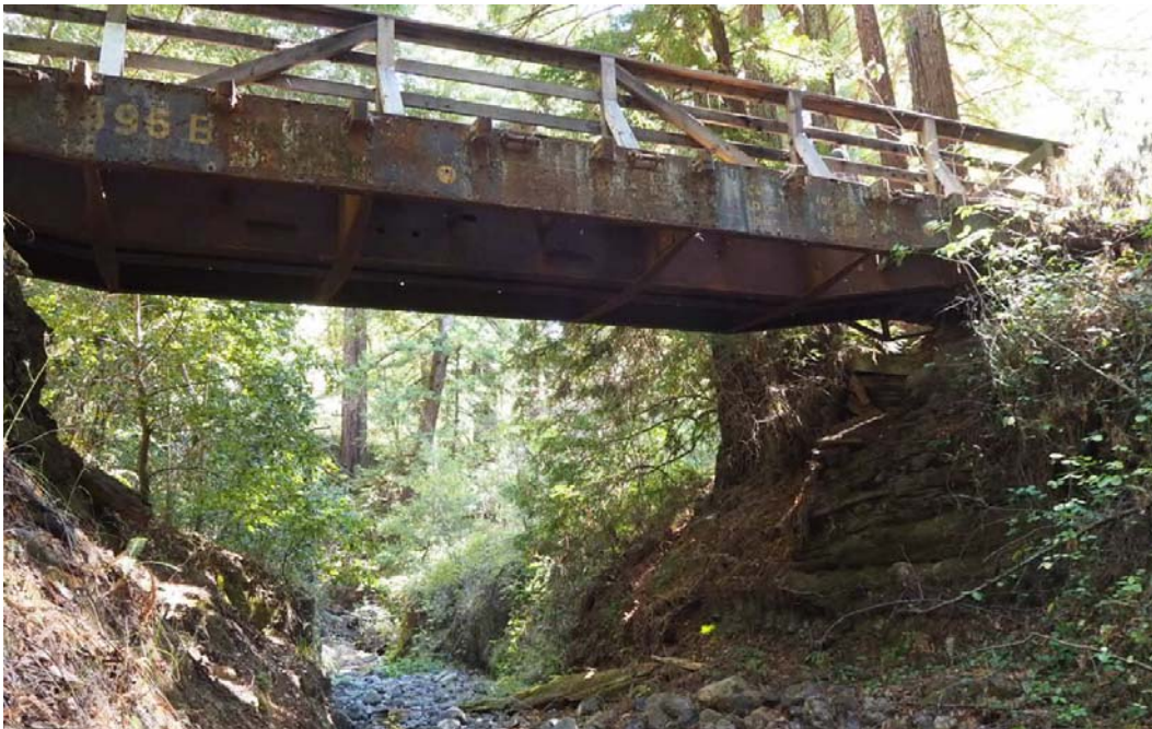
Figure 3-Br-2 Bridge over La Honda Creek at Site D facing west
