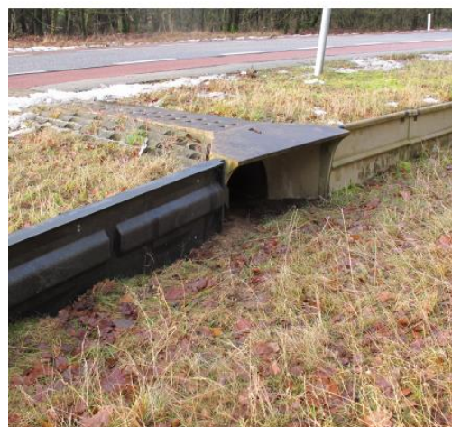
Example of a Guide Wall (from Langton and Clevenger 2021)
