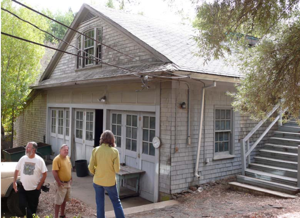
A 2008 image of the Garage at the Hawthorns site. Visible are the paneled and glazed garage doors, the shingling, the arched window at the attic and the exterior stairs to the upstairs apartment.
