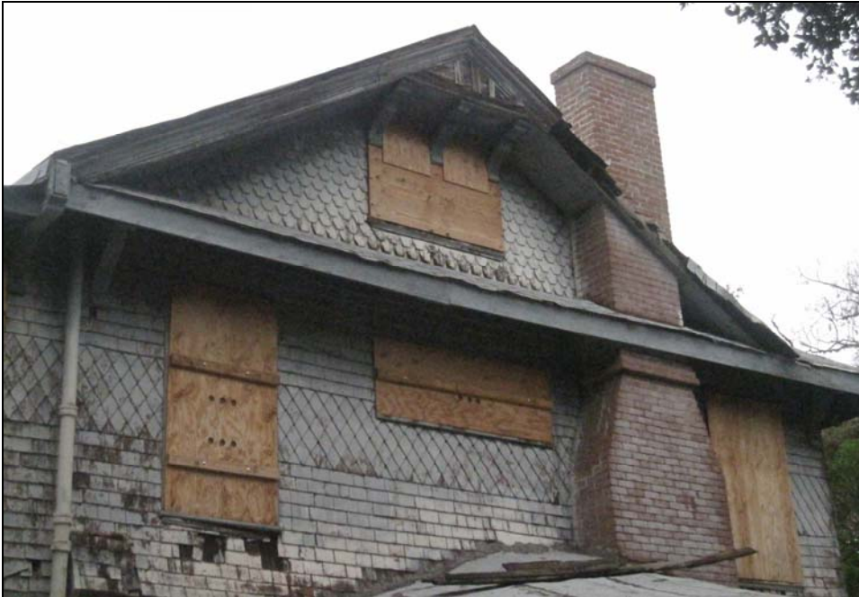
An exterior detail showing the character-defining shingles, brick chimney, gable roofs, and roof brackets. Photograph B. Maley, March 2013.
