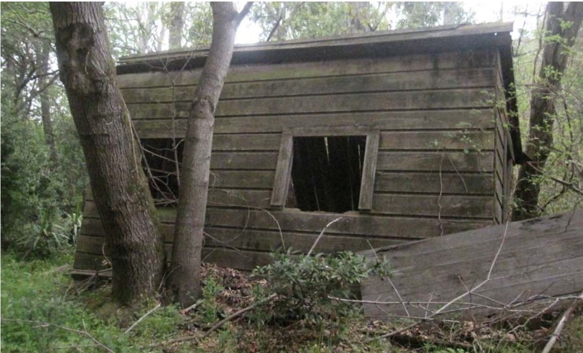
Below: The Pump House. Photograph B. Maley, March 2013.
