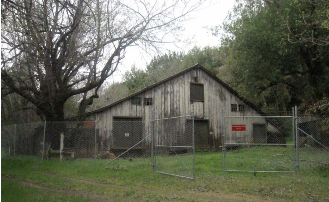
The north elevation of the Lower Barn. Photograph B. Maley, March 2013.
