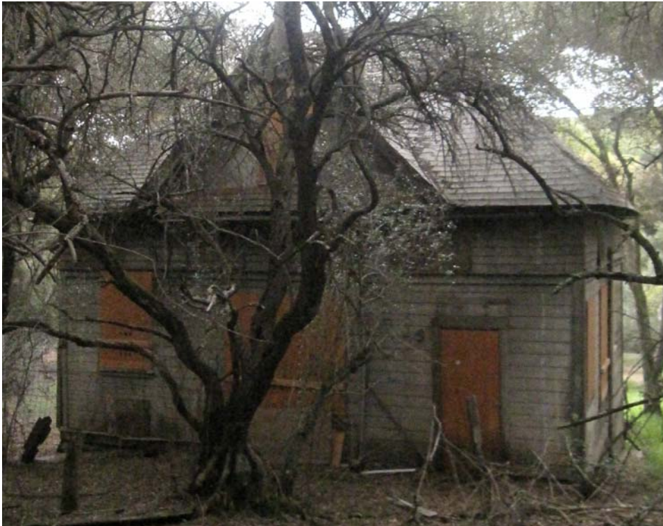
A view of the rear (west elevation) of the Cottage showing the overhanging hipped roof and the steeply pitched dormer. Photograph B. Maley, March 2013.
