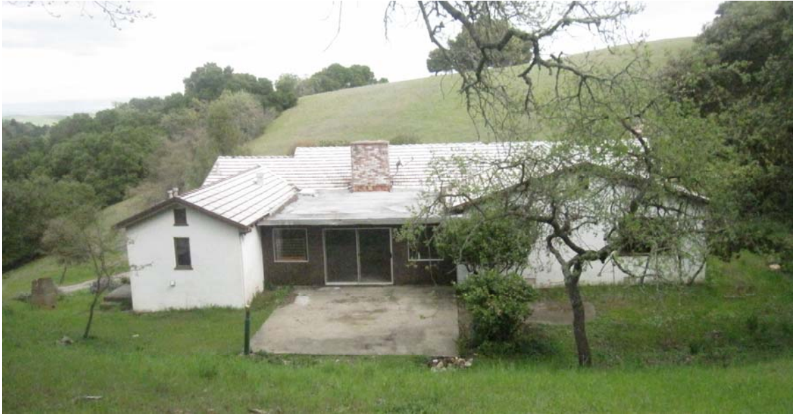
Above: The rear elevation of the Alpine Road House, showing the u-shaped plan and rear patio. Photograph B. Maley, March 2013.
