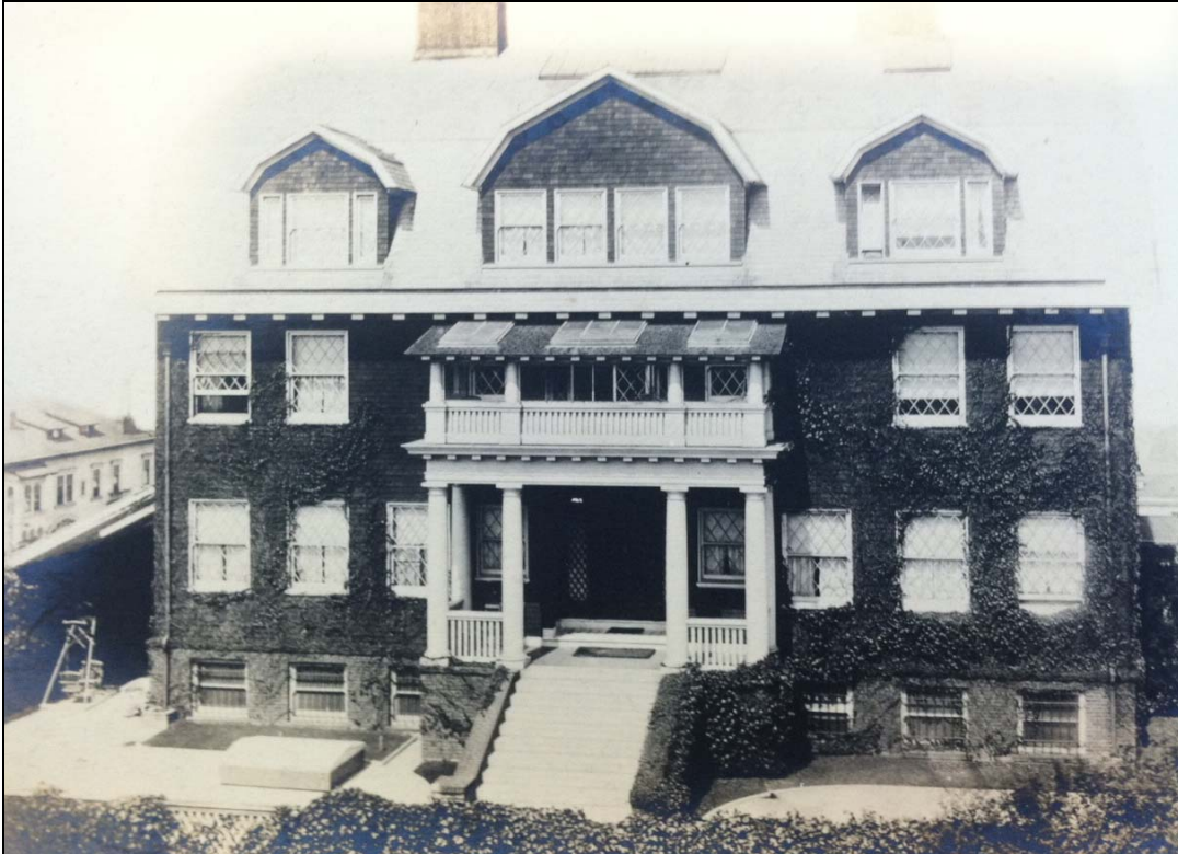
The Edwin and Virginia Newhall house at 2950 Pacific Avenue in San Francisco. This view is not easily seen as the house sits back from Pacific Avenue. The rear of the house is quite visible from below on Broadway. Designed by Albert Farr around 1904, the design was apparently heavily influenced by Mrs. Newhall. The style and features of the house greatly reflect the Martha's Vineyard cottages and houses that Virginia greatly admired and wanted to emulate on the West Coast.
