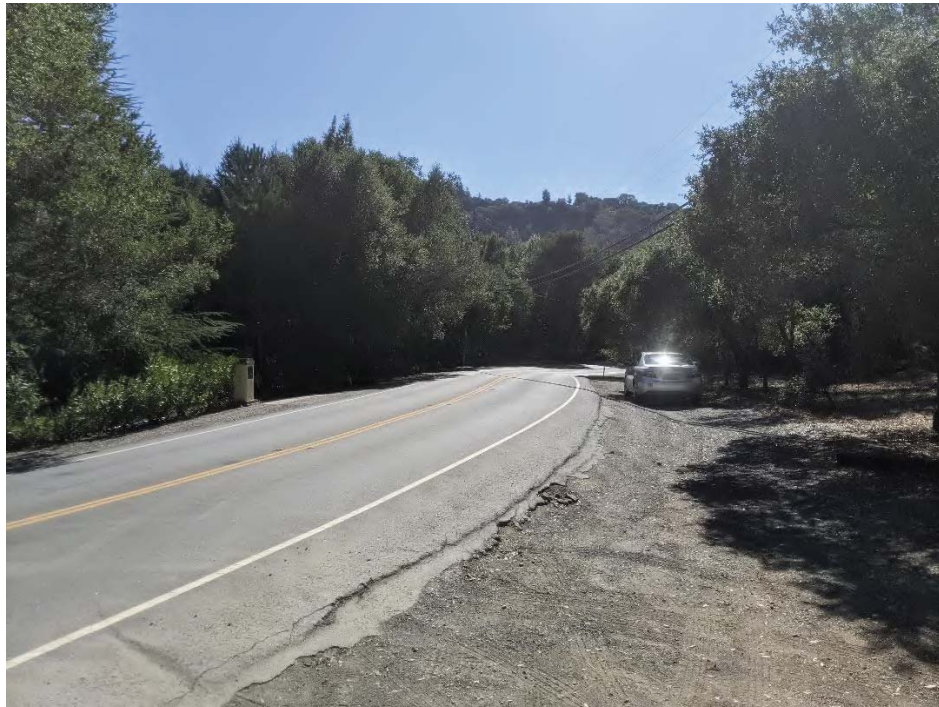
North Los Trancos Rd Driveway Looking South
