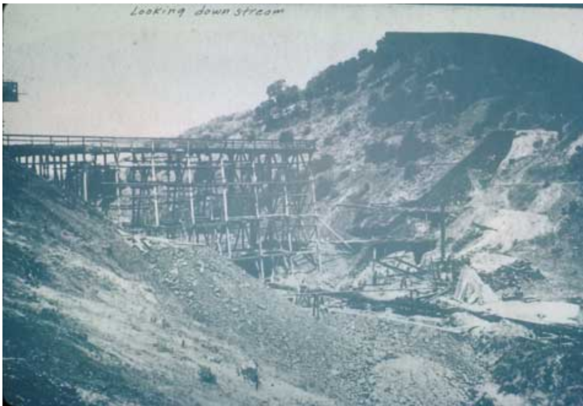
The Searsville Dam under construction around 1890.
