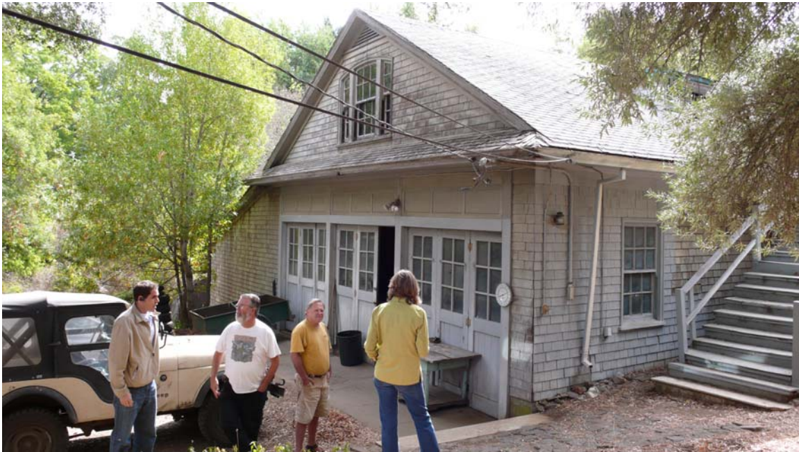
The north elevation of the Garage photographed in 2008 showing the original, paneled garage doors before they were boarded up.
