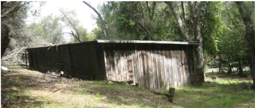
The Upper Barn near the entry to the site off Los Trancos Road. Photograph B. Maley, March 2013.
