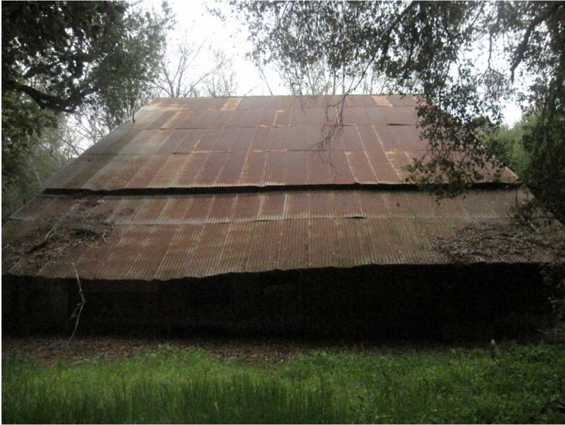
The metal roof of the Lower Barn. Photograph B. Maley, March 2013.
