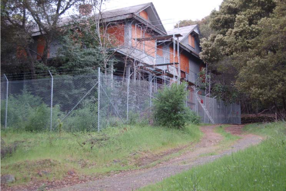
Above: Section of the internal road system that runs in front of the Hawthorn House. Photograph Denise Bradley, March 2013.
