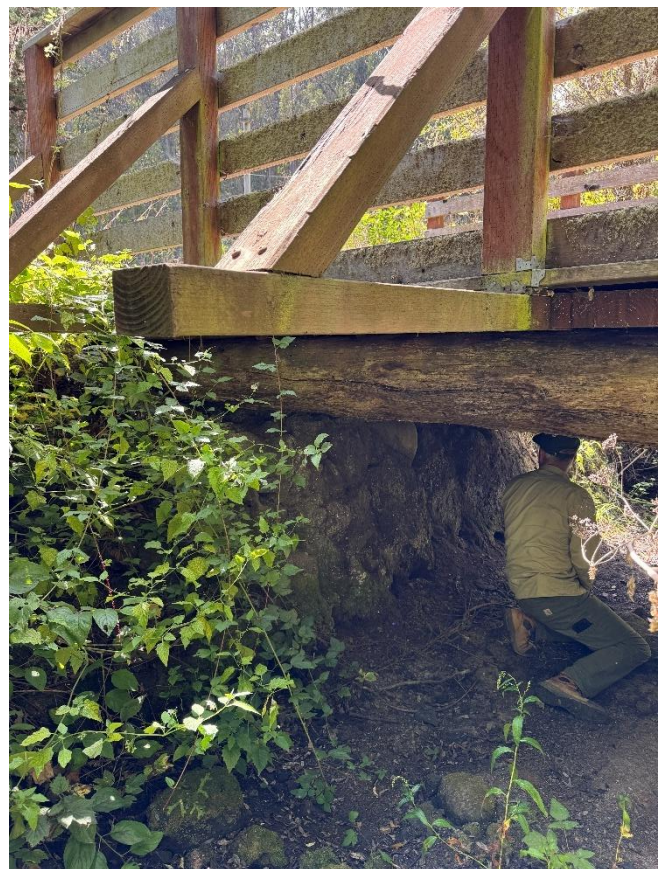
Figure 2, 3. Timbered supports and guard rails (addition by District staff). Creek bed with vegetation. Photograph taken in September 2025.
