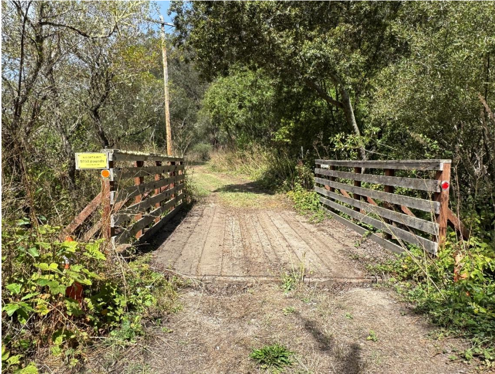
Figure 1. Miramontes (Madonna) Bridge, facing west.
