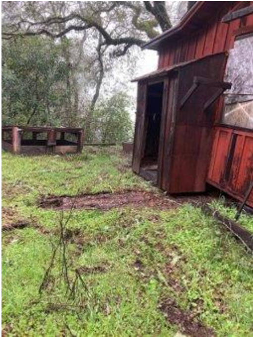
Sink hole at leach field.
