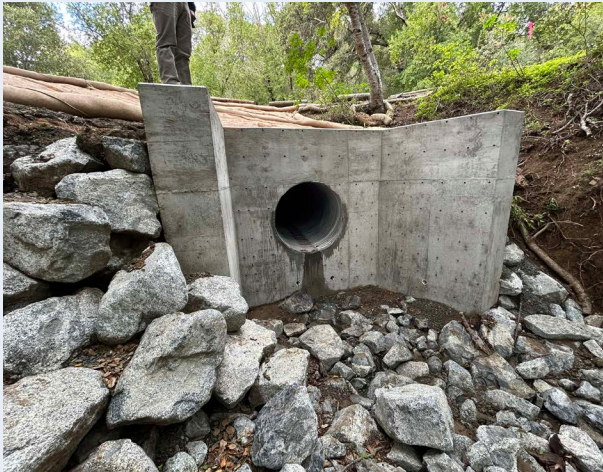
A completed Prospect Road culvert replacement at the main access road into Fremont Older Open Space Preserve. Fremont Older Open Space Preserve (Zach Alexander)
