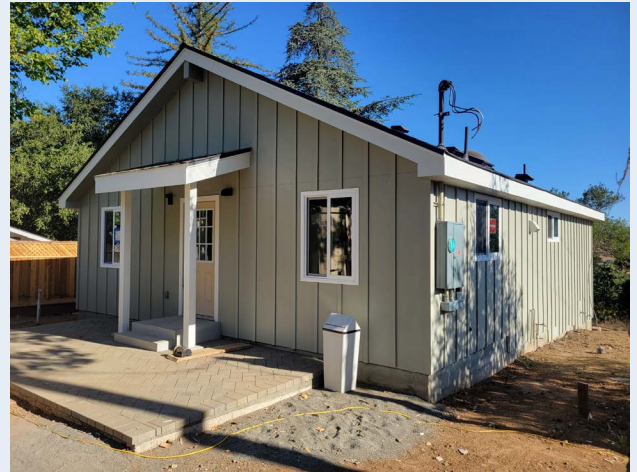
Structure improvements completed to serve as a new ranger residence. Sierra Azul Open Space Preserve (Paul Kvam)
