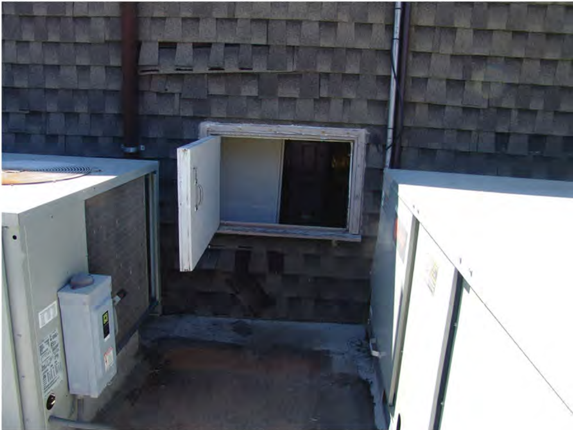
Figure 3 Entrance to the Roof Well - Crawl Space (Dimension is ~ 2 x 3 ft.)
