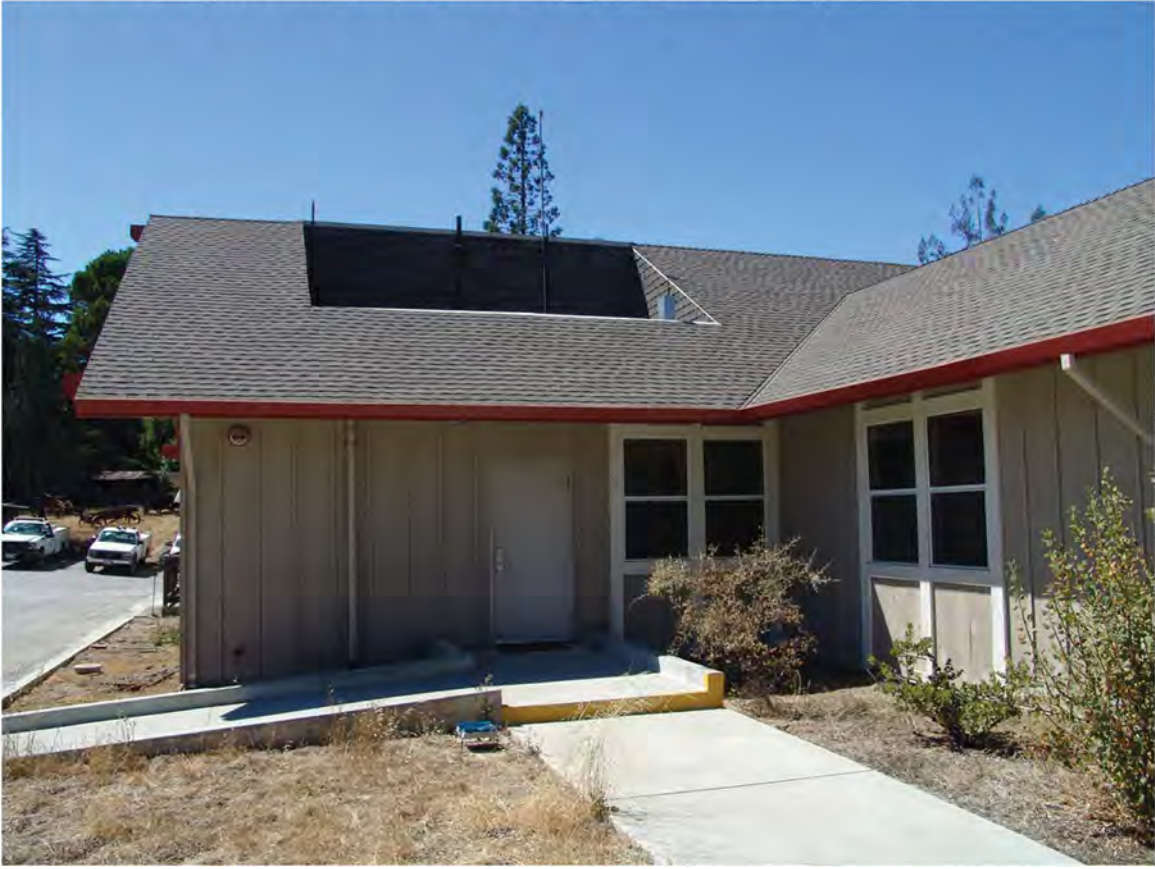
Figure 2 Existing Roof Well, Skyline Field Office, and Surroundings
