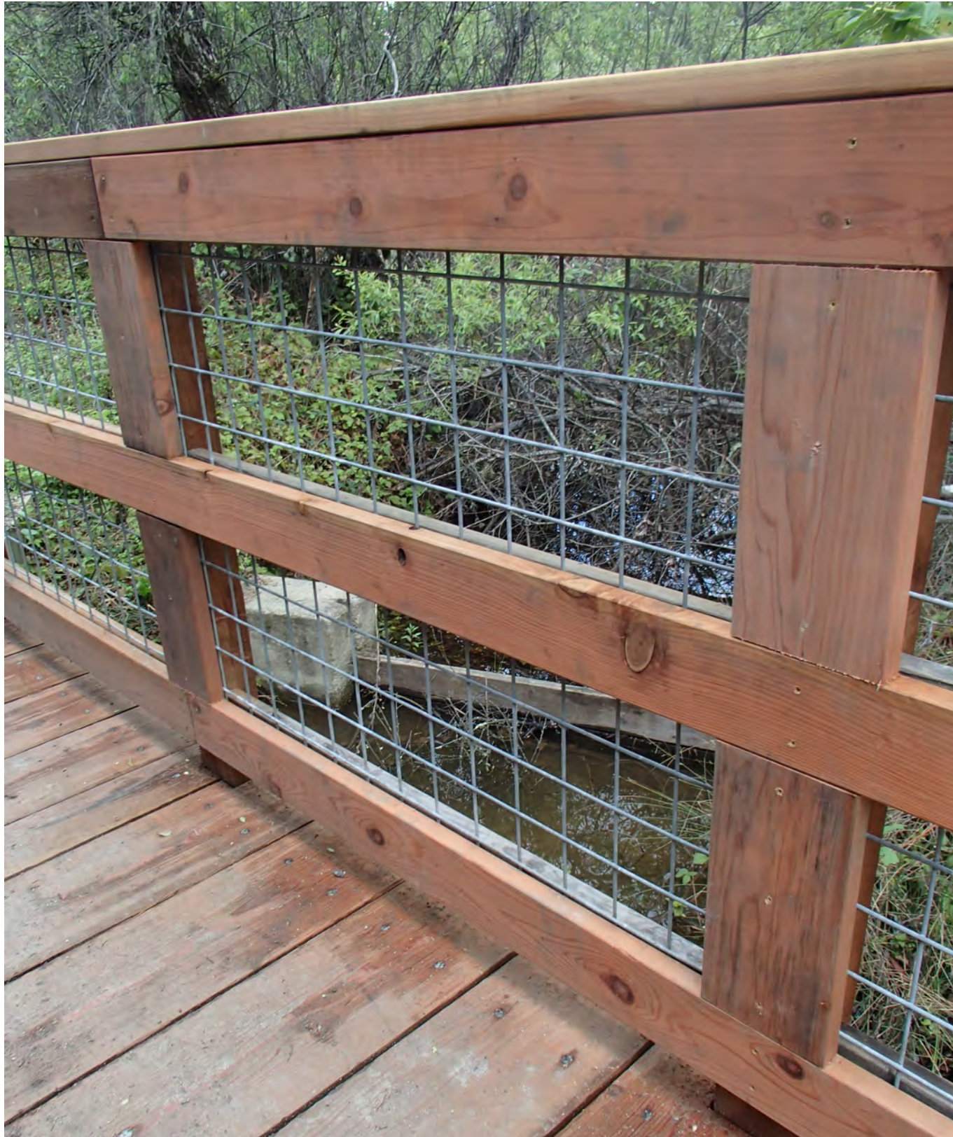
Exhibit C2: Welded Wire Mesh Detail
