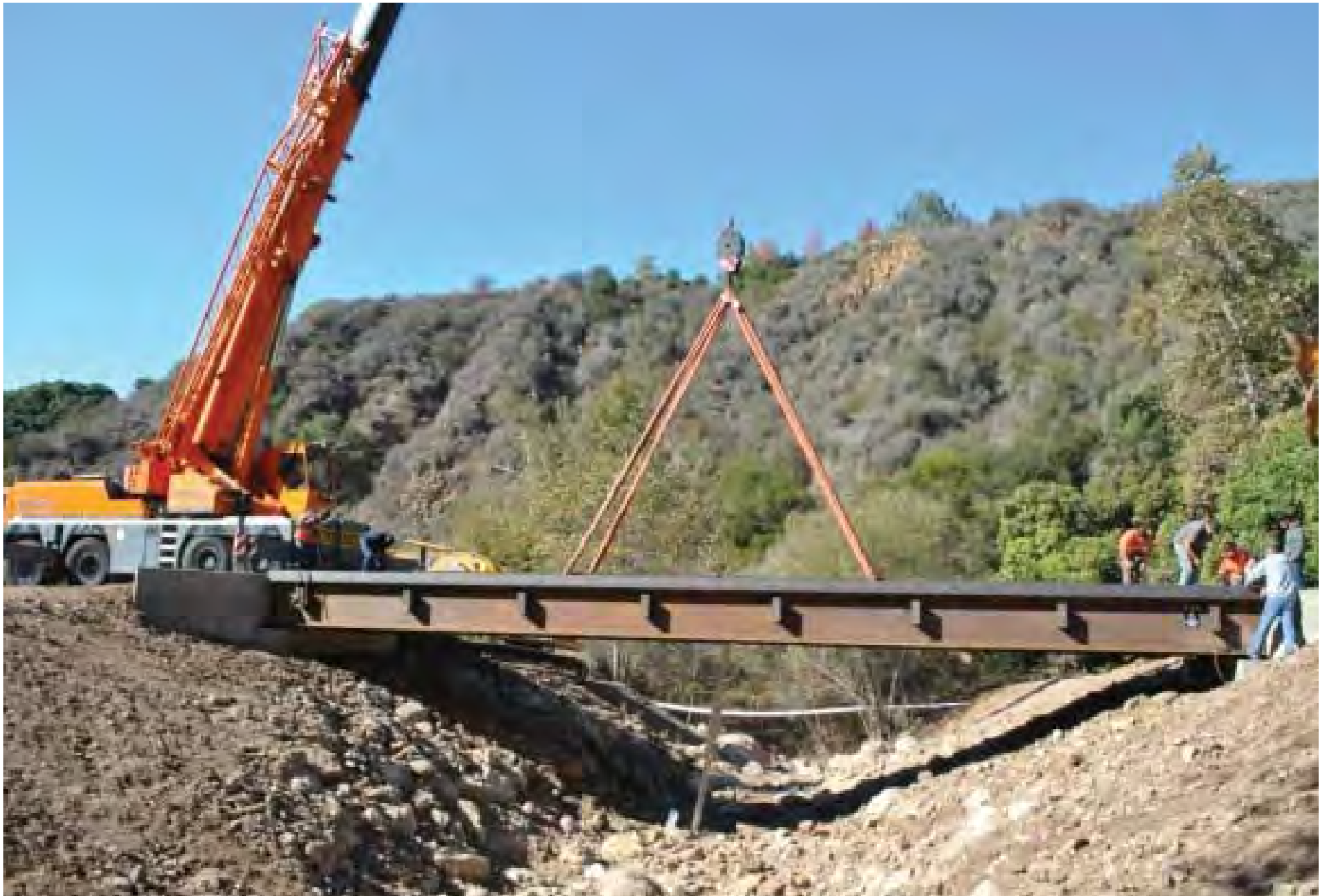
Exhibit B2: I-Beam Bridge Typical
