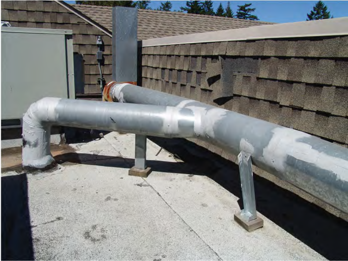
Figure 4 Interior of Roof Well, Ventilation Ducts to Remain
