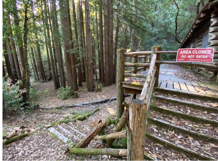
Figure 19. Entry staircase at northeast corner of the Redwood Cabin, facing southeast.
