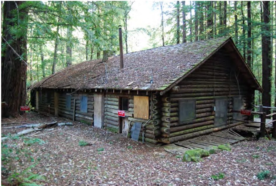
Figure 13. View of west façade (left), and south façade (right), facing northeast.
