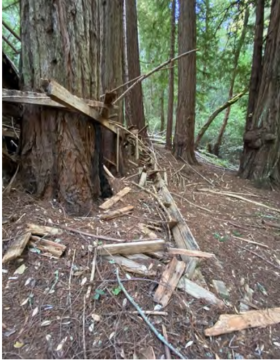
Figure 18. Remnants of rear porch projection at the northwest façade.
