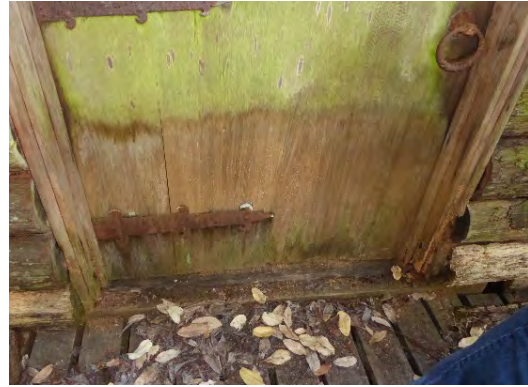
Figure 9. Detail of front entry door and ironwork.
