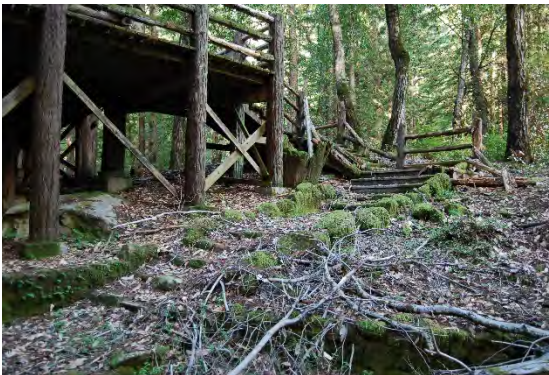
Figure 23. View of the U-shaped entry staircase, facing north.
