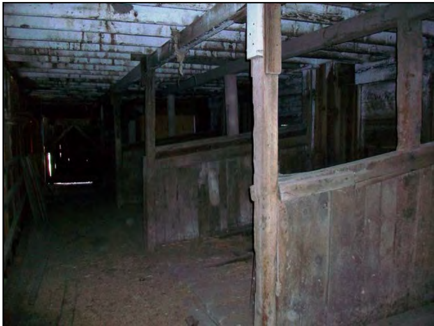
Red Barn, La Honda Creek Open Space Preserve, interior. View of animal feed pens. View north from shed-roof addition, west façade 6/21/16.
