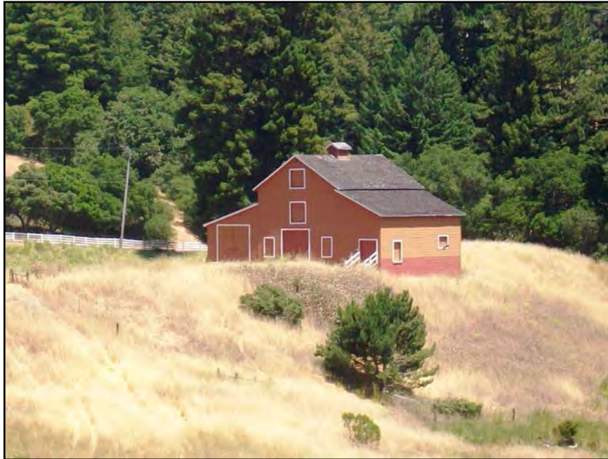
Red Barn, La Honda Creek Open Space Preserve, north and west façades. View to the southeast. 6/21/16.
