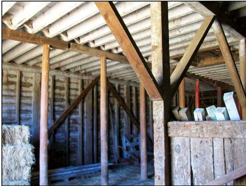
Red Barn, La Honda Creek Open Space Preserve, interior. View southeast from northwest corner. 6/21/16.
