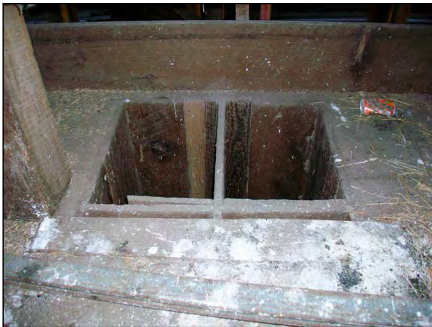
Red Barn, La Honda Creek Open Space Preserve, interior. Detail view of animal feed chutes. Upper floor of shed roof addition, west façade. 6/21/16
