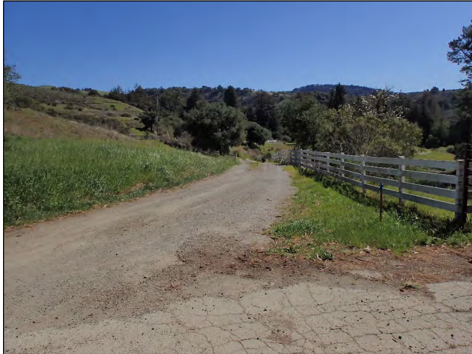
Internal road to Red Barn and Corral. View south. LSA photograph, 3/10/22.
