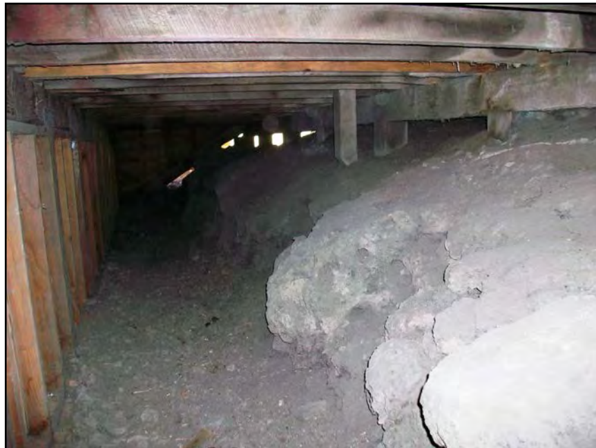
Red Barn, La Honda Creek Open Space Preserve. Detail view of foundation repairs and floor joist reinforcements. South façade, view north. 6/21/16.
