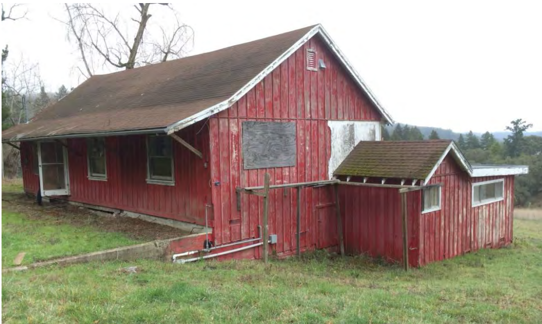
Figure 2 McDonald Ranch House – North and East Elevations
