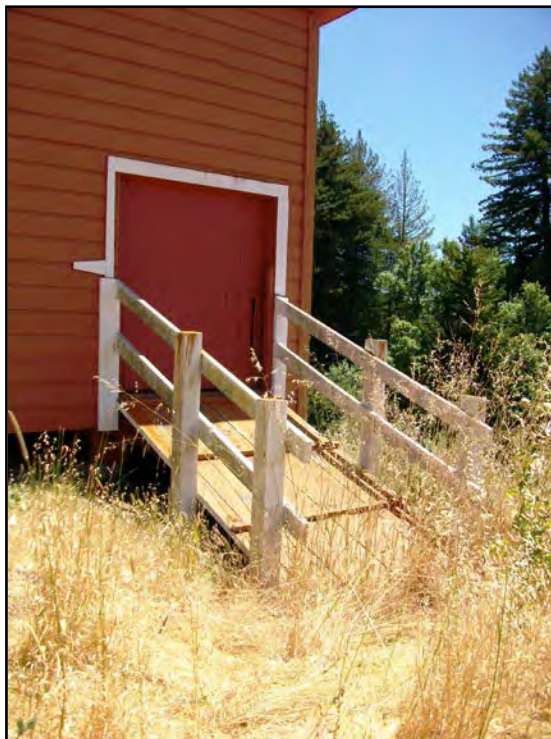
Red Barn, La Honda Creek Open Space Preserve, livestock access ramp, right side of north façade, view south. 6/21/16.
