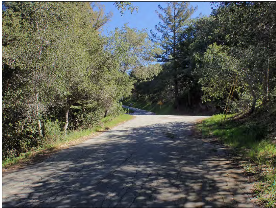
Entrance off La Honda Road/SR 84. Intersection of Old La Honda Road opposite. View northeast. LSA photograph, 3/10/22.
