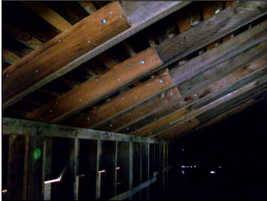
Red Barn, La Honda Creek Open Space Preserve, interior. Detail view of roof rafter reinforcement, west façade view north. 6/21/16.
