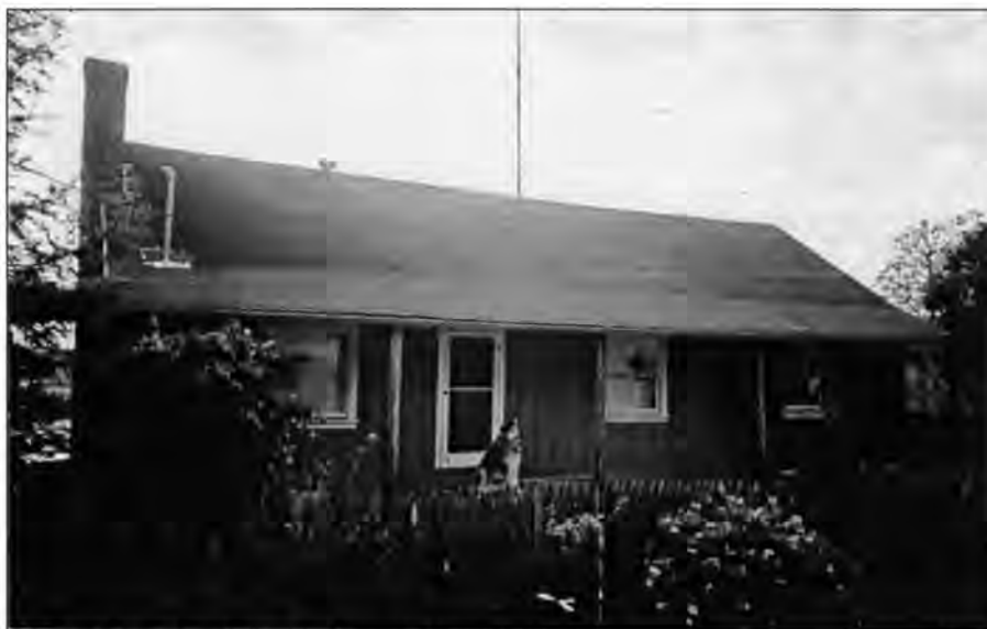
View 17 : East Elevation of Ranch House (by author)
