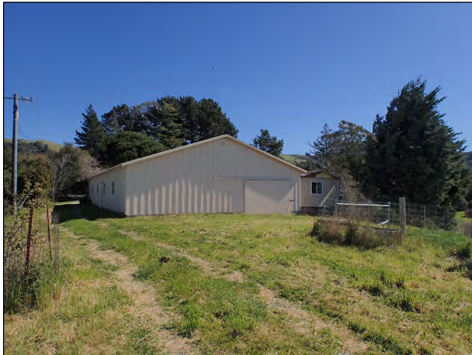
District Residence. Detached shop or storage building. West façade. View east. LSA photograph, 3/10/22.
