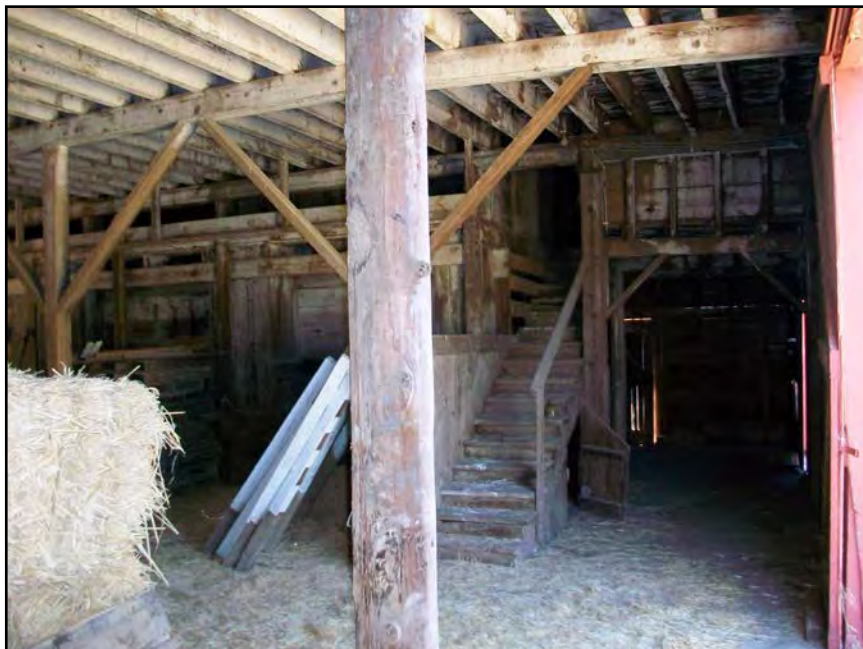
Red Barn, La Honda Creek Open Space Preserve, interior. View southwest from northeast corner. 6/21/16.
