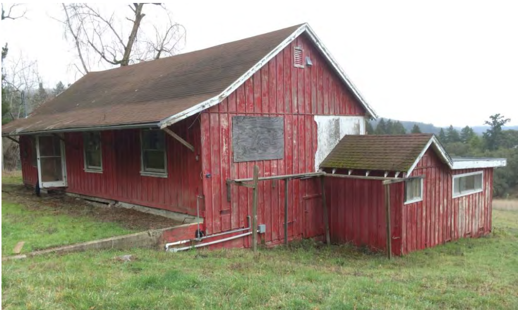
Figure 2 McDonald Ranch House – North and East Elevations
