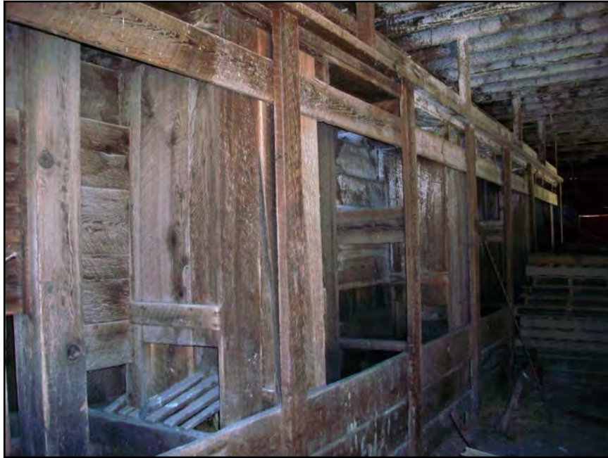
Red Barn, La Honda Creek Open Space Preserve, interior. View of feed chutes and cribs. View northwest from central two-story portion of Red Barn. 6/21/16.
