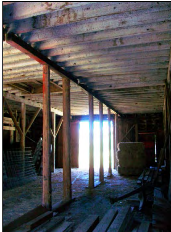
Red Barn, La Honda Creek Open Space Preserve, interior. View northwest from southeast corner. 6/21/16.
