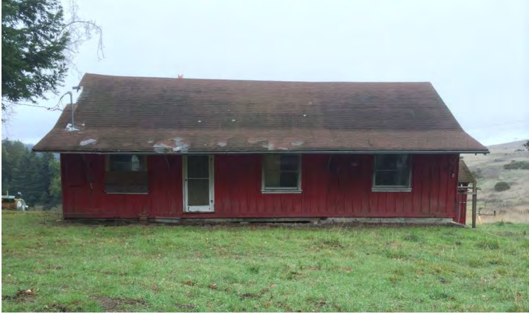
Figure 1 McDonald Ranch House – East Elevation
