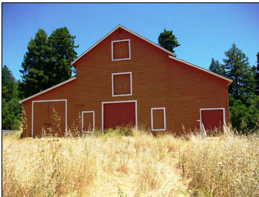
Red Barn, La Honda Creek Open Space Preserve, north façade, view south. 6/21/16.
