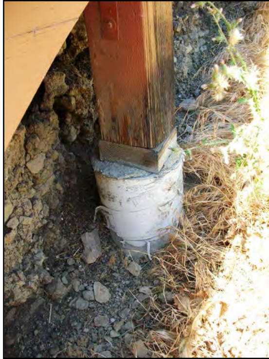
Red Barn, La Honda Creek Open Space Preserve. Detail view of caisson-drilled concrete foundation reinforcement. South façade. 6/21/16.
