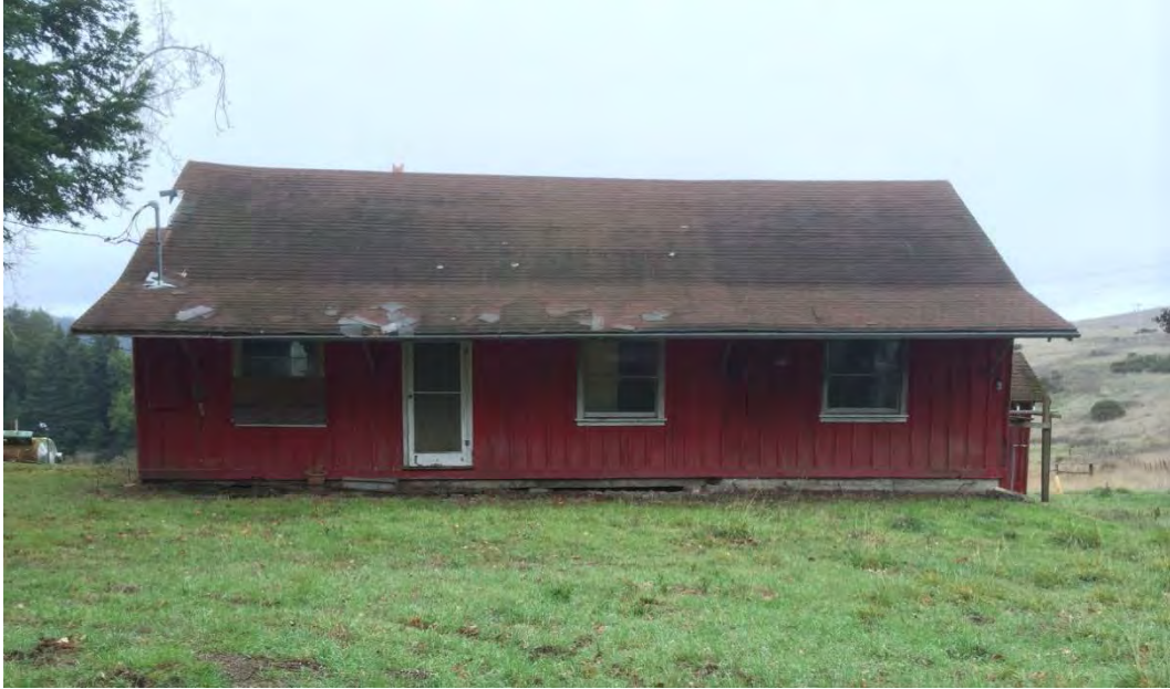
Figure 1 McDonald Ranch House – East Elevation
