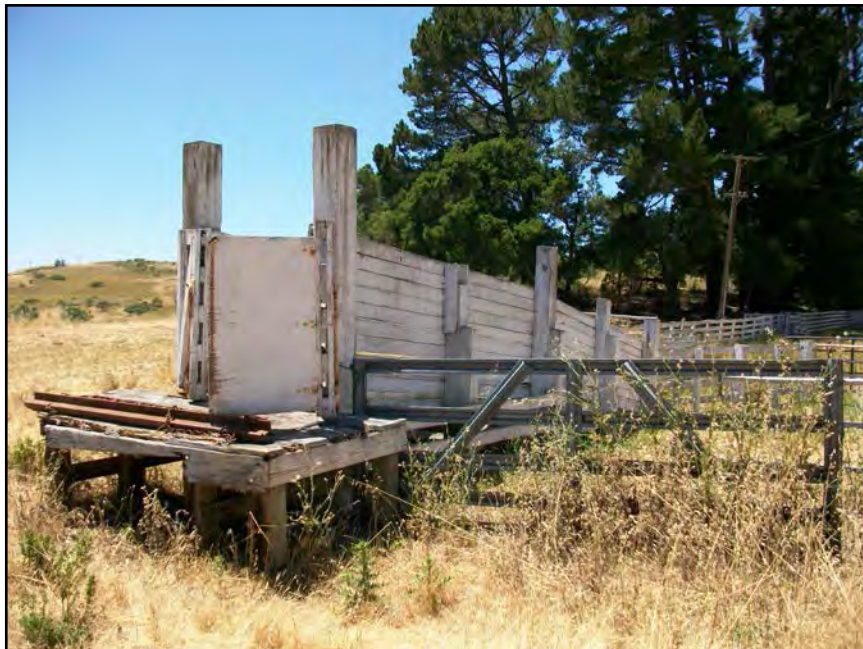
Corral, La Honda Creek Open Space Preserve, squeeze chute and ramp, view north. 6/21/16.
