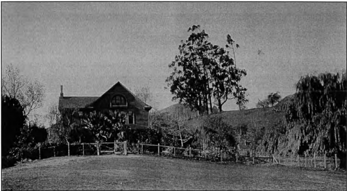
View 6: Burt Weeks' Residence - south elevation (facing barn)
