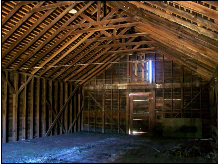
Red Barn, La Honda Creek Open Space Preserve, interior. Hay loft, view southeast from northwest corner. 6/21/16.
