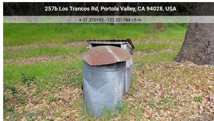
Photograph 10. View of an inactive groundwater production well at the eastern portion of the subject property.
