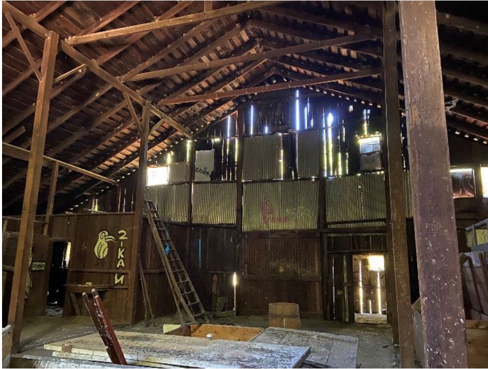
Photo 17. Main room in the lower barn. Note roof sheathing and corrugated metal wall panels.
