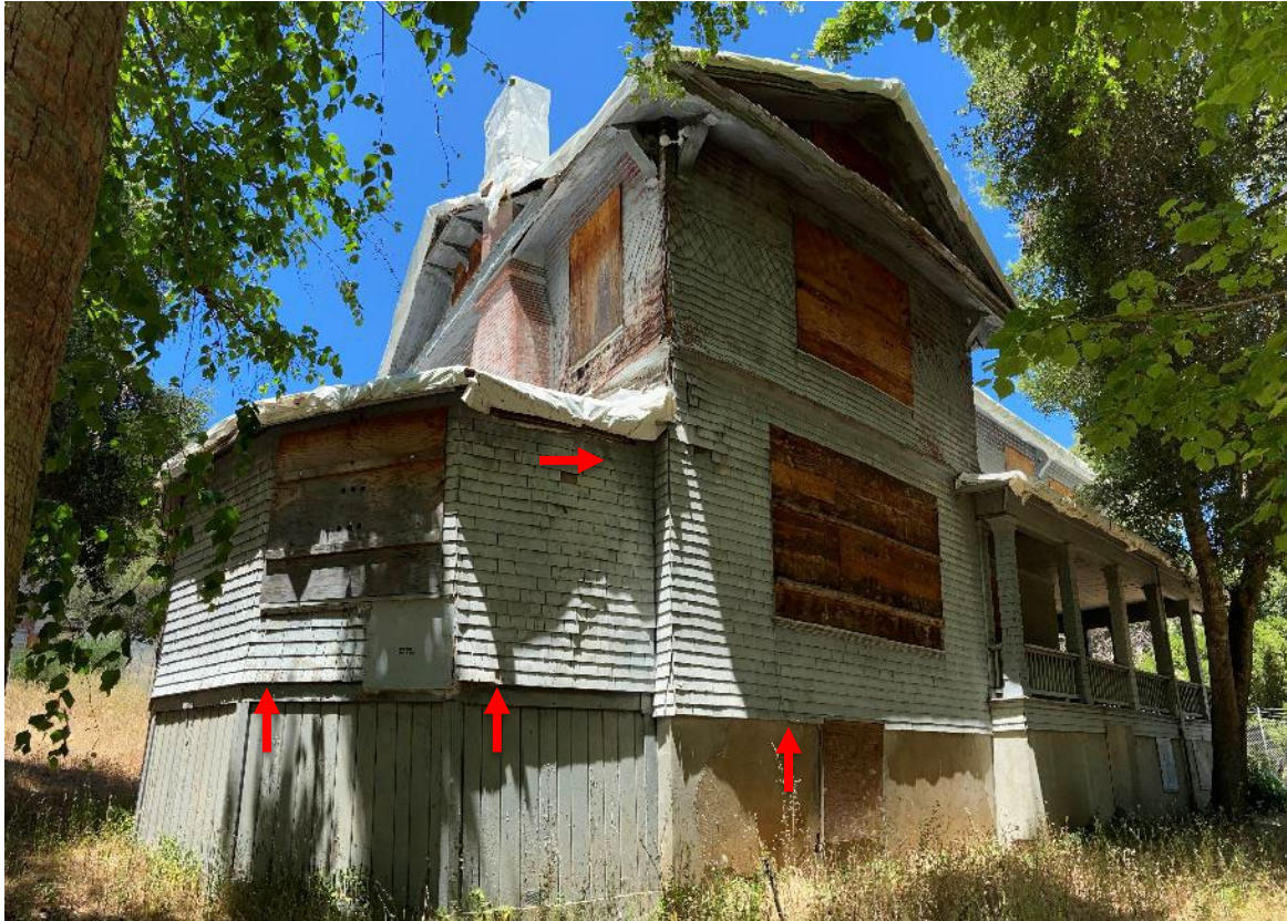
Photo 6. Crevices on the south/southwest exterior of the Hawthorn House.
