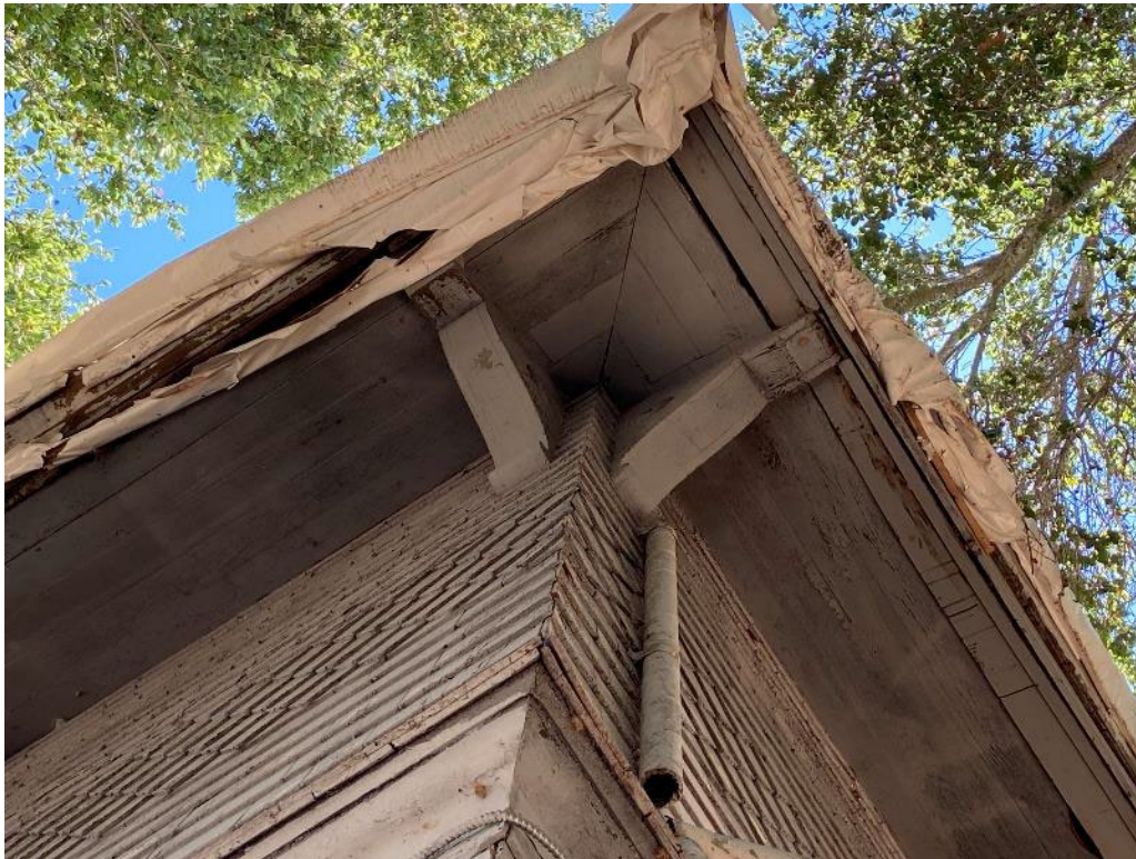
Photo 8. Crevice on the northwest corner of the Hawthorn House.
