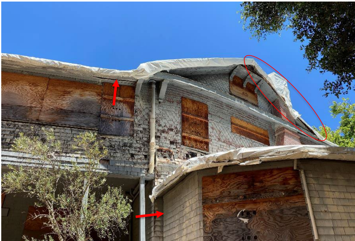
Photo 5. Crevices on the south side of the Hawthorn House.
